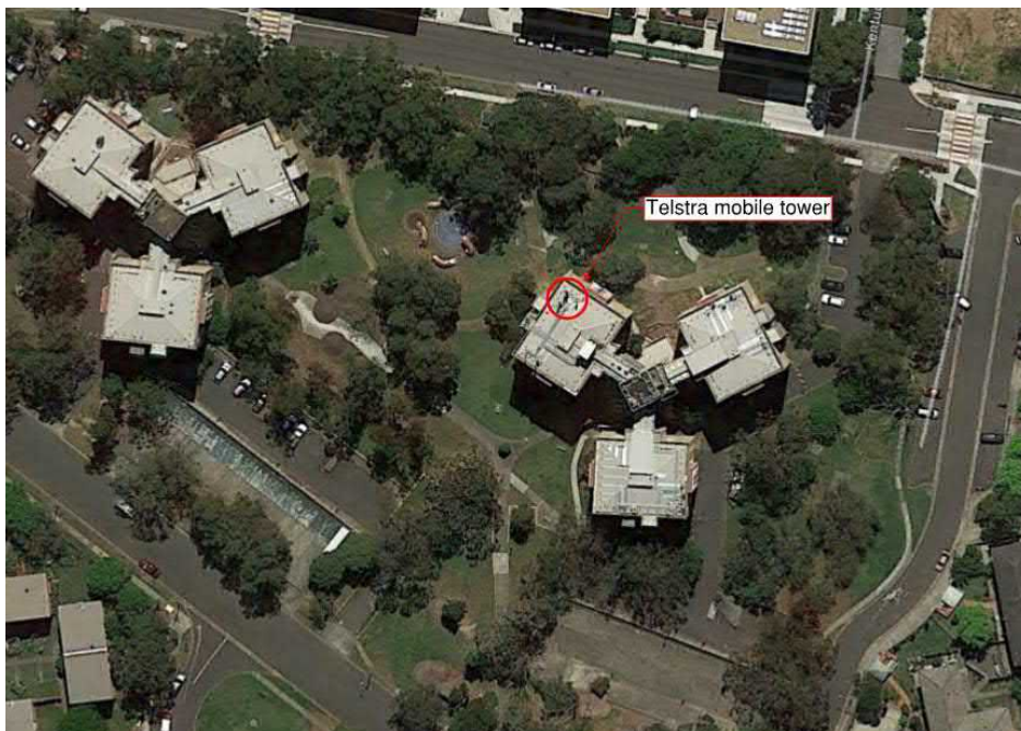
Figure 9: Telstra Mobile Tower Location
