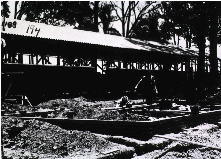
Figure 9: Brick footings and utility trenches under construction at Herne Bay Hospital, 1943. 24
