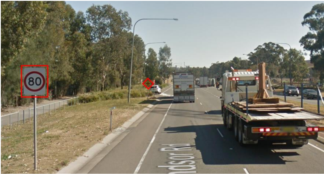
Figure 3.2: Existing road signs on approach to the proposed northbound facing advertising sign
