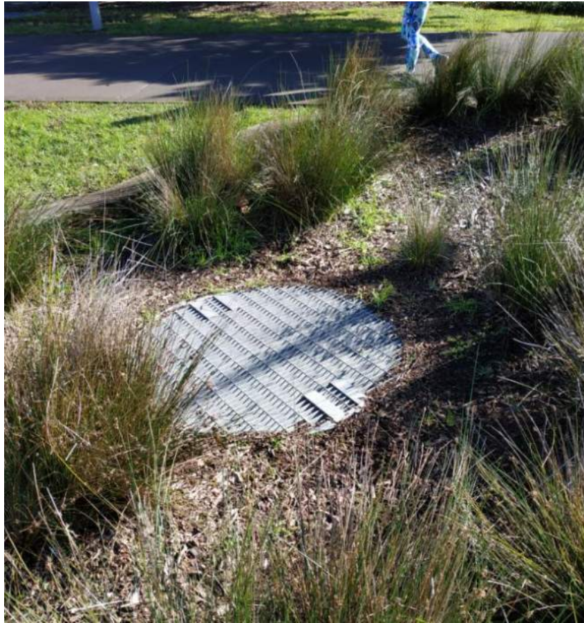
Photo 6-1: Prince Alfred Park Basin Outlet
