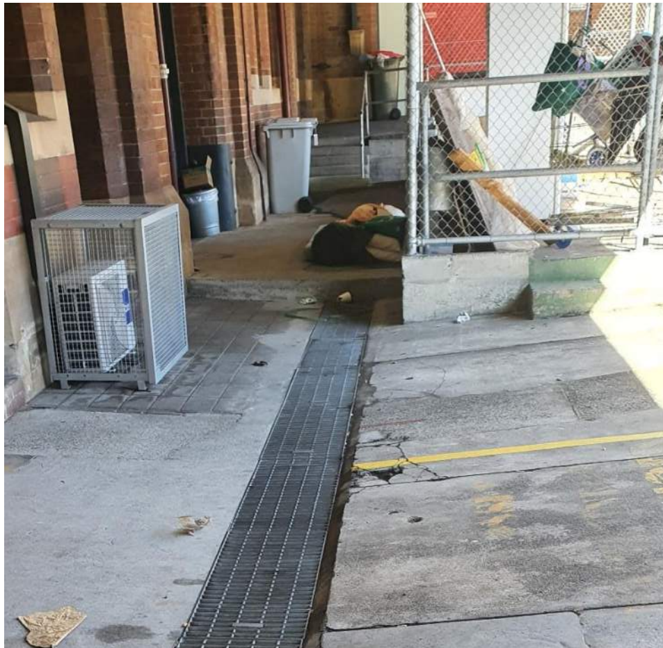
Photo 6-4: Ambulance Ave Grated Drain
