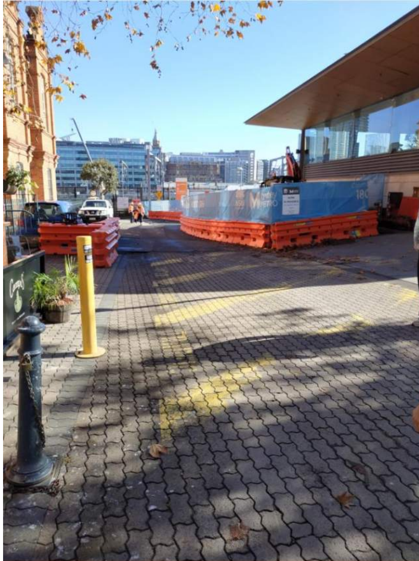
Photo 6-2: Sydney Trains Access Road from Devonshire St/Chalmers St Intersection
