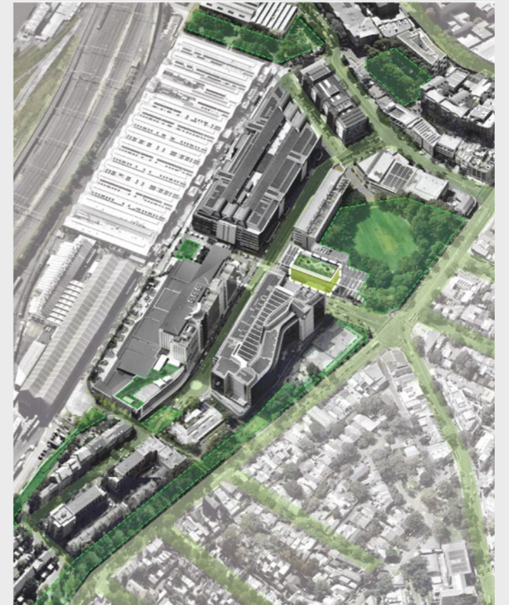
The rooftop contributes to a connected network of green infrastructure, even in a heavily urbanised environment.
