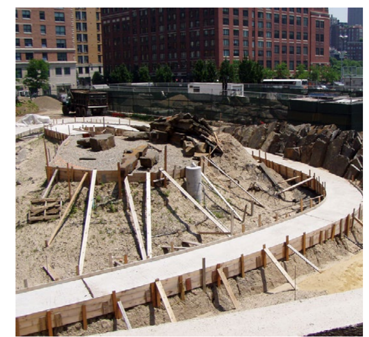
Construction of the mounded landform. Image: MVVA
