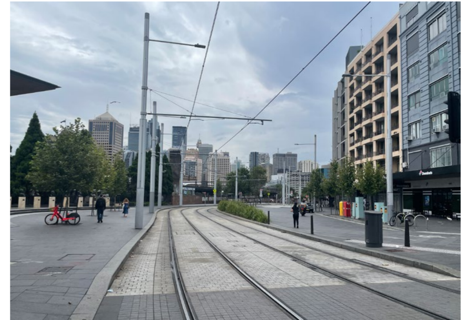
Chalmers Street has been transformed by the recent light rail development and will improve further with greater activation and larger tree canopies. The current pedestrian experience offers clear sightlines yet little protection from the elements.
