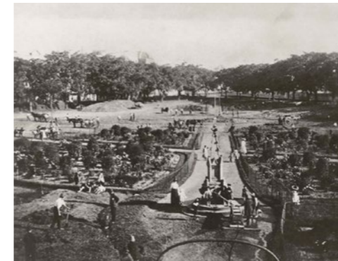
1879 photograph of construction in Belmore Park. Source: NSW State Archives
