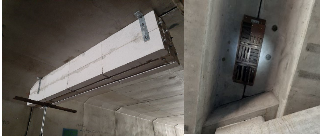
Concrete crevices similar to deep bridge expansion joint designed for replacing roosting spaces under concrete bridges
