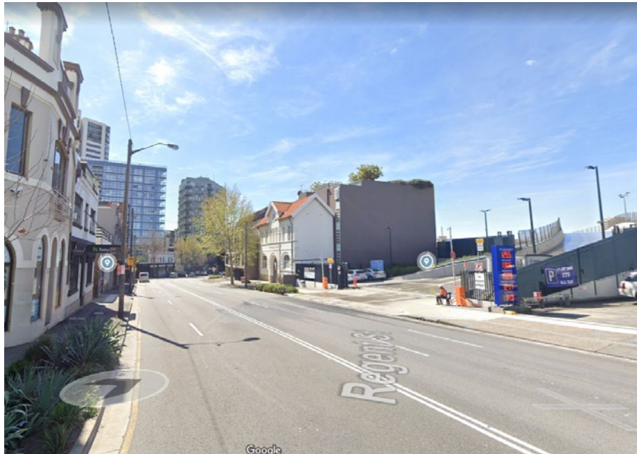
On Regent Street , Plane trees and Mortuary Station gardens provide a breath of green, yet pedestrians on the eastern footpath navigate a bus depot, railyards access and a petrol station. The western side skirts apartments, terraces and warehouses with links through to Chippendale.
