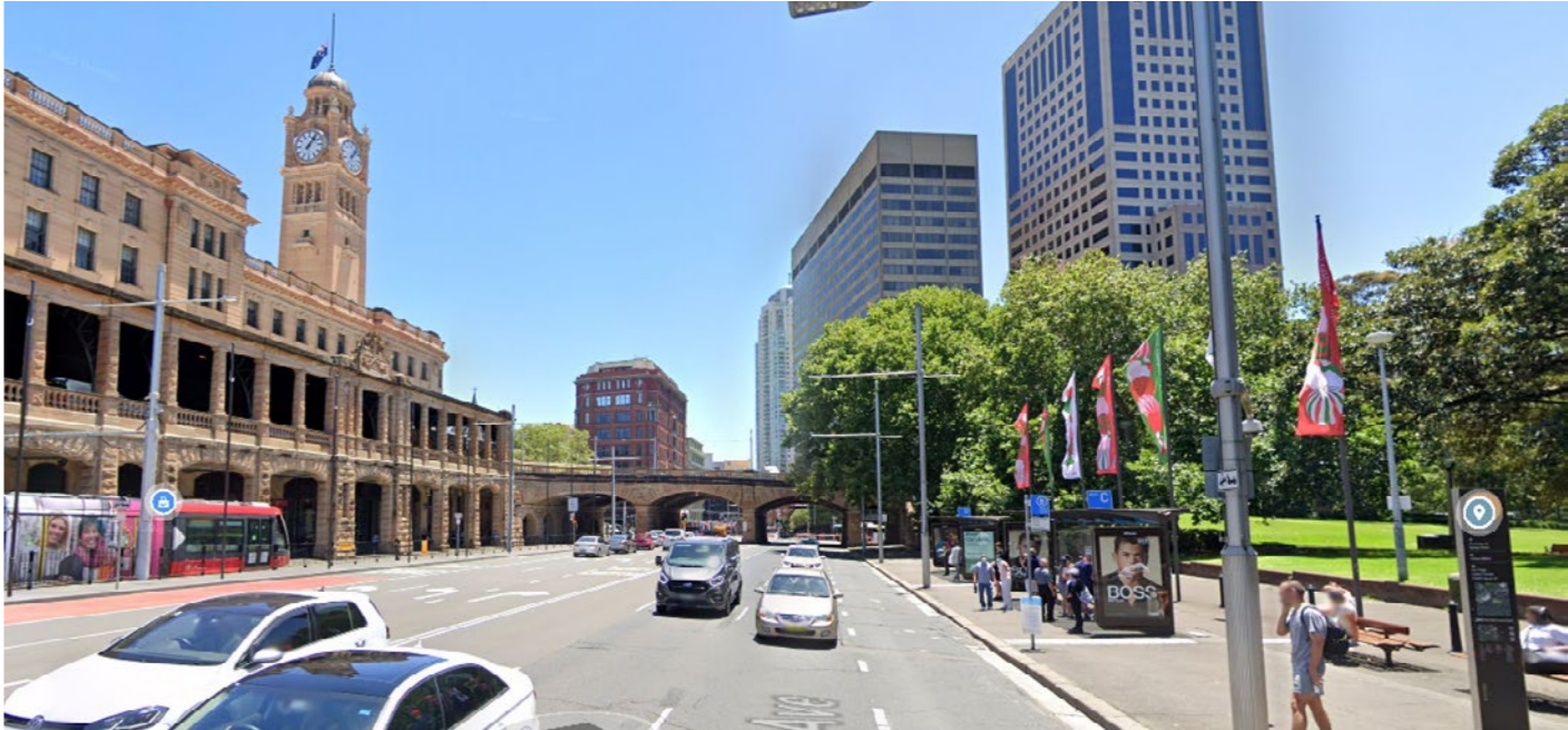
Framed by Belmore Park, the Sydney Terminal Building and two overpasses, Eddy Avenue has the proportions of a grand civic boulevard. Currently eight lanes of vehicles, bus bays and light rail, pedestrians crowd along the edges and funnel through tunnels with limited opportunities to cross. The mature Fig trees of Belmore Park and the terminal colonnade provide street presence and offer pedestrians protection from the elements.
