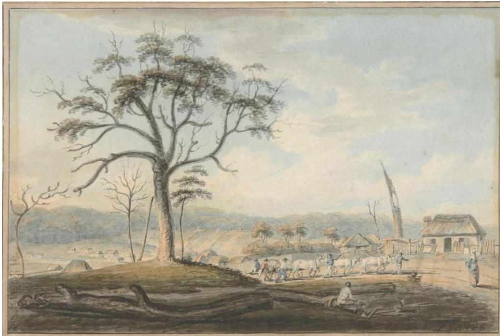
Figure 17: Brickfield Hill and village on the High Road to Parramatta, 1797. Source: National Library of Australia 41
