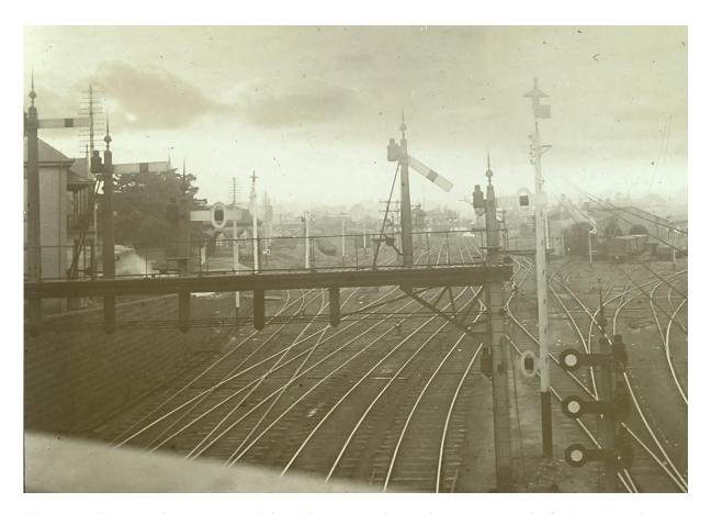
Figure 22. The growing number of signalling and safeworking structures in Sydney Yard is illustrated in this 1880s photograph by John Henry Harvey, with Mortuary Station on the left (Source: State Library of Victoria, H91.300/43)
