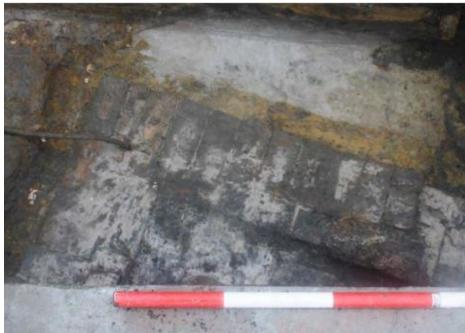
Figure 393. View of brick footing in section below modern concrete. Source: Mountains Heritage 2021 Plate 2:2.
