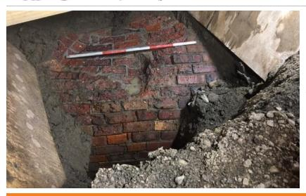
Figure 9. Brick drain uncovered in Sydney Yard on 10 April 2021 during works for MTMS 2. Source: Artefact Heritage
