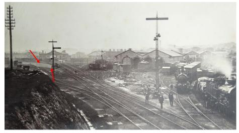
Figure 297. 1877 photograph, showing the retaining wall of the Darling Harbour dive. Source: SLNSW. Photographic views: The Railways of New South Wales / compiled from reports by Rae [John], commissioner, and Whitton [John], Engineer-in-Chief for Railways. PXD 1175.
