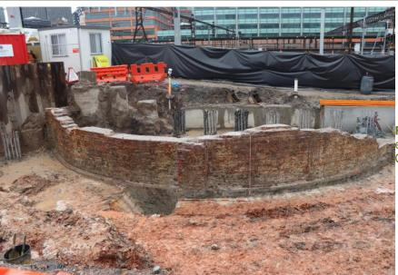
Figure 667. The Gas Holder following excavation in February 2019 during the CMS works. Source: Artefact 2020
