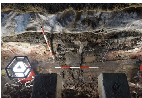
Figure 402. Small brick footing exposed in the east section of the drainage trench. Source: Mountains Heritage 2021
