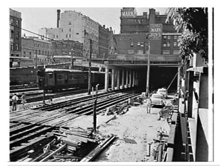
Figure 118 c.1962. Goulburn Street Parking Sta.tion under construction. Note the large structural piers between the railway lines.
