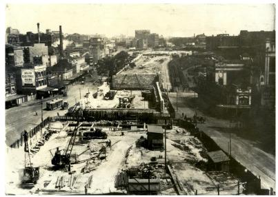
Figure 99. c.1925. Looking south from Goulburn Street. Electric railway lines between Central Station and Town Hall under construction. Note the extensive excavation work required to construct the lines, which are located beneath street level.
