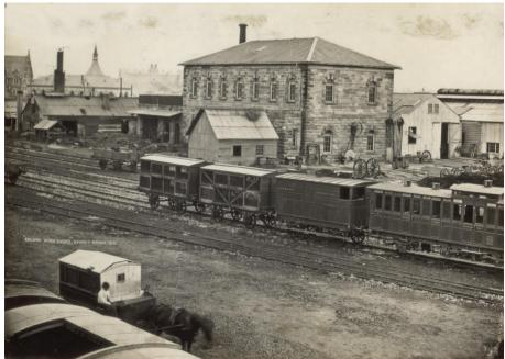
Figure 21. 'Redfern Railway Workshops, Sydney, March 1871' Note: Two-storeyed workshop building with first Blacksmith's at rear (before demolition) and showing c.1860s expansion of workshops to the west (in less robust materials). Source: Redfern Railway Workshops, Redfern Nsw 1871." State Records NRS 17420 State Rail Authority **Archives Photographic Reference Print Collection,** 1871.
