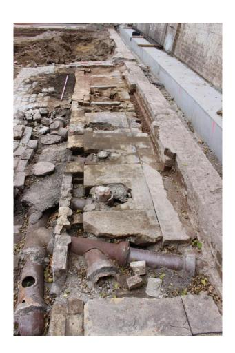
Figure 306. Northeast view of the lower portion of the South Toilets cubicles following the removal of the top concrete and bricks.
