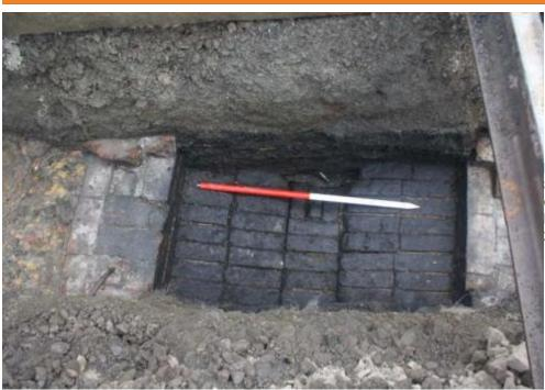
Figure 389. View of SY0197/H22 inspection pit with central drain. Source: Mountains Heritage 2021 Plate 2:6.
