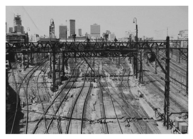
Figure 26. By 1980 the overhead wiring and signalling systems in Sydney Yard had been fully adapted for the end of steam train services (Source: City of Sydney Archives, A-000197)
