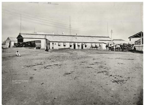
Figure 13. First Sydney Railway Station, 1871. This is the first Sydney Railway Station, showing the remains of the old tramway tracks where man is sitting. The Goods Shed is on the far left and the platform on the right side became the George St Platform. Source: State Records, Digital ID 17420\_a014\_a0140000245
