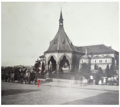
Figure 289. 1877 photograph of Mortuary Station, showing the stone and iron railing fencing and the timber railing fencing in the background. Source:-SLNSW. 16. Mortuary, Sydney, looking east.
