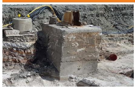
Figure 251. Typical stanchion base and hold down structure, Test Trench 1 CSM. Source: Artefact, 2018.
