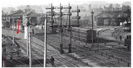
Figure 300. Photograph taken prior to 1904 of the 1884 Sydney Station Signal Box, showing the Darling Harbour branch dive retaining wall at the base of the signal box. Source: ARHS NSW in Taaffe 2019, p. 173.
