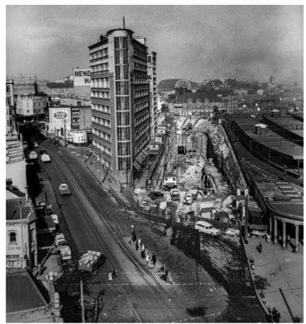
Figure 347. Photograph showing excavation of the ESR, extending across the total width of Chalmers Street. Source: City of Sydney Archives, SRC136.
