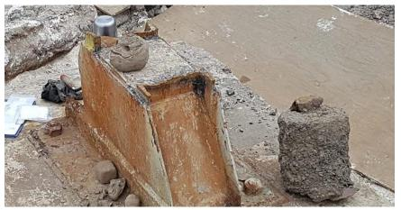
Figure 252. Detail of stanchion base pedestal and hold down structure for the mast. In this case the mast has been cut off and the whole structure was buried "in situ" only to be excavated as part of the Test Trench 1 excavations for Central Station Metro. Source: Artefact, 2018.
