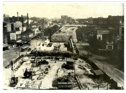
Figure 115. c.1925. Looking south from Goulburn Street. Electric railway lines between Central Station and Town Hall under construction. Note the extensive excavation work required to construct the lines, which are located beneath street level.
