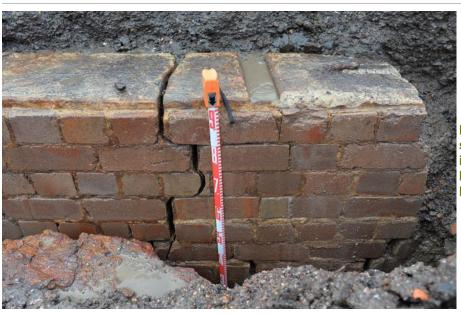
Figure 347. A photograph of a section of the wall of the ash pit identified during excavation for MTMS 2 (H1). Source: Mountains Heritage, 2020
