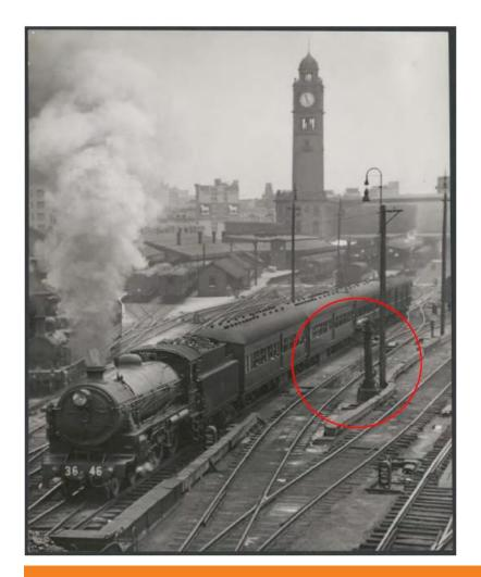
Figure 249. Photograph of a train leaving Central c.1940s. Example of a water column next to an ash pit is circled red. Source: Mountains Heritage 2021 Plate 2:10; Flickr – Central Station collection
