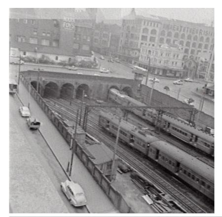
Figure 116. c.1956. Looking north towards the six underground railway tunnel entrances located beneath Goulburn Street. Signal box in the right corner. Note the level of ground disturbance due to the construction of the railway lines and their location beneath street level. This area is now concealed by the Goulburn Street Parking Station.
