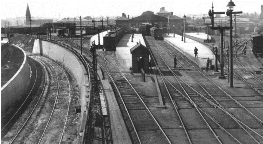
Figure 18: Northern view towards the Darling Harbour rail cutting to the left of frame. 95
