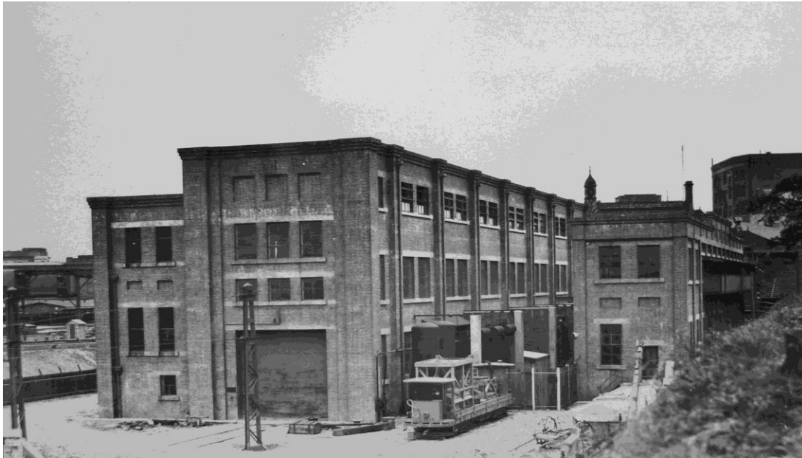
Figure 28: The Prince Alfred Substation c.1928, showing the main substation on the left, switching house to the right and outdoor transformers in the centre. 144
