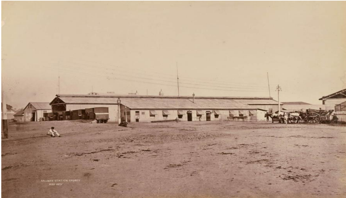
Figure 13: View towards the first Sydney Station, 1871 showing the remains of the old tramway tracks . The Goods Shed is located to the left while the platform on the far right became the George Street platform.
