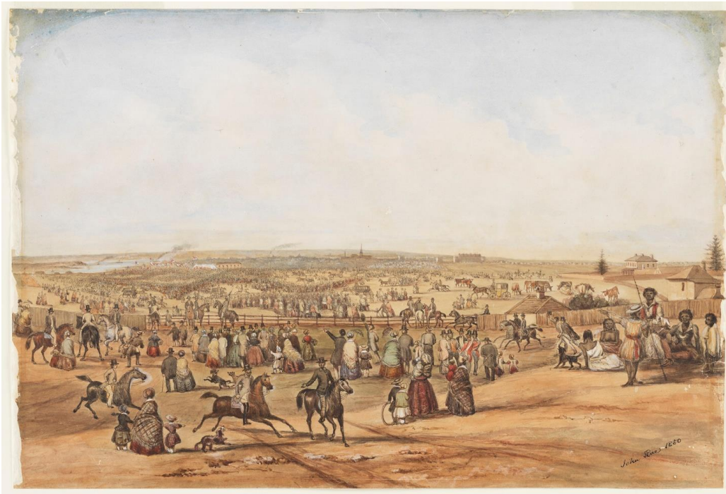
Figure 7: Turning the first turf of the first railway in the Australasian colonies at Redfern, Sydney, July 1850. John Rae. Source: State Library of NSW
