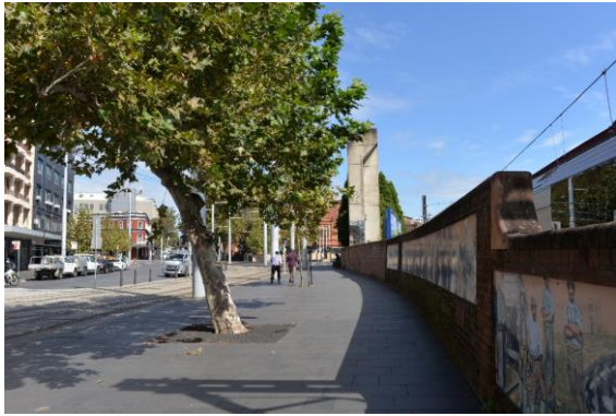
Figure 39: View towards Devonshire Tunnel entrance, with zero surface visibility
