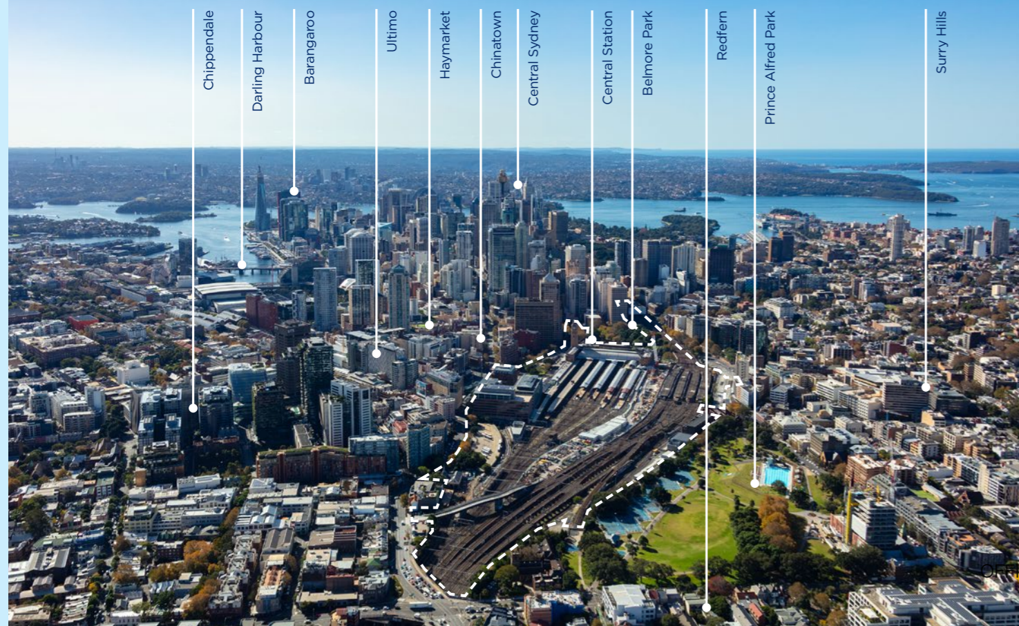
01. Aerial (source: airview online)
