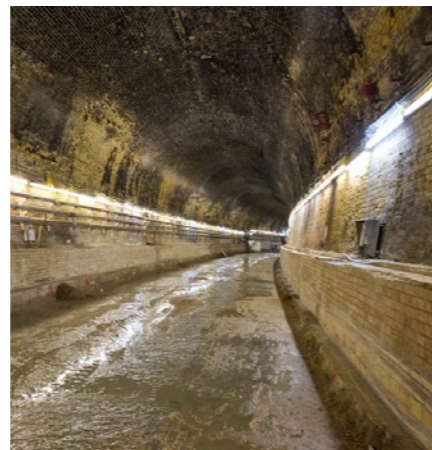
161. Photograph of lighting installation at the Connaught Tunnel, UK. Image: Crossrail
