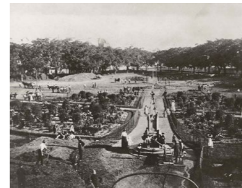
235. 1879 photograph of construction in Belmore Park. Source: NSW State Archives
