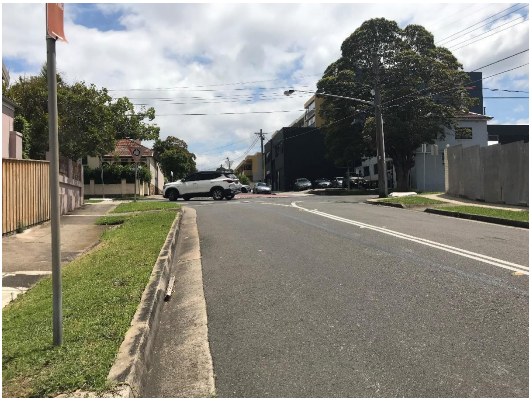
View looking southeast along Formosa Street towards its intersection with Day Street
