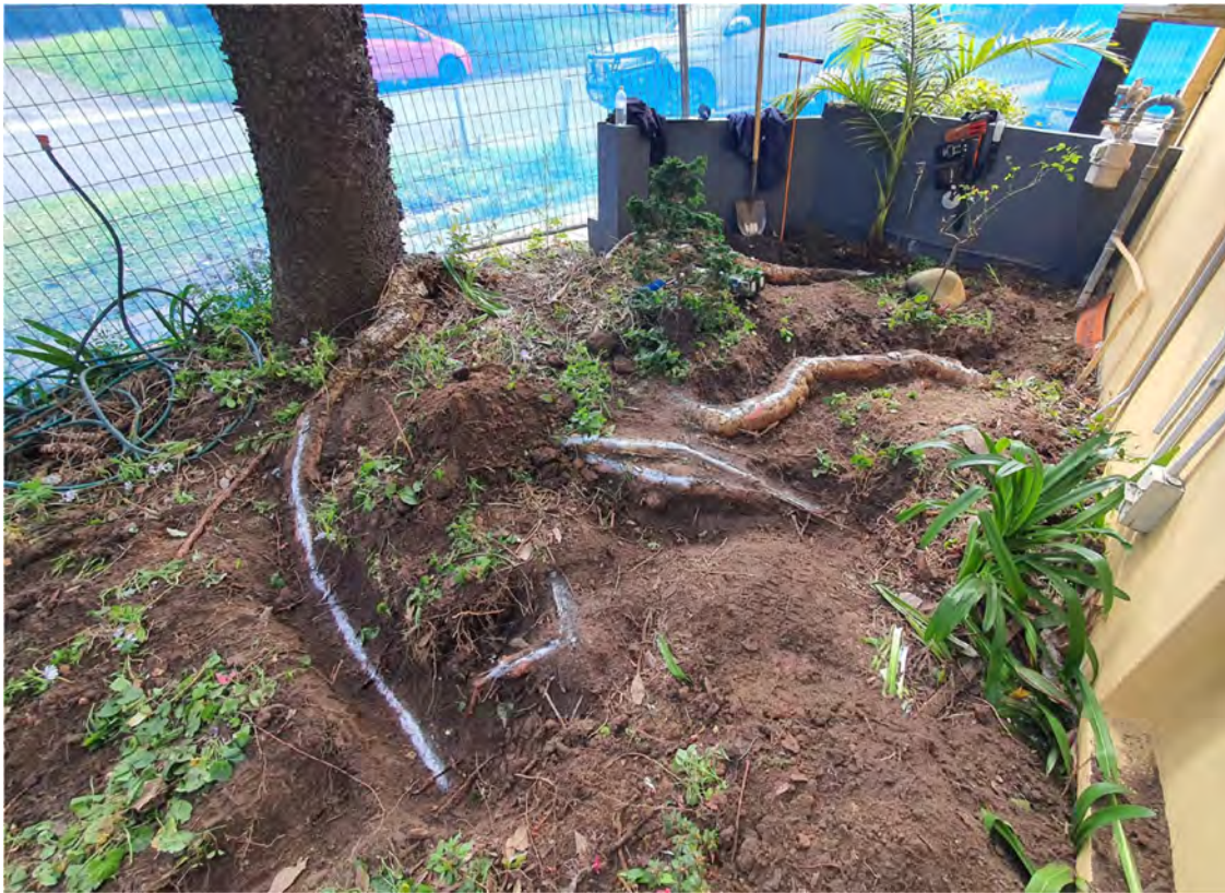
Image 3: Tree roots as discovered. Roots were marked with white line marking paint for contrast in photos.
