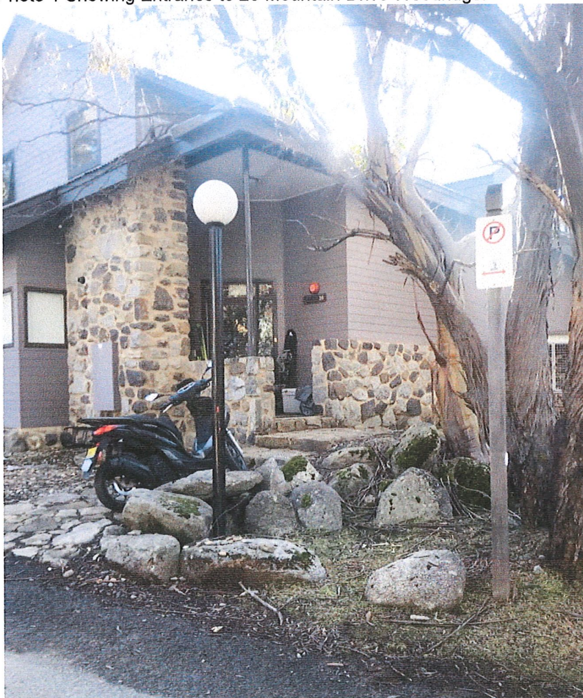
Photo 1 Showing Entrance to 20 Mountain Drive Woodridge.
