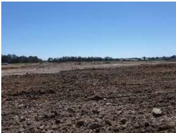
Figure 15: View of construction site from southern extent of study area
