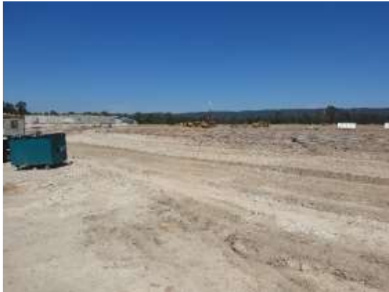
Figure 13: View of construction site from eastern extent of study area
