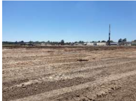
Figure 14: View of construction site from southern extent of study area
