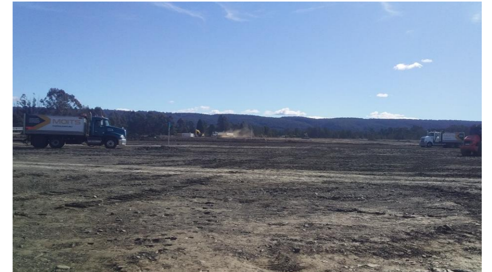
PIC 6. VIEW FROM SITE TOWARDS WESTERN BOUNDARY
