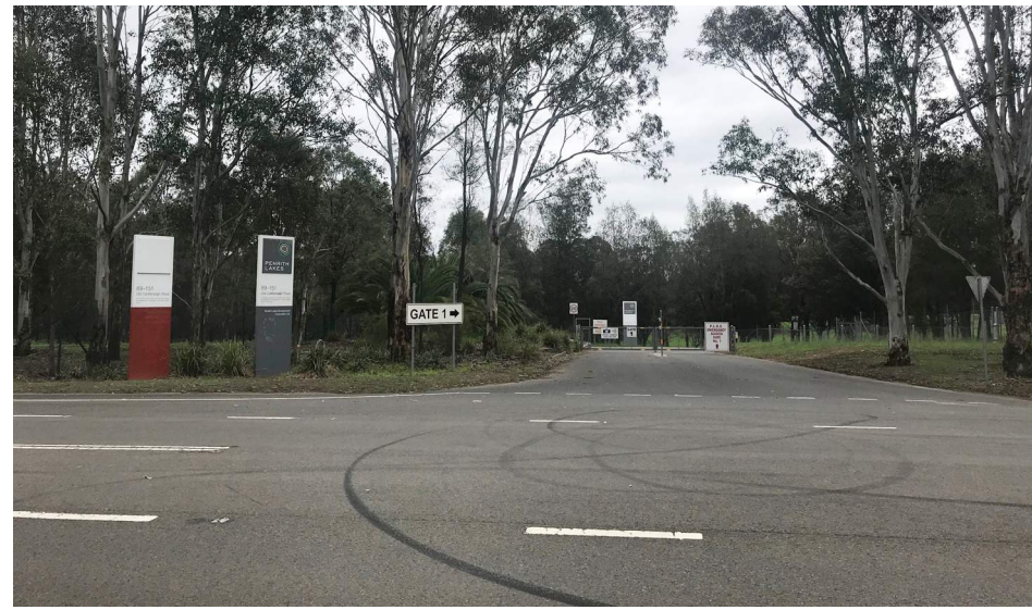
11 EXISTING ENTRY TO PLDC OFFICE COMPOUND
