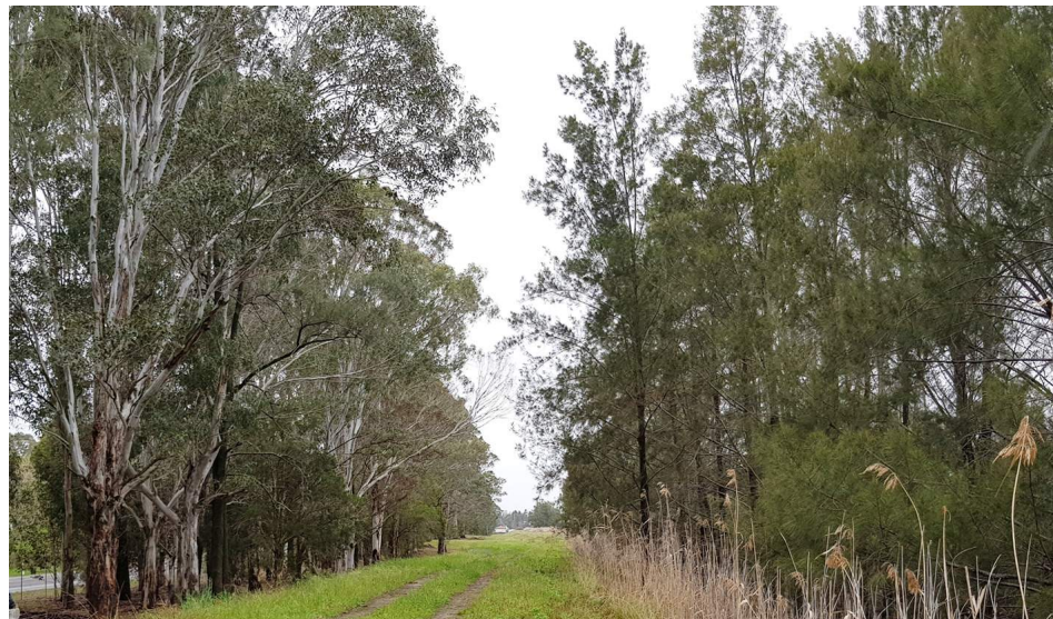
7 TOP OF EMBANKMENT PARALEL TO OLD CASTLEREAGH ROAD
