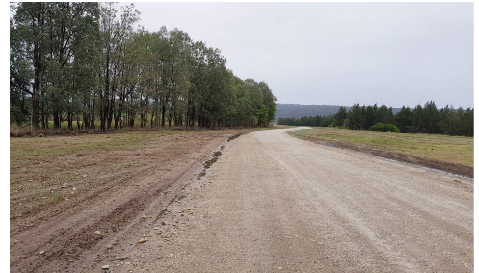
6 VIEW FROM SITE TOWARDS WEST AND DETENTION BASIN
