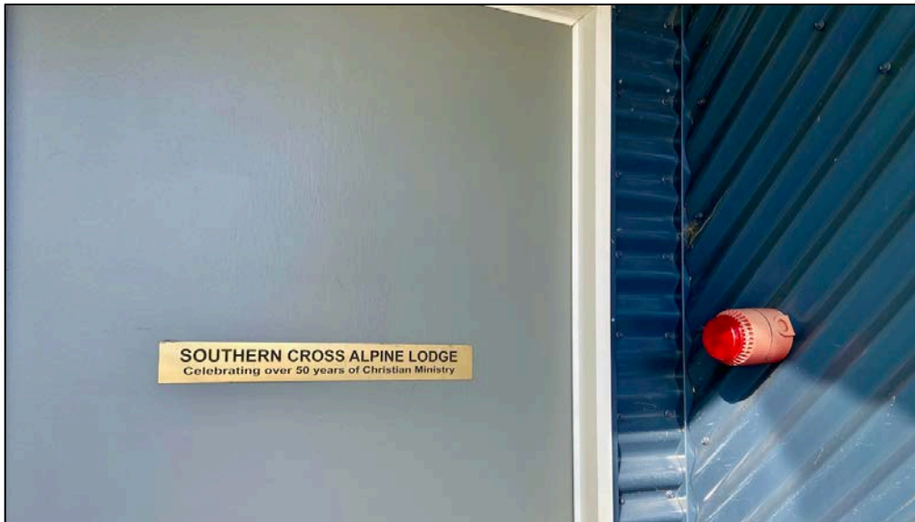
Figure 16 – Strobe associated with fire detection system (Dau, 2020)
