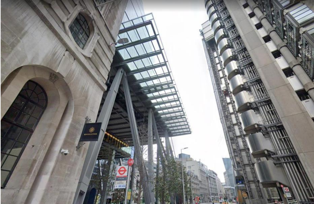
Figure 50: Example of localised wind mitigation measure (awning)
