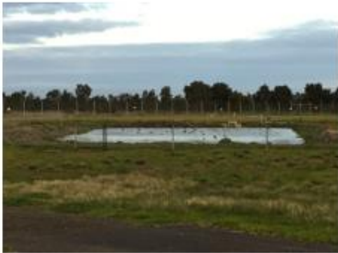
Figure 23. Retention or detention areas with inadequate fencing and gently sloped banks have the potential to attract terrestrial animals such as kangaroos.
