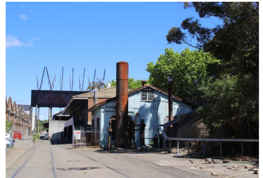
Plate. 6 Detail of eastern elevation of the Compressor House and view west down Carriageworks Way
