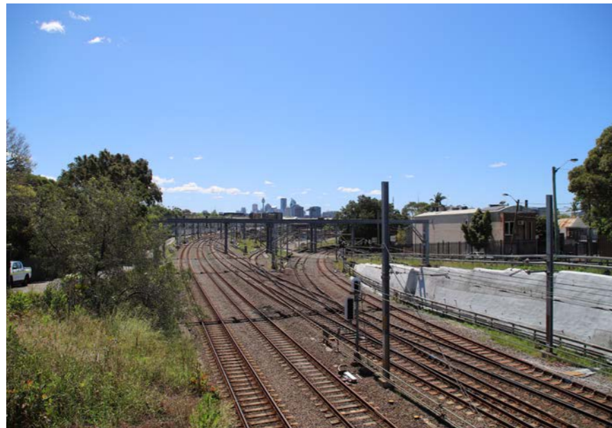
Plate. 23 View north-east from pedestrian bridge at Erskineville Station
