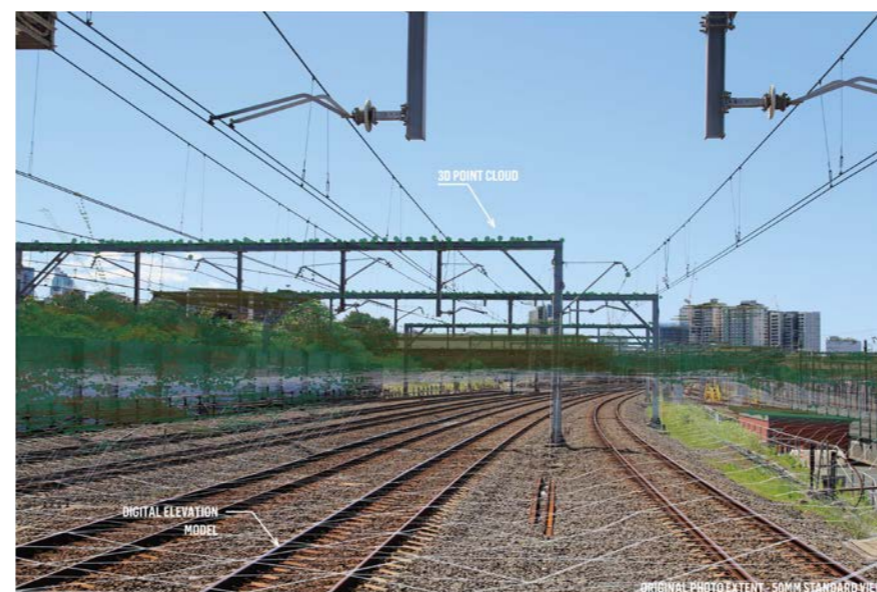
Figure 41 View 07 - Existing conditions with 3D point cloud for accurate alignment of model overlay on photograph
