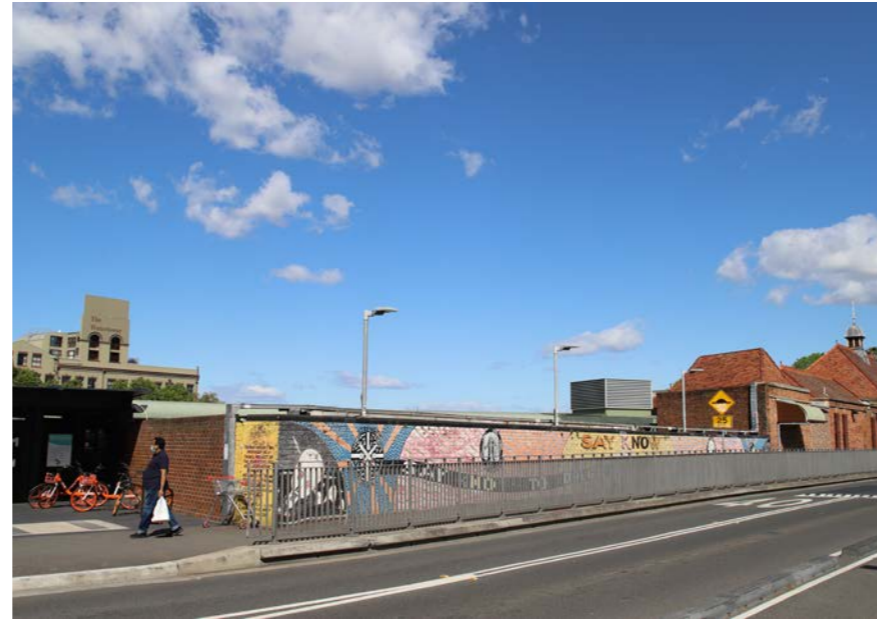
Plate. 11 View south-west from northern side of Lawson Street opposite the entry to the Redfern Station Southern Concourse
