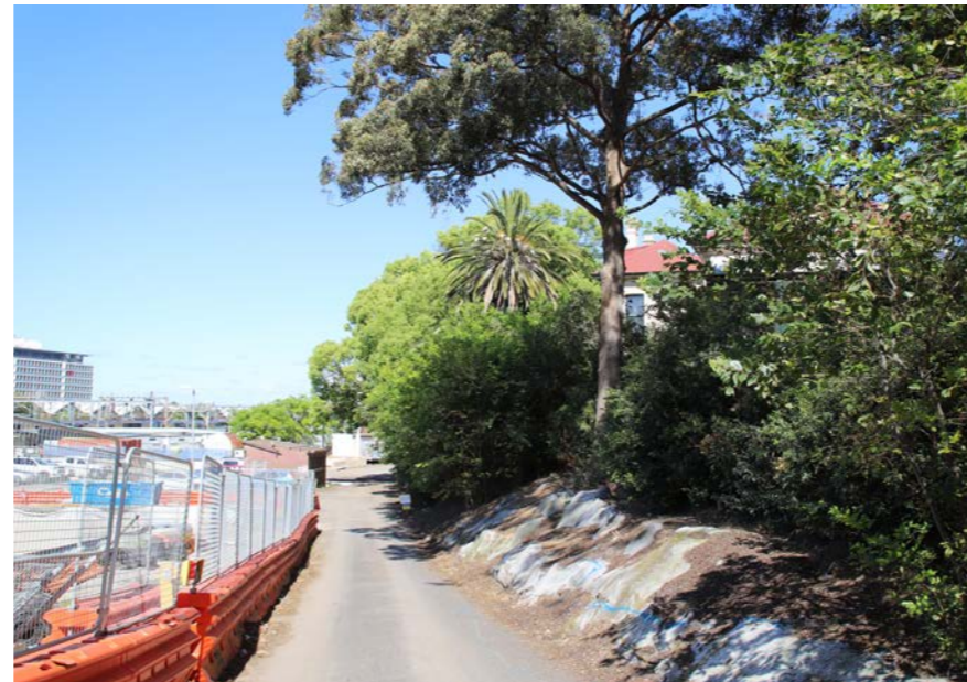
Plate. 14 View to north-eastern corner of site from western end of Little Eveleigh Street
