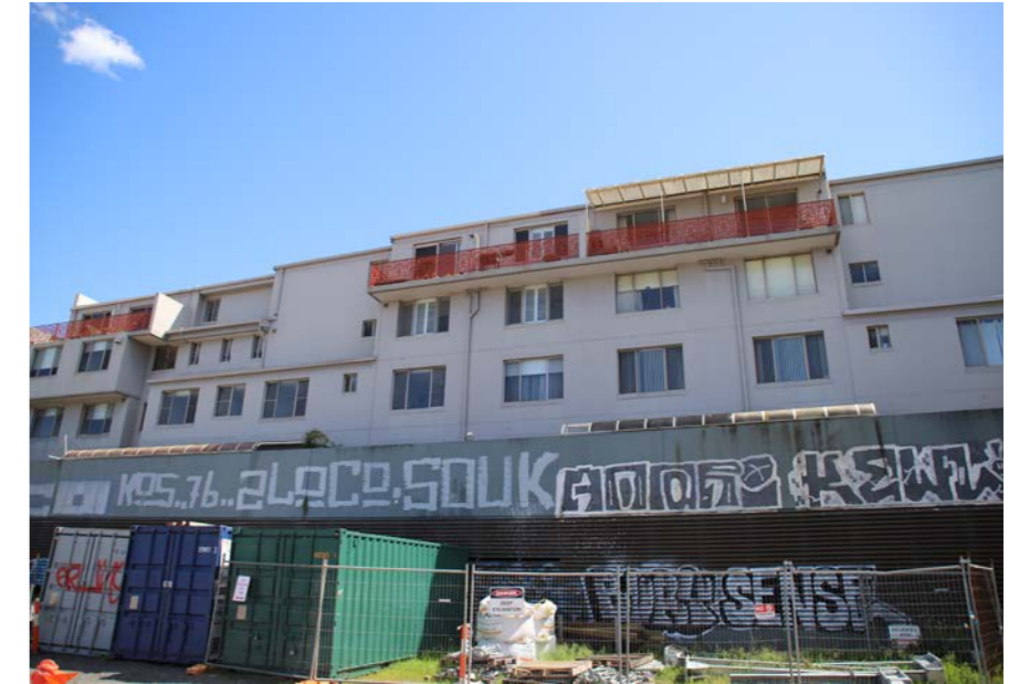
Plate. 18 Detail of southern elevation of Beveridge Mews (501 Wilson Street) on the southern side of Wilson Street
