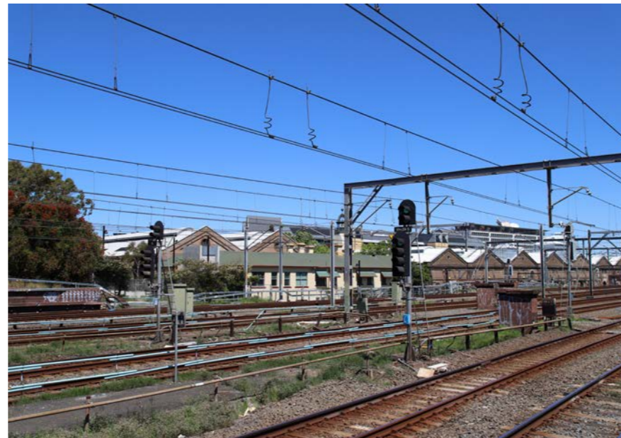
Plate. 29 View south-west from end of Platform 3 at Redfern Station
