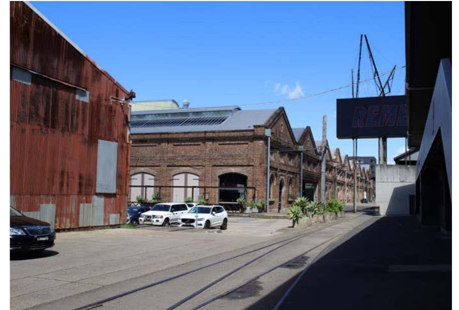
Plate. 3 View south-west towards the Carriage Workshop and northern elevation of the Paint Shop Extension
