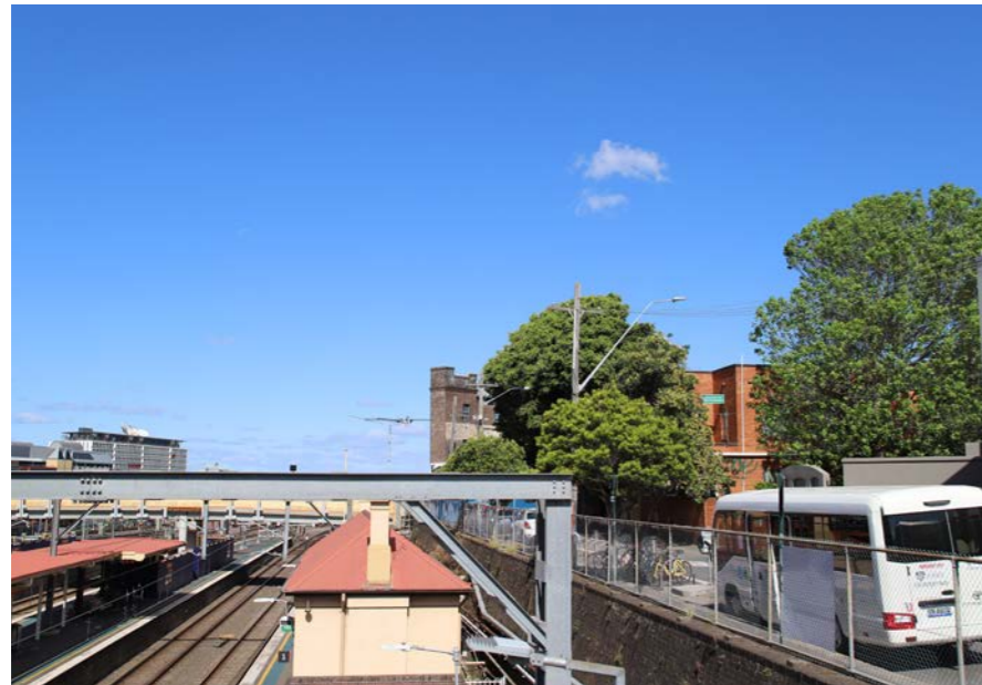
Plate. 13 View south-west from entry to western most platform at Redfern Station
