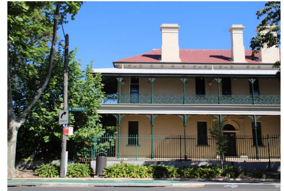
Plate. 30 Detail view of Chief Mechanical Engineer's Office from the north
