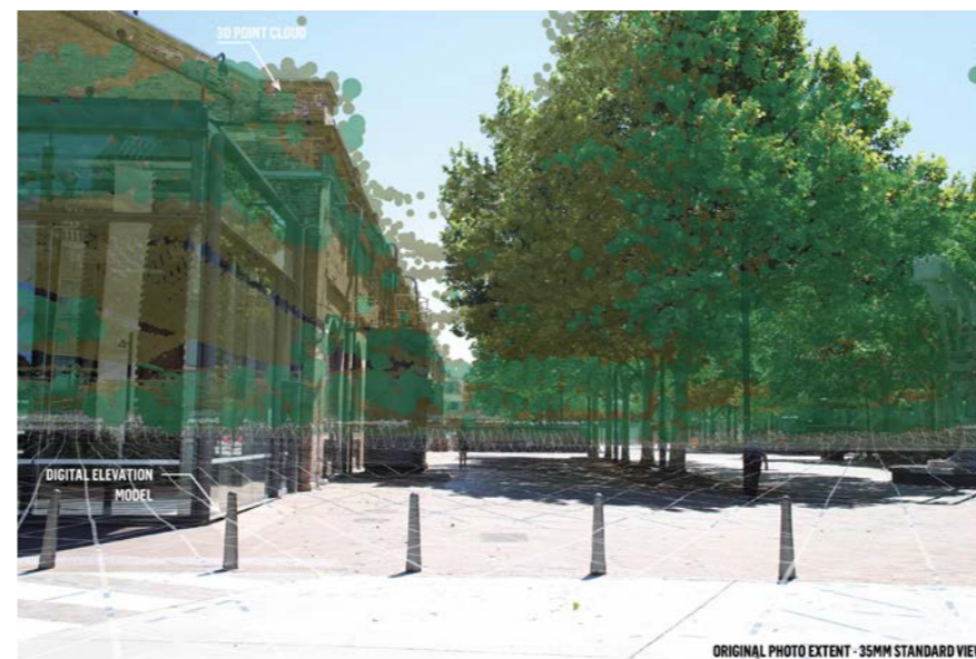
Figure 44 View 08 - Existing conditions with 3D point cloud for accurate alignment of model overlay on photograph
