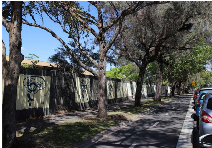
Plate. 19 Detail of steel fence on the northern boundary of the site
