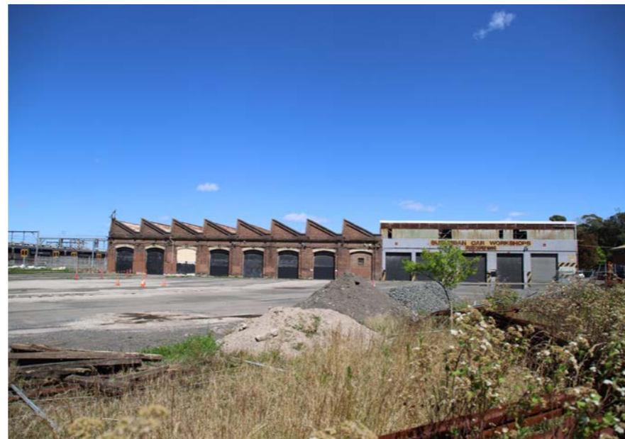
Plate. 5 View west to the eastern elevation of the Paint Shop and Paint Shop Extension
