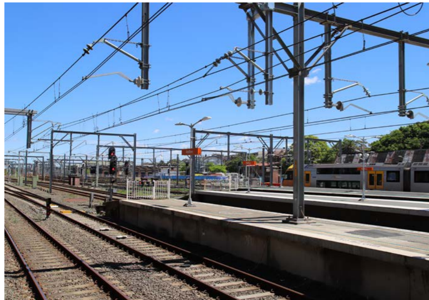
Plate. 28 View north-west to site from end of Platform 3 at Redfern Station
