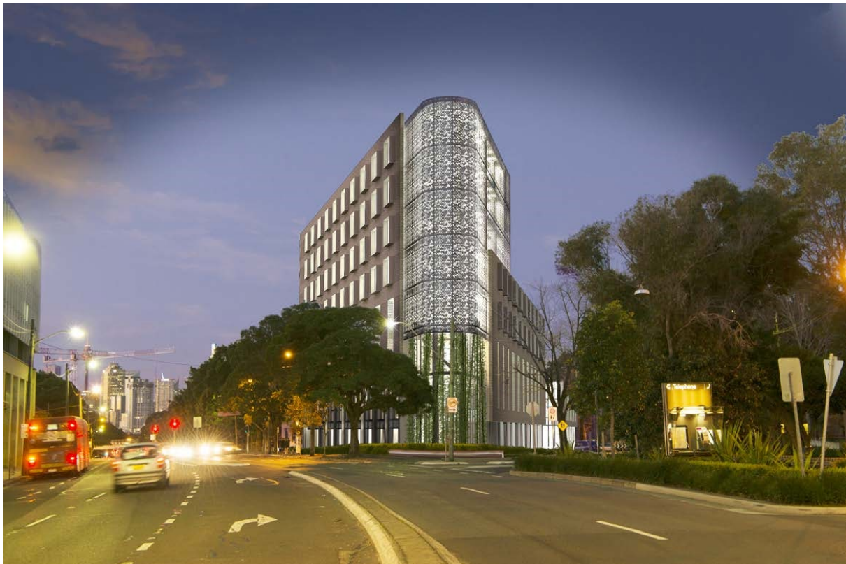
Figure 6 New Regiment Building at Camperdown-Darlington Campus
