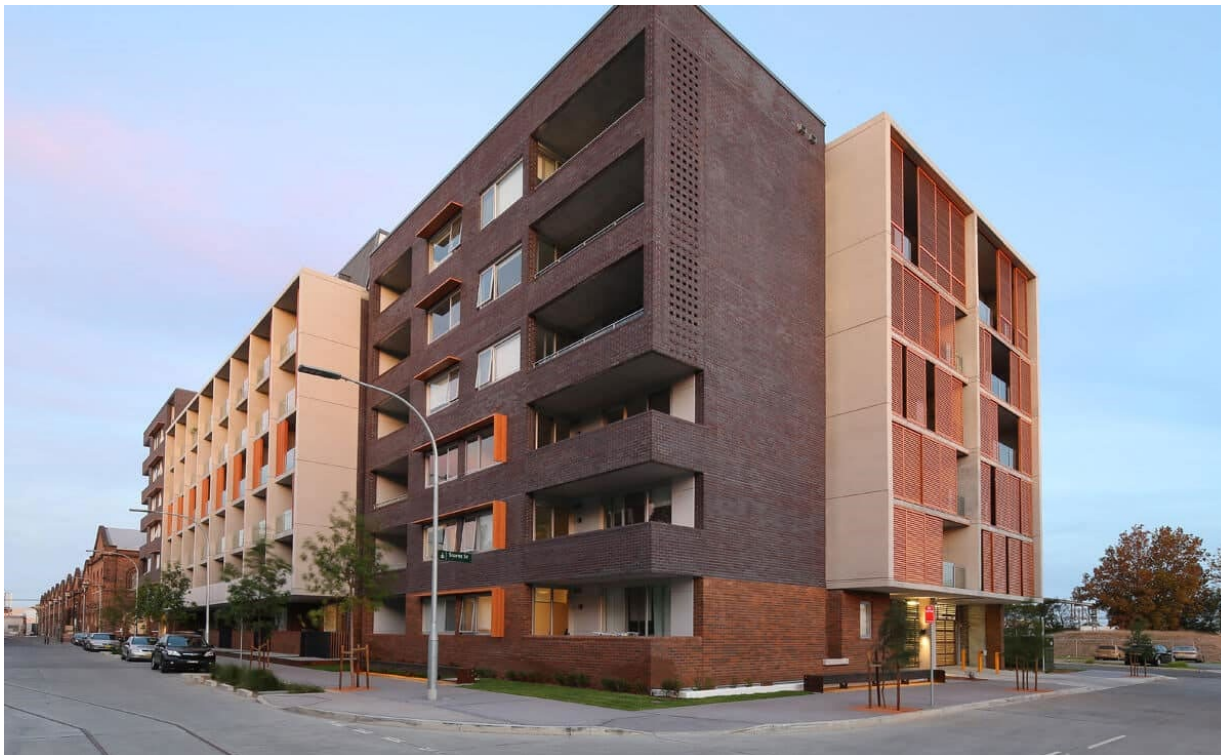
Figure 24 North Eveleigh affordable housing delivered by CityWest in the Clothing Store sub-precinct
