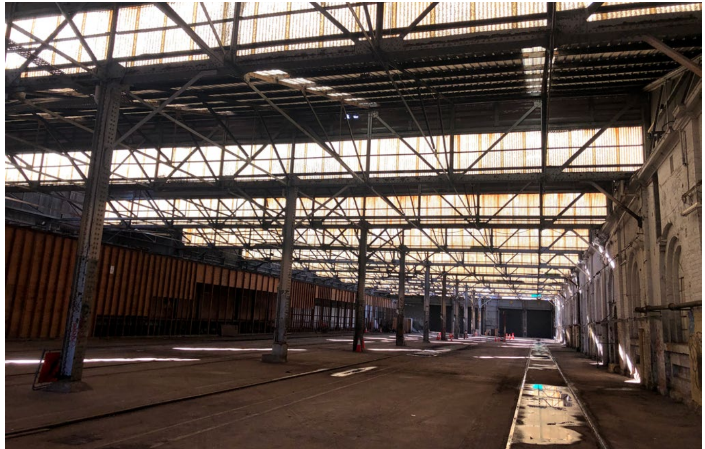
Existing Paint Shop structure
