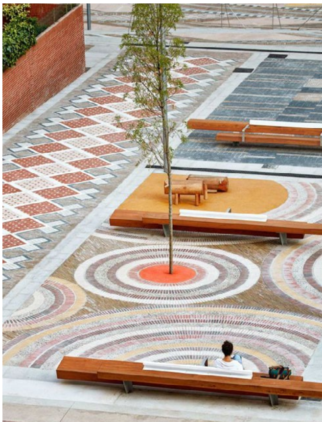
Refurbishment of Penedès Square in Cerdanyola del Vallès
