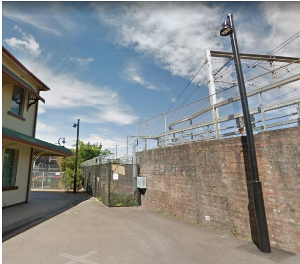
Figure 3-2 Street lighting adjacent to rail corridor (Google Maps photo, located at South Eveleigh near MacPherson Greenleaf adjacent to Redfern Station)
