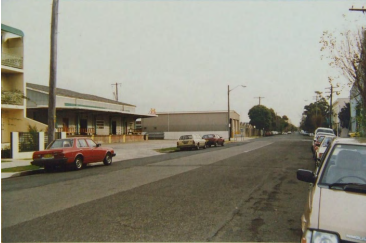
Figure 3.40: View west along Wilson Street, c1980-1989. Former Parcels Depot and Fire Shed on left of image (Source: City of Sydney Archives [A-00019541]. https://archives.cityofsydney.nsw.gov.au/nodes/view/580186 )
