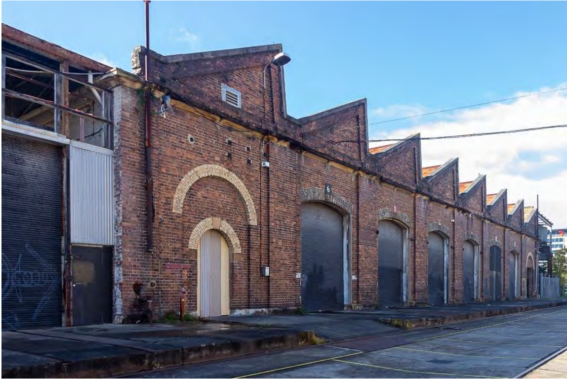
Figure 4.6: Paint Shop western elevation from Traverser No.1 (Source: Curio 2021)
