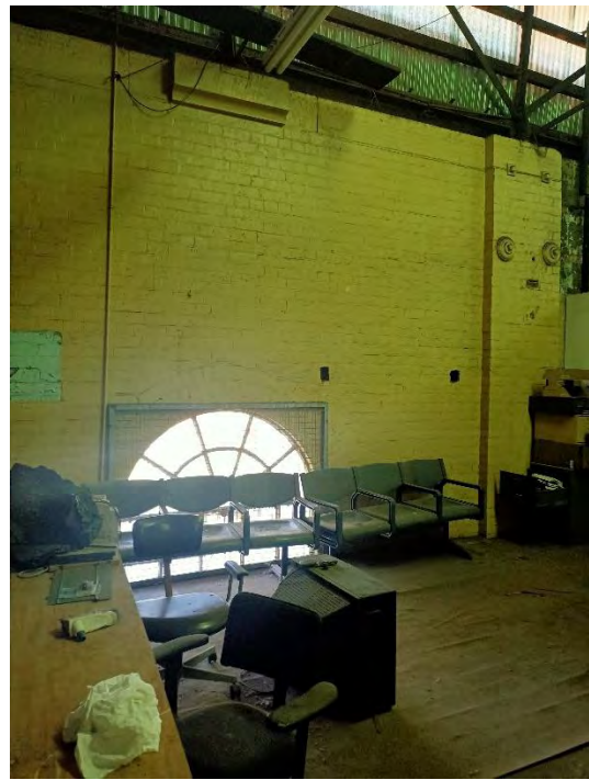
Figure 4.18: Office space in south-west Mezzanine (Track 0) (Source: Curio 2021)
