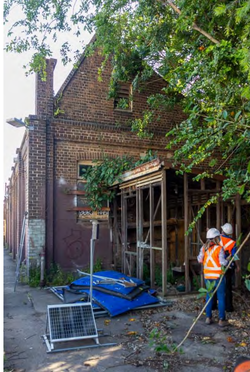
Figure 4.100: View west along path from Platform 1 of Redfern Station to eastern wall of the TEC (Source: Curio 2021)
