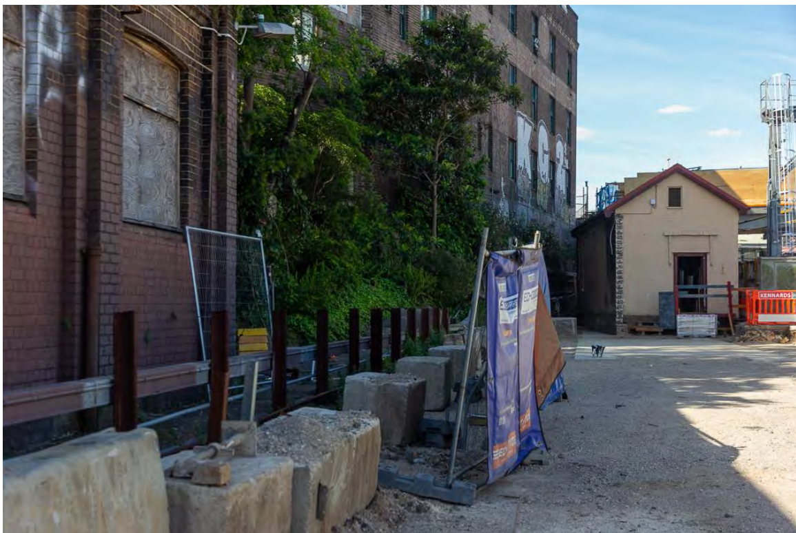
Figure 4.141: Northern eastern view of Platform level 1 building and TEC (Source: Curio 2021)
