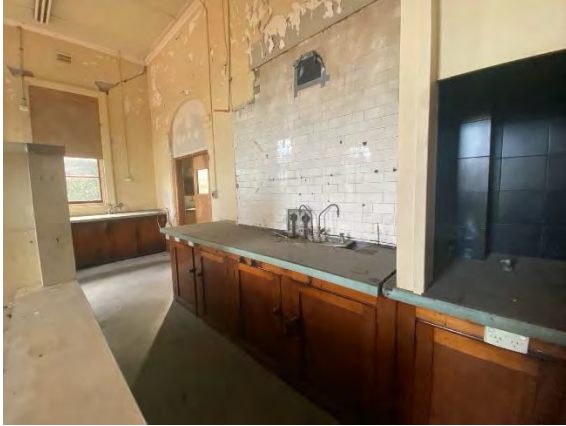
Figure 4.76: Laboratory room on first floor of building (Source: Curio 2021)
