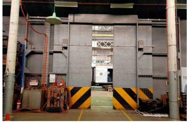
Figure 4.16: Modern central dividing wall between northern and tracks and southern Tracks 0-1 (Source: Curio 2021)
