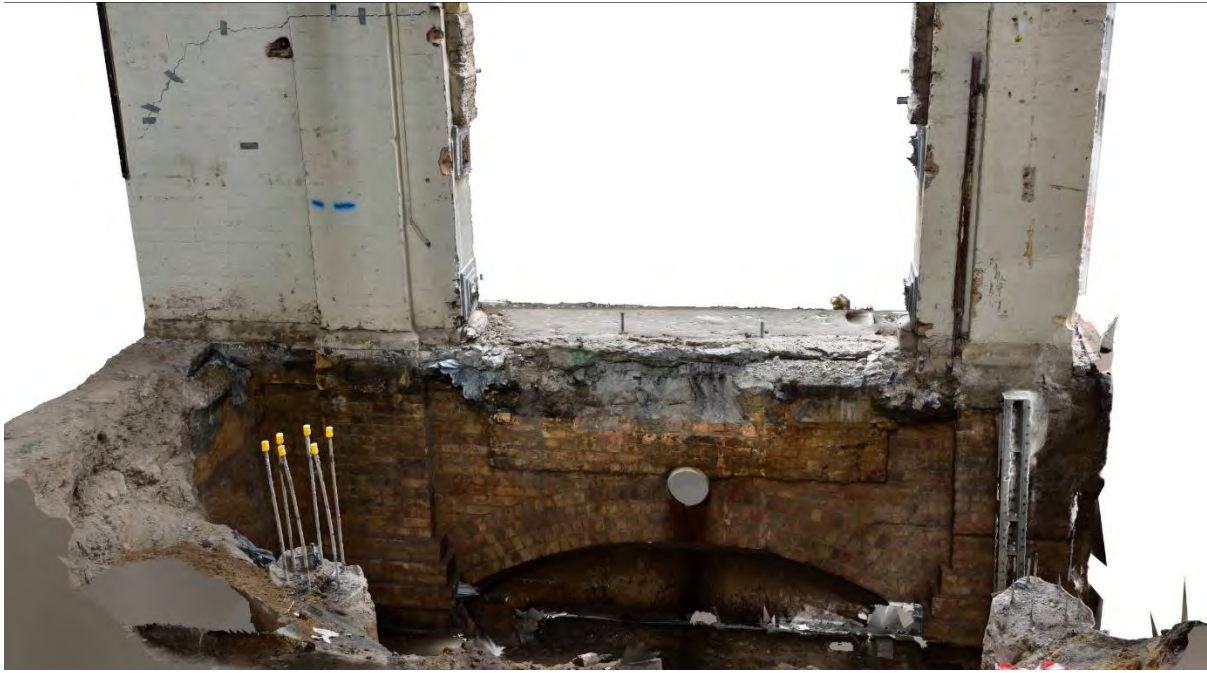
Figure 5.4: Photogrammetry model of Brick footings and arch of Locomotive Workshops uncovered and recorded during archaeological monitoring of construction works (Source: Curio 2019)
