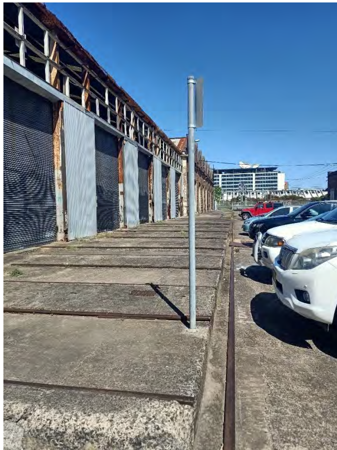
Figure 4.27: Western elevation of the Former Car Suburban Workshops. Original Paint Shop visible in background and location of Traverser No.1 in the background to the right (Source: Curio 2021)
