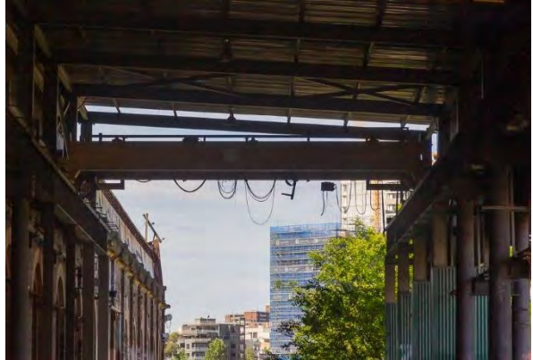
Figure 4.24: Close up of Crane in situ within the Southern Annex (Source: Curio 2021)
