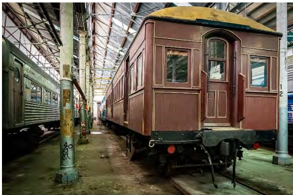
Figure 4.12: Carriages stored on the roads within the Paint Shop building, view east (Source: Curio 2021)
