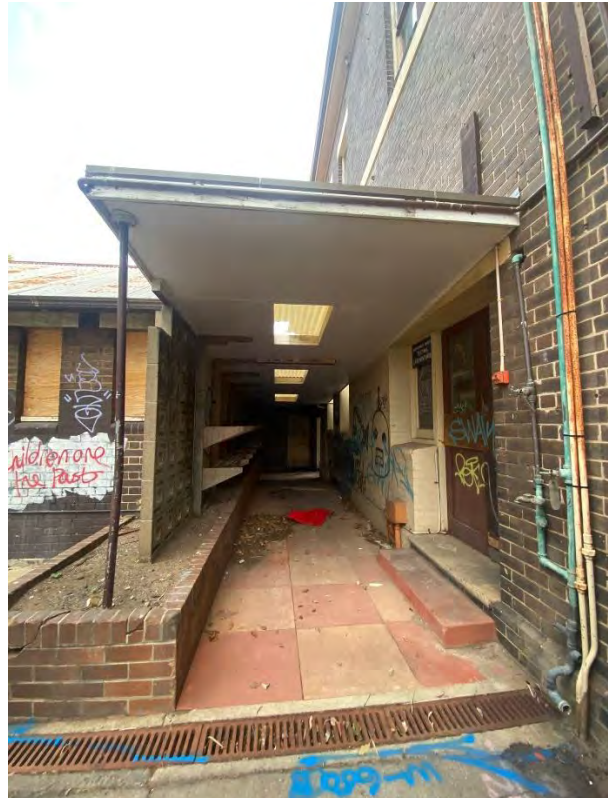
Figure 4.73: Southern view of passageway between the Scientific Services Building No.1 and the CME Toilet Block towards the Scientific Services Building No.2 Entrance (Source: Curio 2021)
