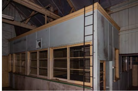
Figure 4.121: Western view of the internal walls abutting the interior fine joinery walls (Source: Curio 2021)
