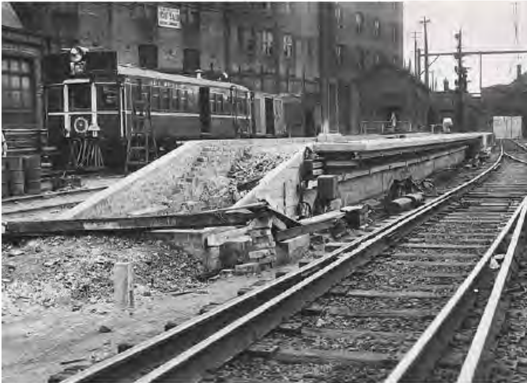
Figure 3.35: 'Elston's Sidings' adjacent to Redfern Railway Station, 1956. (Source: State Rail Authority Archives Photographic Reference Print Collection, 16)
