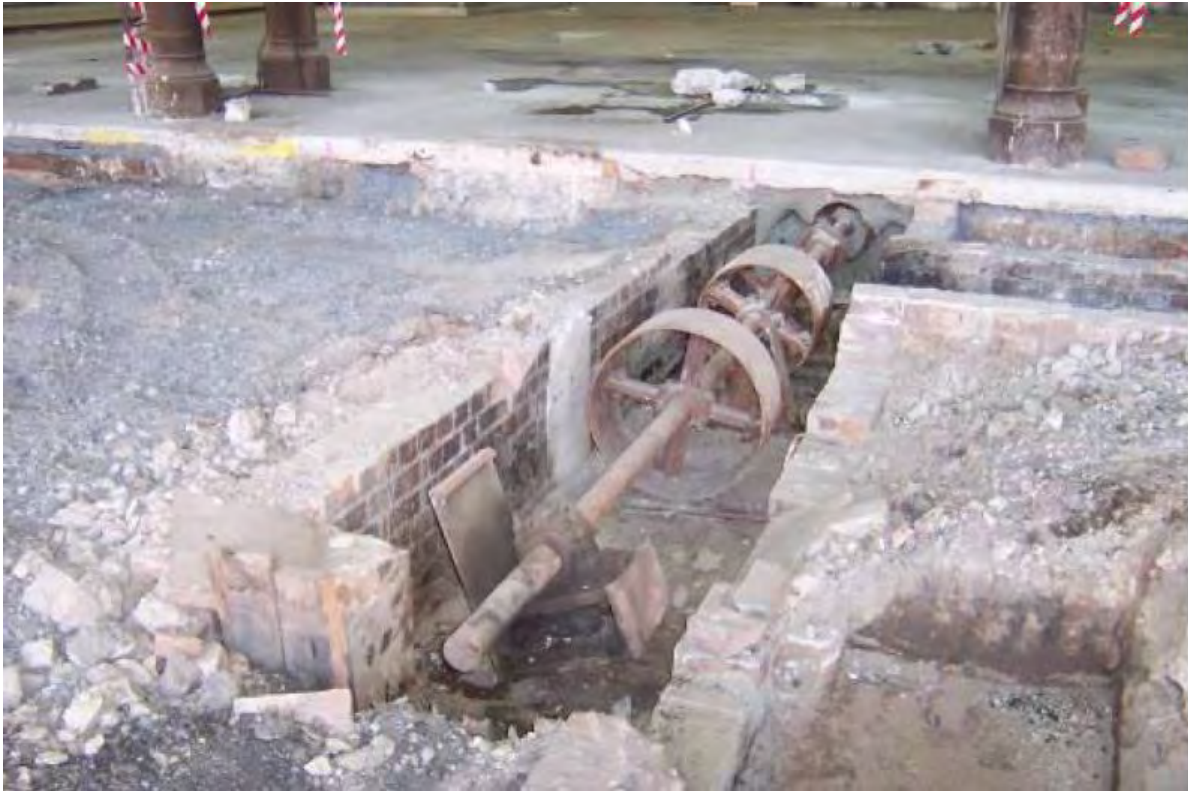
Figure 5.5: Example of brick pits and machinery (a line or counter shaft) uncovered beneath the floor of the Carriage Workshop building during archaeological monitoring and investigation works in 2004 (Source: AHMS 2008: 17)
