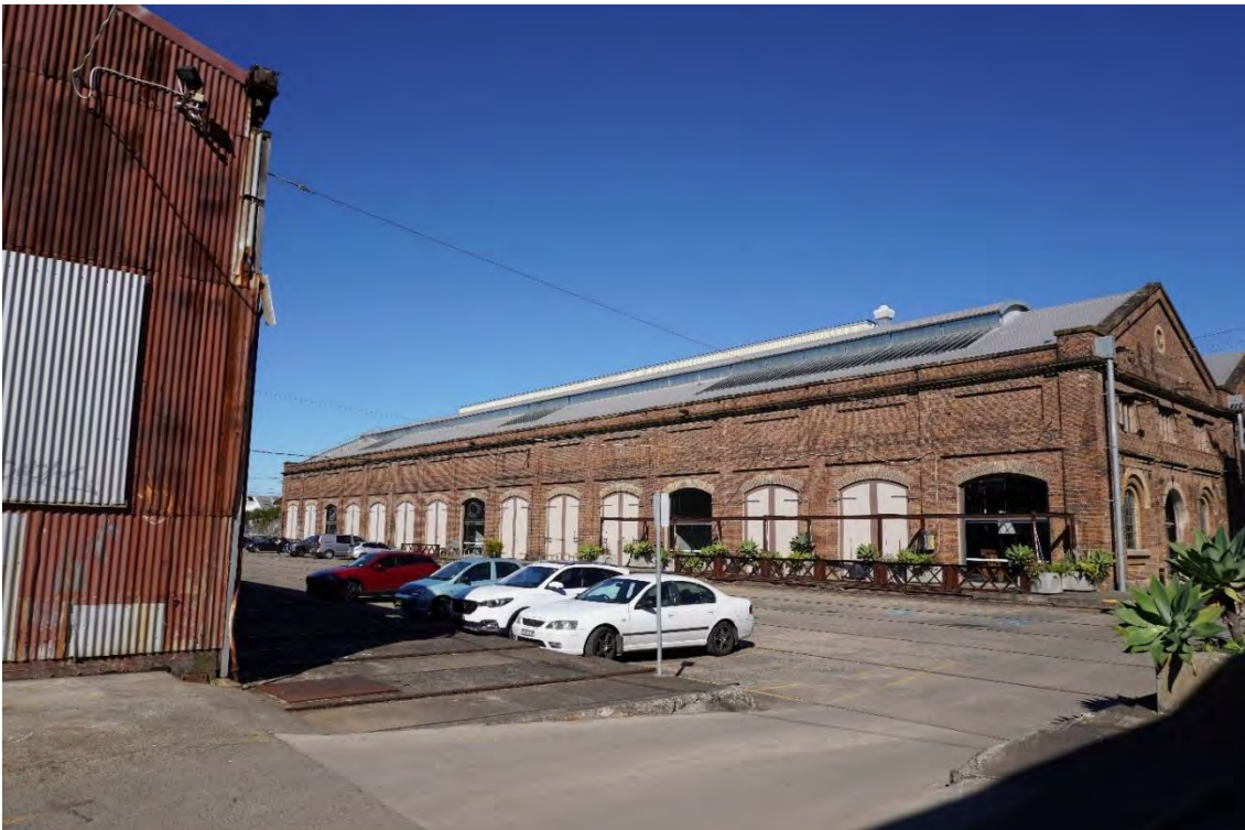
Figure 4.187: South western view from the north of the Former Suburban Car Workshops towards Carriageworks and Traverser No.1 (Source: Curio 2021)
