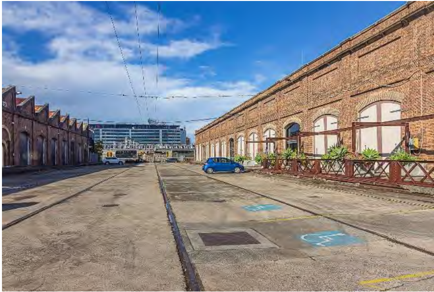
Figure 4.2: View south across Traverser No. 1 square, the eastern façade of the Carriage Workshops building to the right, the Paint Shop to the left (Source: Curio 2021)
