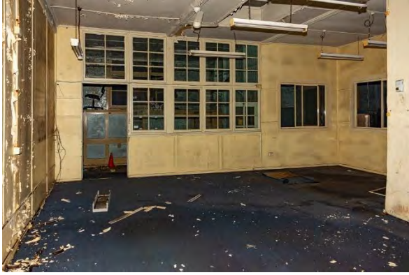
Figure 4.113: Northern view of internal walls in western half of the TEC and damage to walls and floor (Source: Curio 2021)
