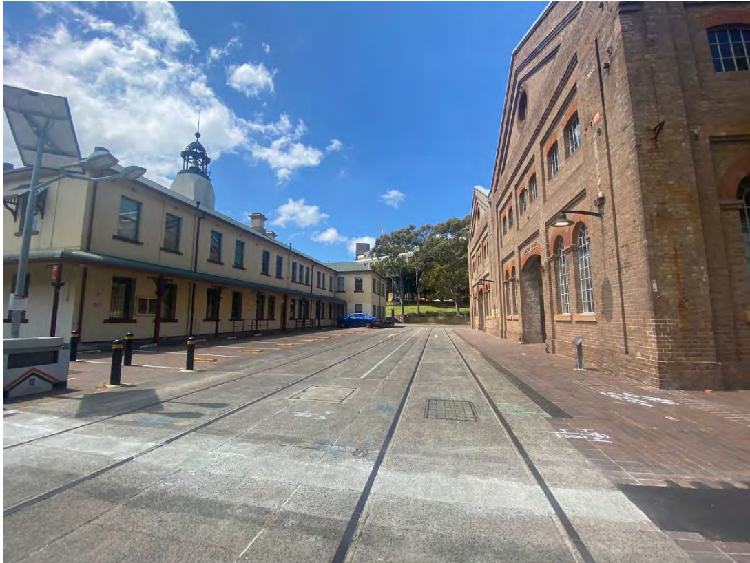
Figure 4.154: South eastern view of the Work Manager's and Timekeepers Office and New Locomotive Workshops (Source: Curio Projects)
