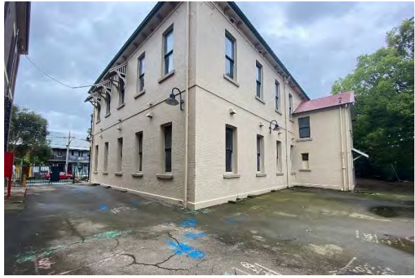
Figure 4.51: CME Exterior view north of the southern and western building façades (Source: Curio 2021)
