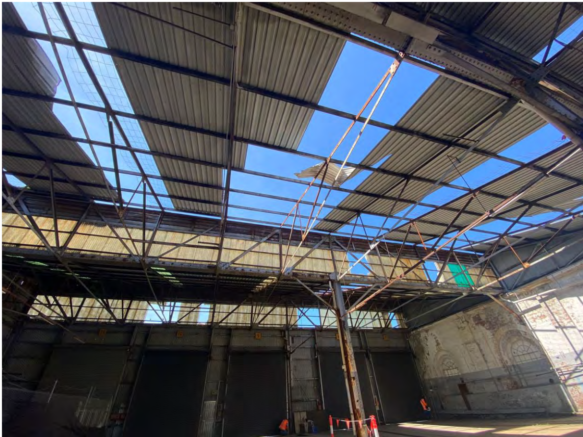
Figure 4.36: Condition of the former Suburban Car Workshops Roof (Source: Curio 2021)
