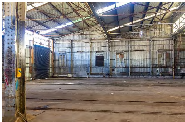
Figure 4.31: Interior of the former Suburban Car Workshops, view north (Source: Curio 2021)
