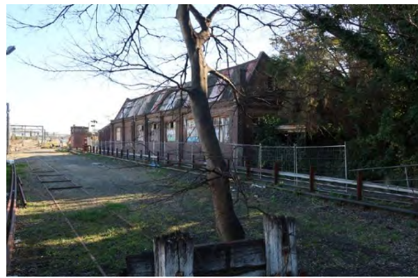
Figure 4.138: 2017 Western view of Head Shunt and overgrown tracks Elston’s Sidings and TEC in the background (Source: TZG Architects 2017)
