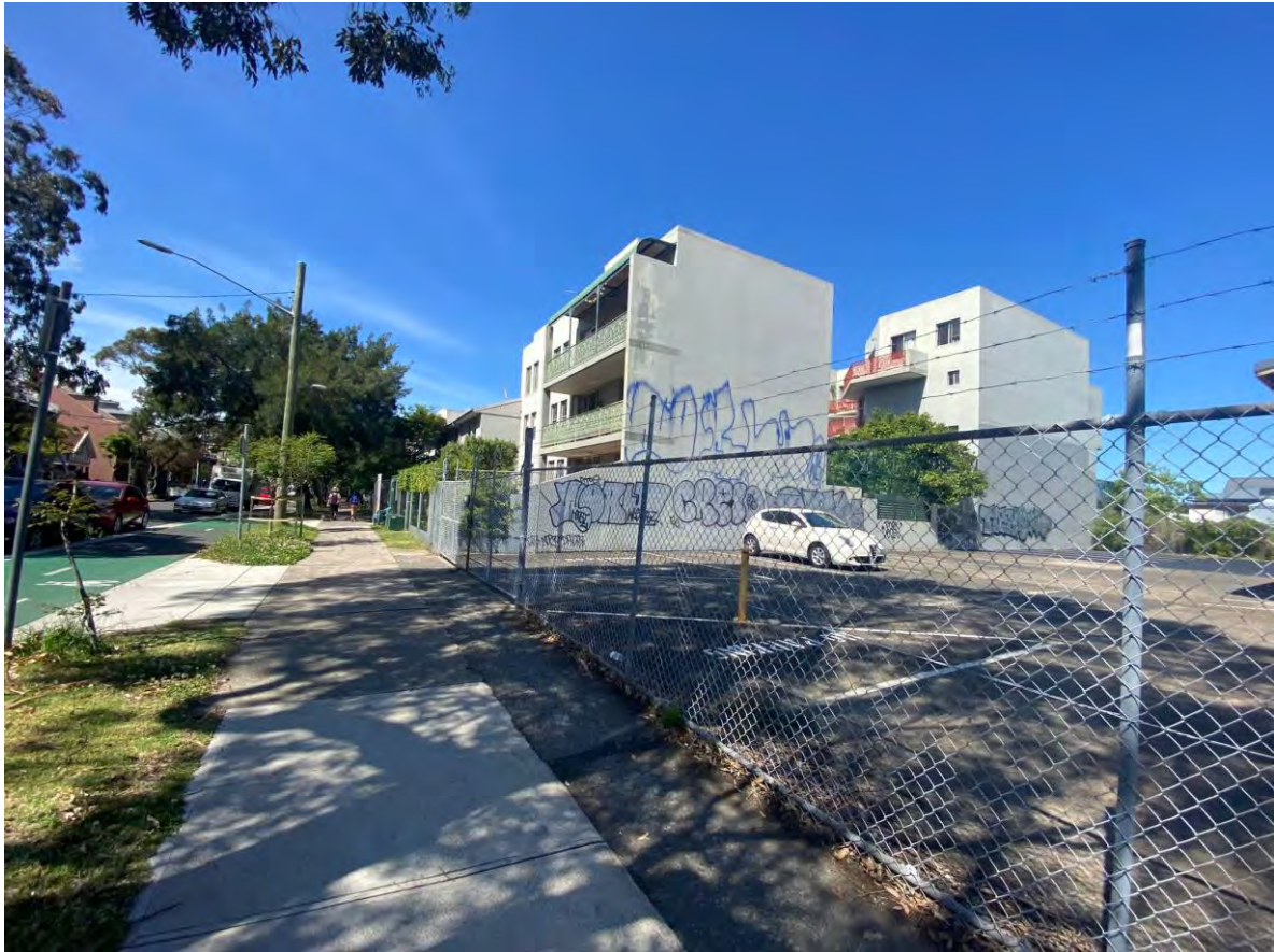
Figure 4.167: Eastern view down Wilson Street near the residential apartments abutting the subject site (Source: Curio Projects)
