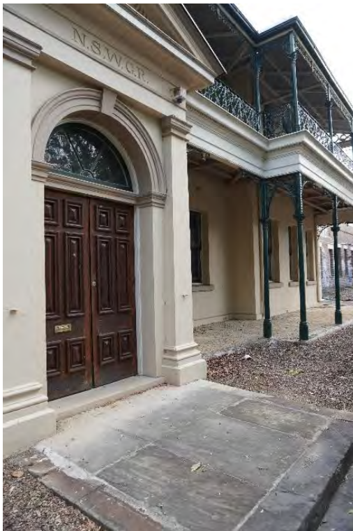
Figure 4.38: Front door of CME Building along Wilson Street (Source: Curio 2021)
