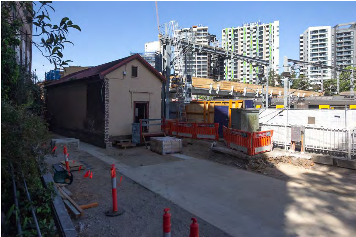
Figure 4.140: Eastern view of Platform 1 building and slab where the Platform 1 building will be moved as part of the Redfern Station Southern Access project (Source: Curio 2021)
