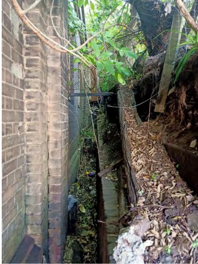
Figure 4.104: North eastern facing facade of the TEC adjacent to the precinct retaining wall (Source: Curio 2021)
