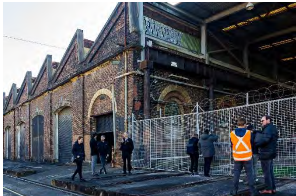
Figure 4.8: North eastern view of the Paint Shop building and carriage lifting crane annexe adjacent to the southern façade (Source: Curio 2021)
