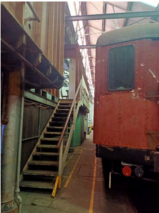
Figure 4.17: Mezzanine in south-west (Track 0) (Source: Curio 2021)
