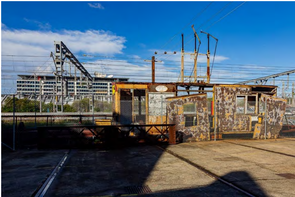
Figure 4.97: Southern view of Traverser No.1 (Source: Curio 2021)
