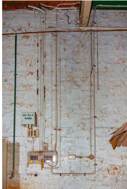
Figure 4.127: Service lines on internal south eastern wall of TEC (Source: Curio 2021)
