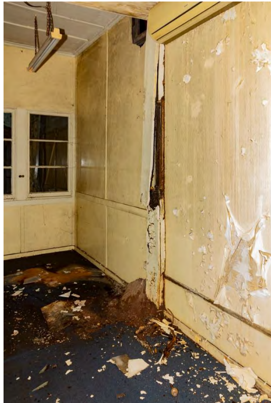
Figure 4.133: Damage to structural columns and floor in TEC office space (Source: Curio 2021)
