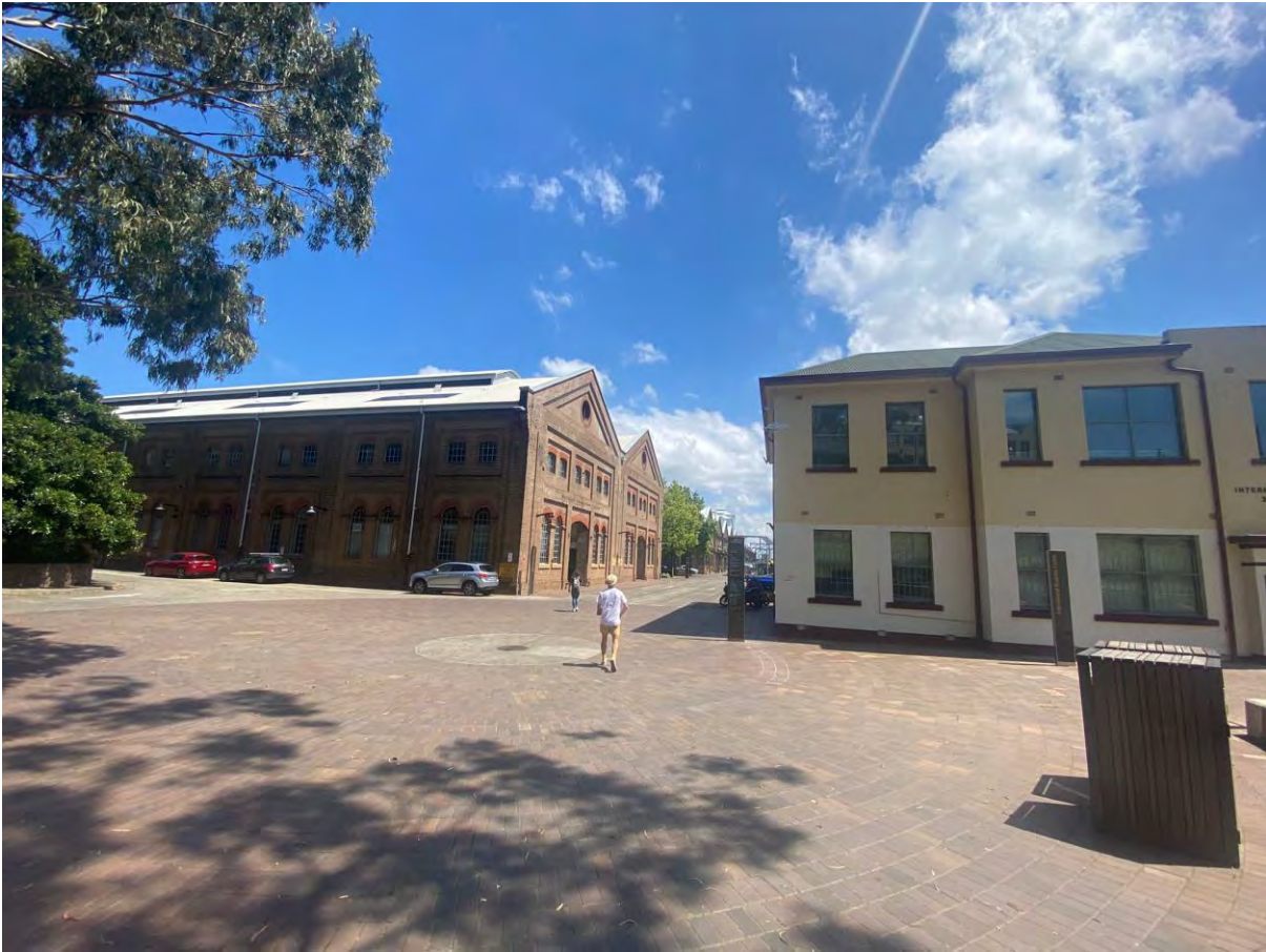
Figure 4.156: Western view with the Work Manager's and Timekeepers Office and New Locomotive Workshops in the foreground and the Locomotive Workshops in the background (Source: Curio Projects)
