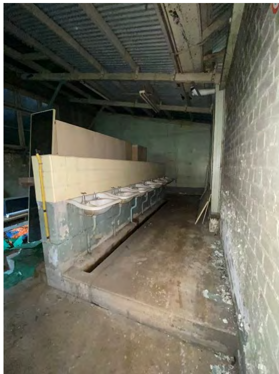
Figure 4.119: South western view of the modern annex and infill between the northern toilet block and TEC with the surviving early urinal (Source: Curio 2021)
