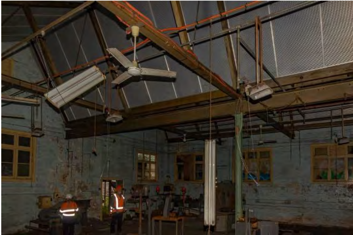
Figure 4.134: Eastern view of the north eastern interior corner of the TEC original workshop area (Source: Curio 2021)
