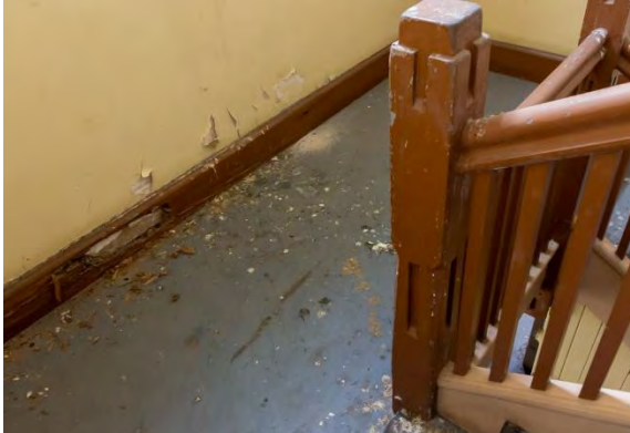
Figure 4.82: Termite damage to a skirting board along the staircase in the Scientific Services Building No.1 (Source: Curio 2021)
