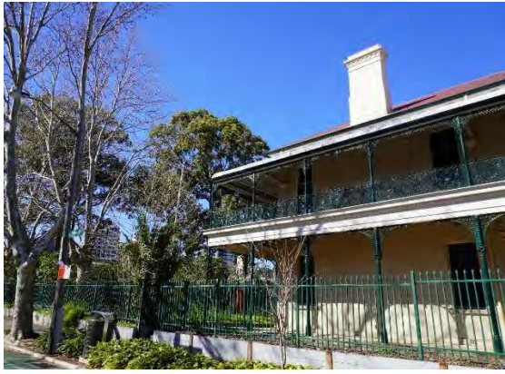
Figure 4.50: View southeast of the northern façade and verandah of the CME Building along Wilson Street and CME gardens (Source: Curio 2021)
