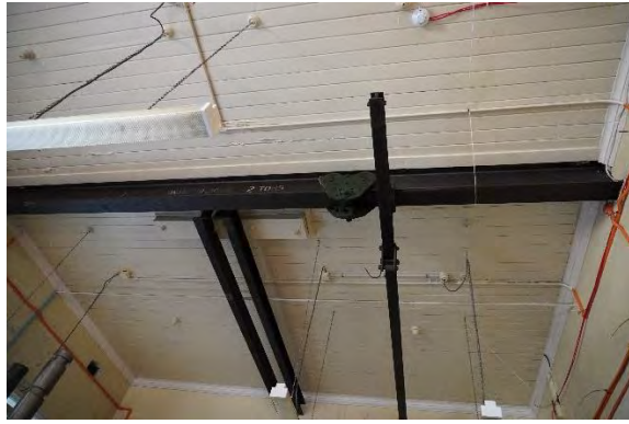
Figure 4.91: Ceiling of room in ground floor of Scientific Services Building No.1 with crane in situ (Source: Curio 2021)
