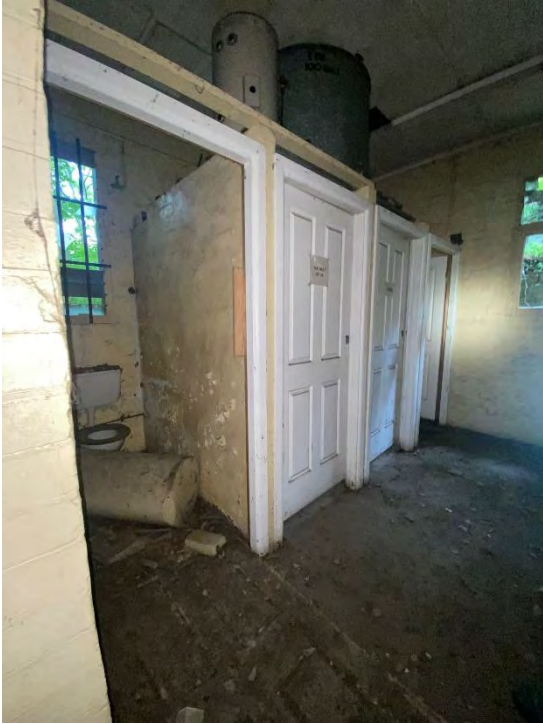
Figure 4.130: North western view of toilet cubicles in northern toilet block (Source: Curio 2021)
