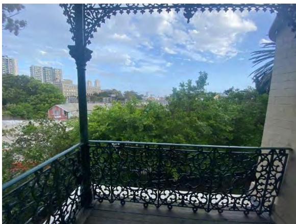
Figure 4.60: View from CME Building level one verandah along eastern façade facing south toward South Eveleigh (Source: Curio 2021)
