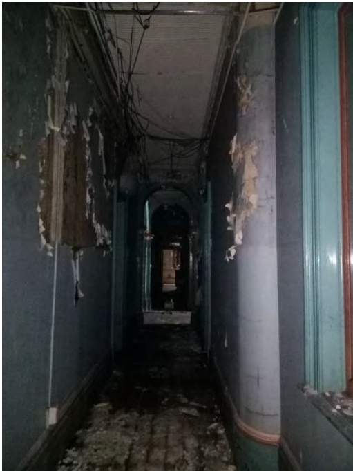
Figure 4.48: Intrusive surface mounted electrical elements, water damage and lead painted walls (Curio 2021)
