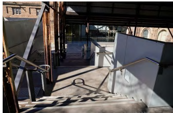
Figure 4.148: View south down Wilson Street Stairs towards Carriage Workshops building (Source: Curio 2021)
