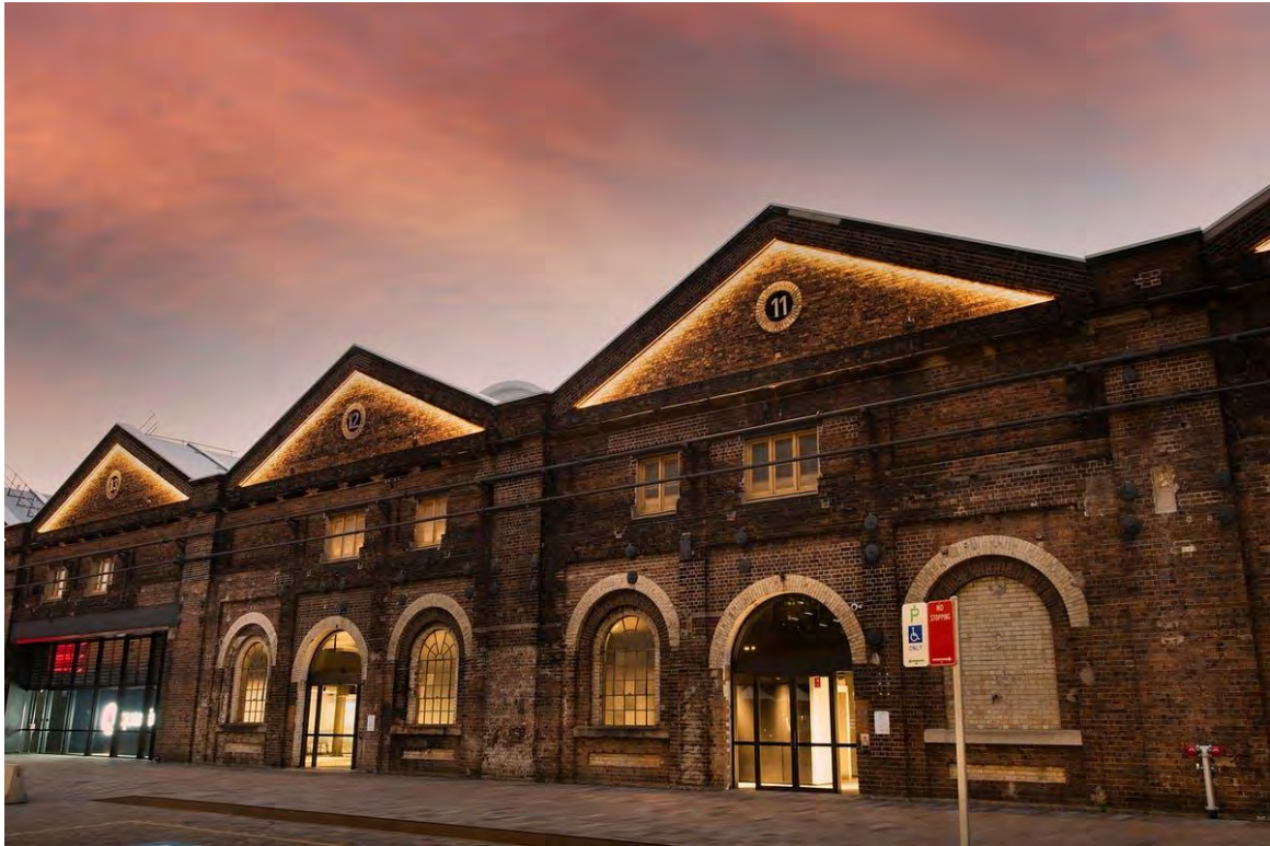
Figure 4.152: North western view of the southern façade outside Bays 11, 12 and 13 at the Locomotive Workshops in South Eveleigh (Source: Sissons)
