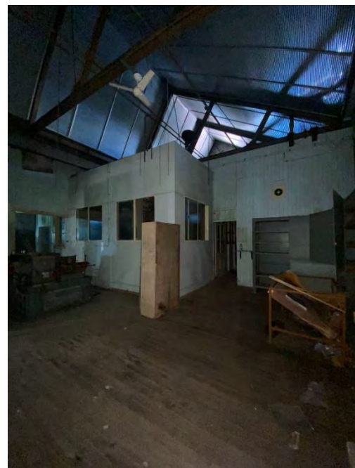
Figure 4.110: South western view of internal walls within the TEC (Source: Curio 2021)
