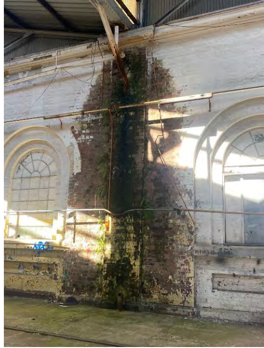
Figure 4.35: Condition of Northern Wall of the Paint Shop (Source: Curio 2021)
