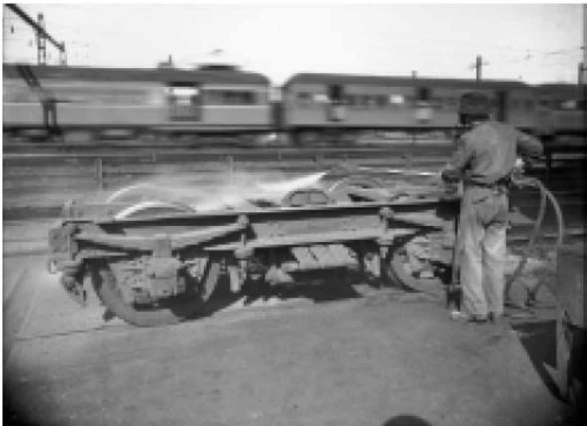
Figure 3.33: View of a bogie being cleaned outside the Paint Shop and Carriage Workshop, undated (Source: SRAO)
