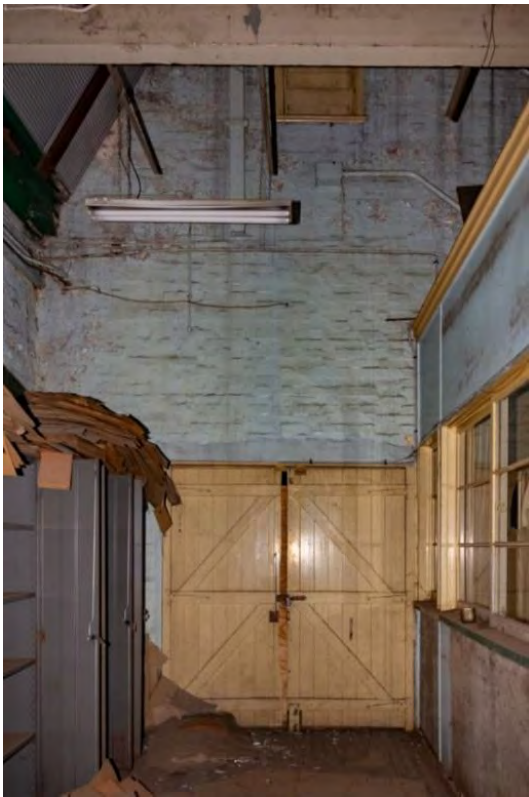
Figure 4.115: South western façade entrance of the TEC and exposed interior walls (Source: Curio 2021)
