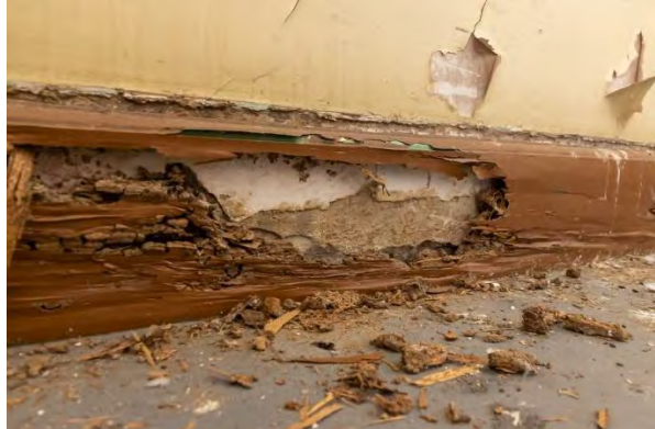
Figure 4.83: Termite damage to a skirting board along the staircase in the Scientific Services Building No.1 (Source: Curio 2021)
