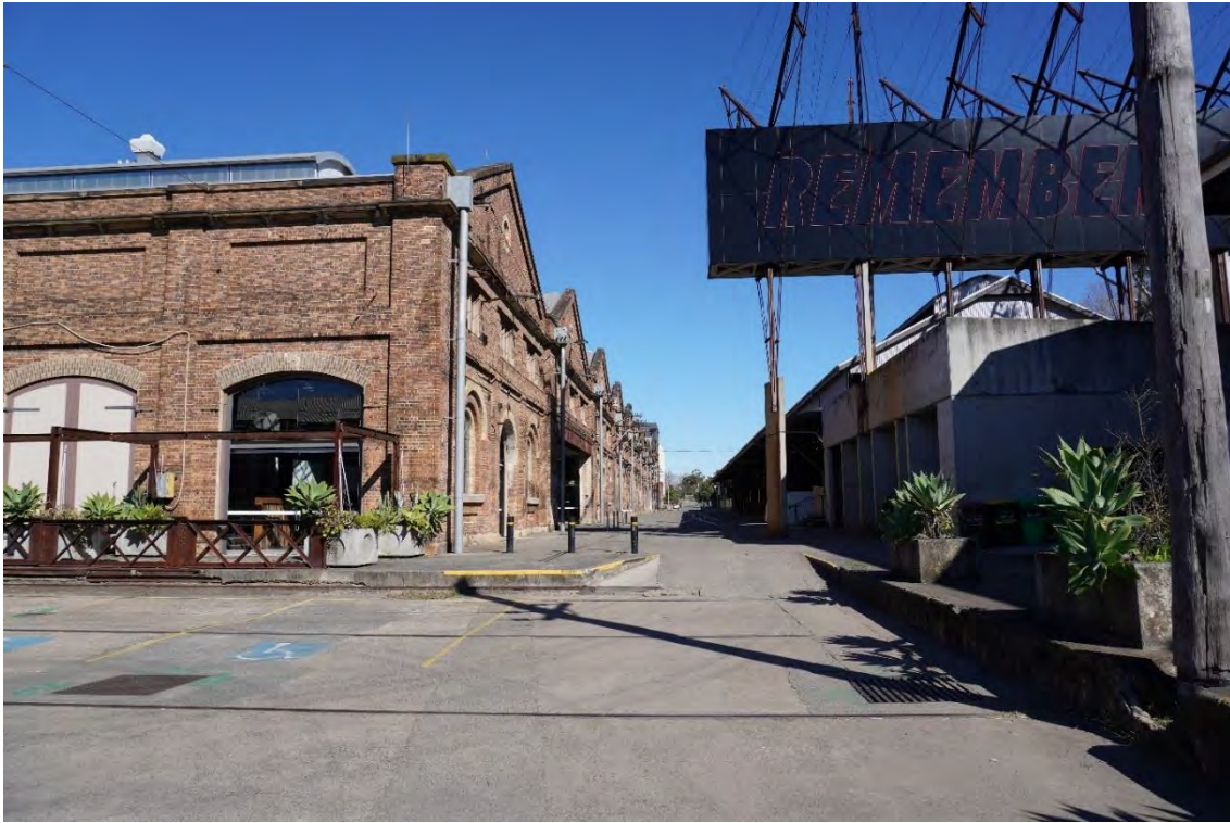
Figure 4.188: Western view of the Carriageworks building and Traverser No.1 along the western boundary of our subject site (Source: Curio 2021)
