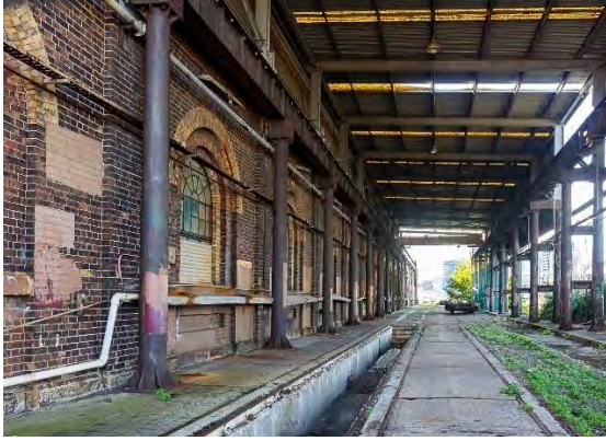
Figure 4.23: View east along the southern façade of the Paint Shop, within the southern annexe for the Carriage lifting crane (Source: Curio 2021)
