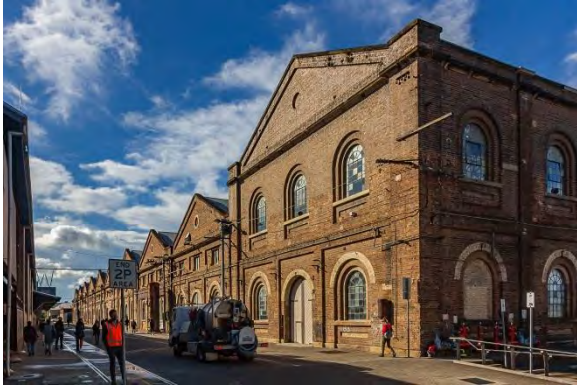
Figure 4.143: Eastern view of the western façade of the Carriageworks building from Carriageworks Way (Source: Curio 2021)
