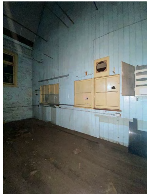
Figure 4.136: Northern internal wall Store Room from the main work area in the TEX (Source: Curio 2021)
