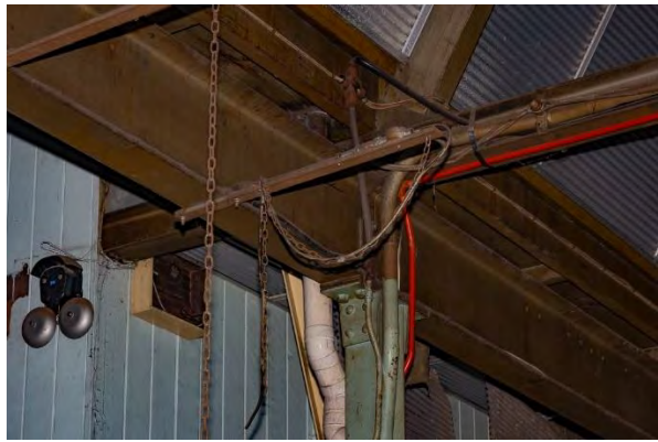
Figure 4.123: Steel roof beams with modern service lines (Source: Curio 2021)
