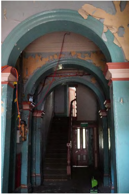
Figure 4.40: Entrance Hall from the Wilson Street entrance on the ground floor level, showing the staircase in the background (Source: Curio 2021)
