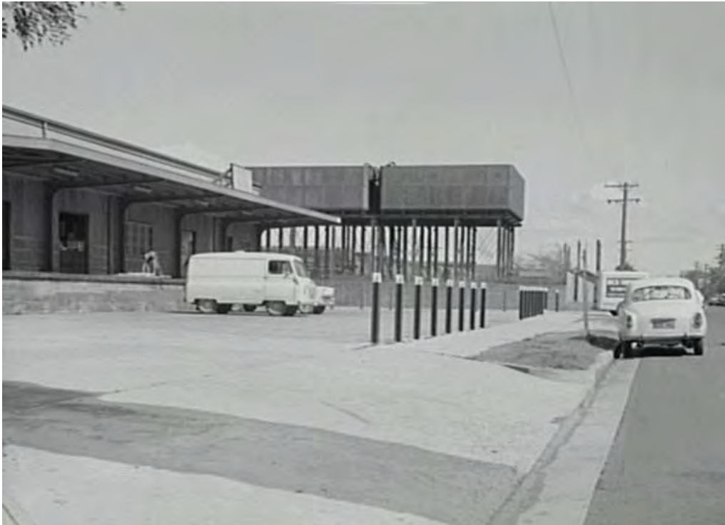
Figure 3.39: Railways Parcel Office, Wilson Street Darlington, 1963. View SW along Wilson Street. Former water tanks (now demolished) visible in background (Source: City of Sydney Archives, [A-00045917] https://archives.cityofsydney.nsw.gov.au/nodes/view/687625 )
