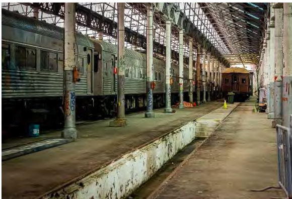
Figure 4.11: View east along one of the internal 'roads' within the Paint Shop Building (Source: Curio 2021)
