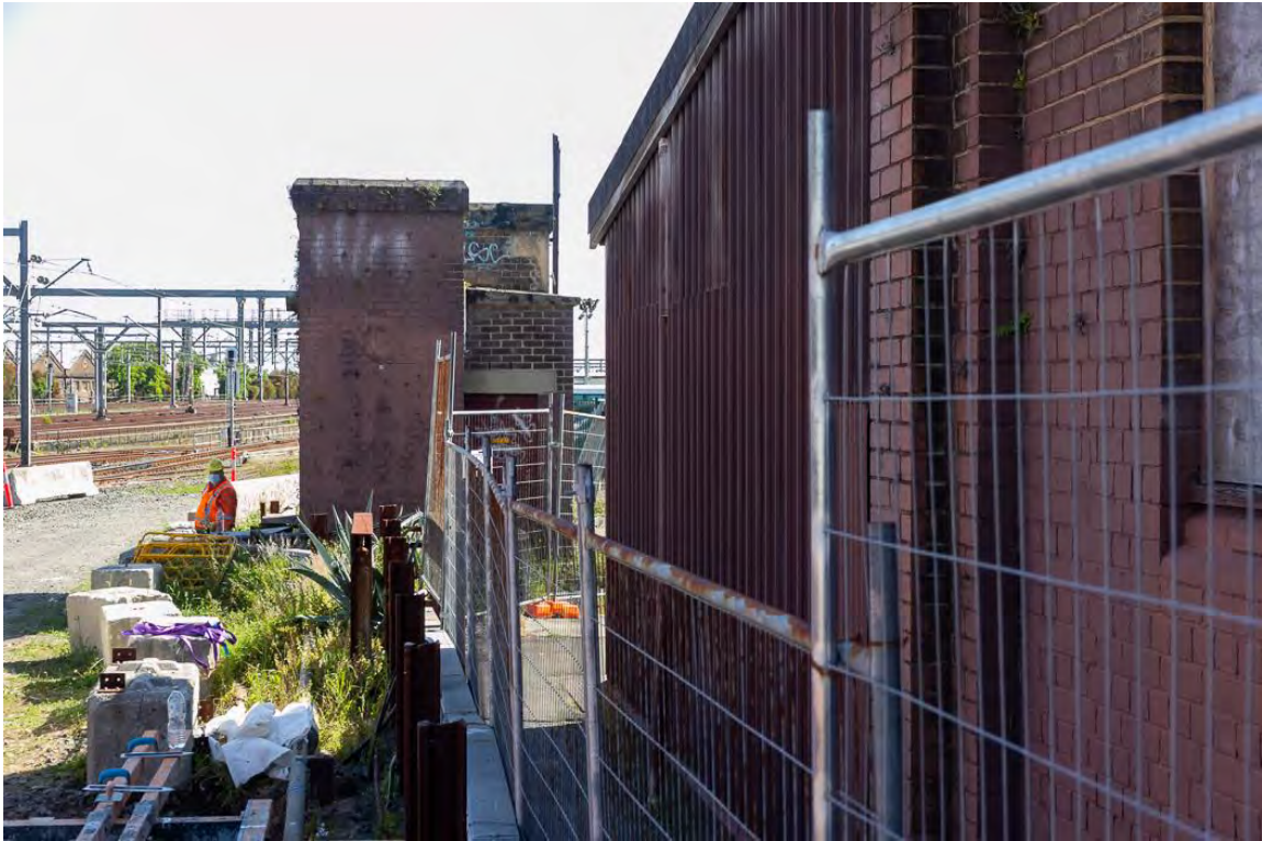
Figure 4.102: South western view of the south eastern corner of the TEC in the foreground and the Overbridge Footing in the background (Source: Curio 2021)
