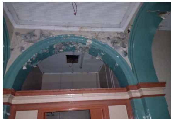
Figure 4.43: Example of degrading interior condition exhibiting water damage, mould, peeling lead paint, within CME Building (Source: Curio 2021)
