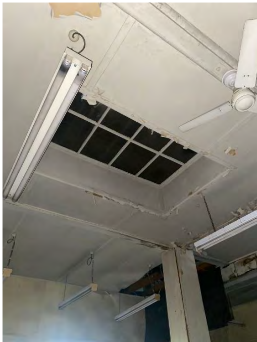
Figure 4.135: Skylight in Supervisors Office (Source: Curio 2021)
