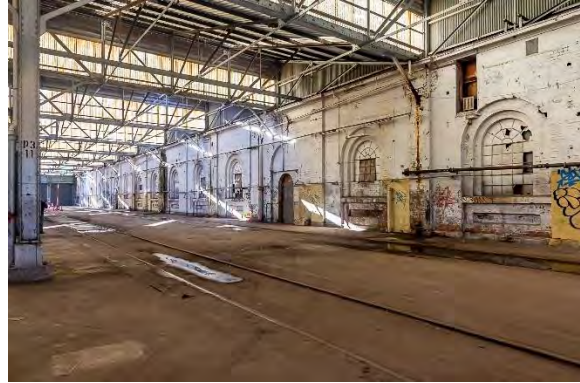
Figure 4.10: Paint Shop northern façade, now forming interior wall with the northern Paint Shop Extension (former Suburban Car Workshops) (Source: Curio 2021)
