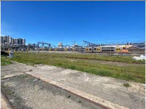
South eastern view across Fan of Tracks towards South Eveleigh (Source: Curio 2021)
