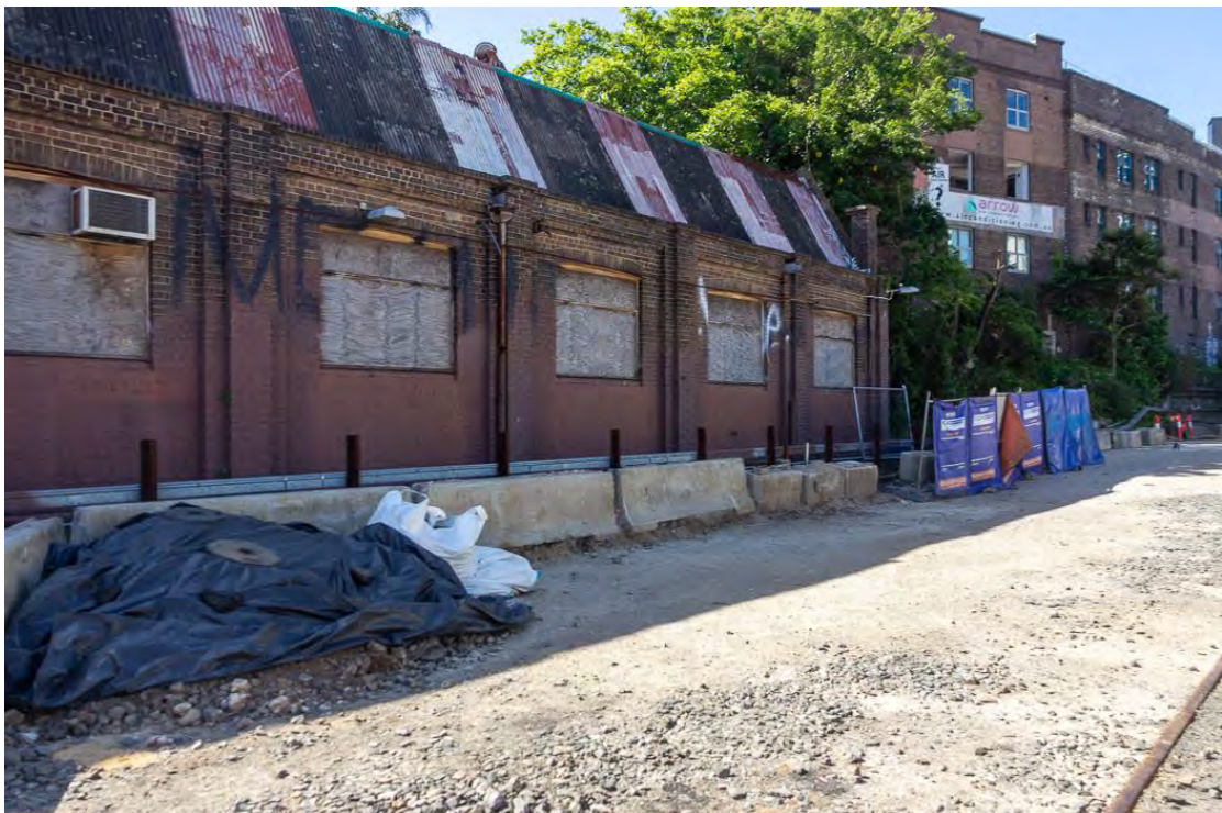
Figure 4.101: Northern view of the TEC from previous area of Elston's Sidings (Source: Curio 2021)
