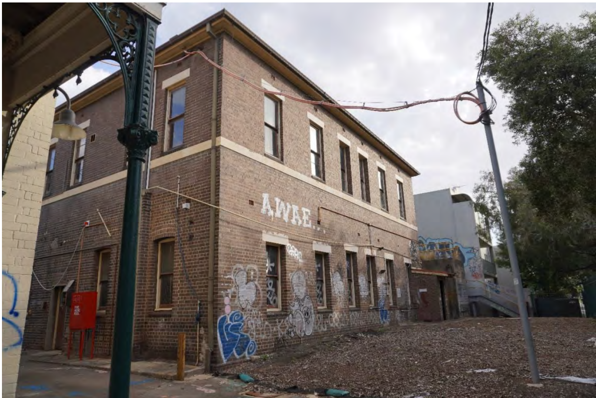
Figure 4.63: South western view from Wilson Street of the Scientific Services Building No.1 northern façade (Curio 2021)
