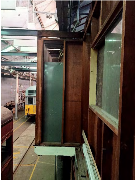
Figure 4.19: Mezzanine insert in south-west (Track 0) (Source: Curio 2021)
