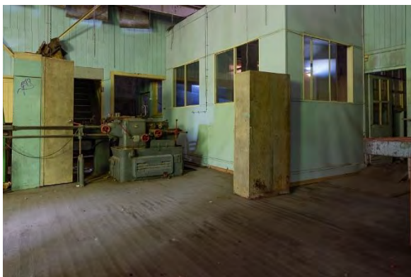
Figure 4.111: Southern view of internal walls within the TEC and insitu machinery (Source: Curio 2021)
