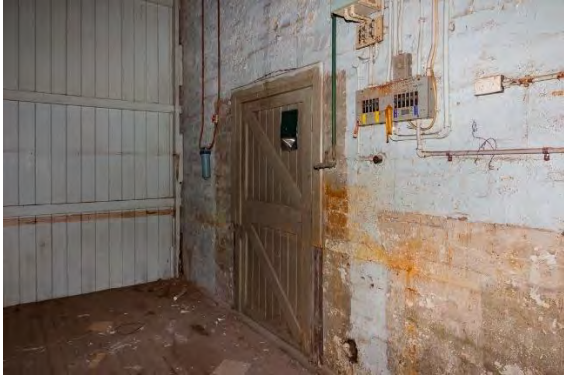
Figure 4.120: Eastern view of the south east entrance to the TEC with interior fine joinery walls in background (Source: Curio 2021)
