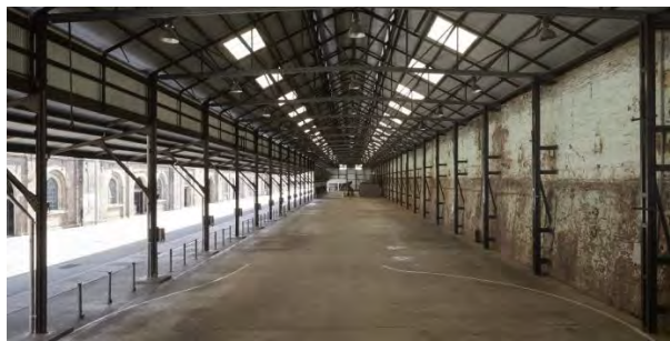
Figure 4.146: Interior of Blacksmith Workshop, view west. Original northern masonry wall to right, opening along southern façade towards Carriage Workshops (Source: Eveleigh Stories)
