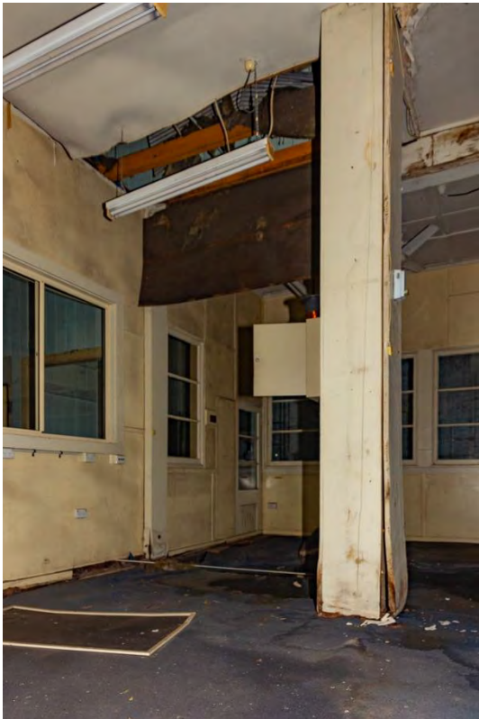
Figure 4.132: Collapsing roof and modern lighting in TEC office space (Source: Curio 2021)
