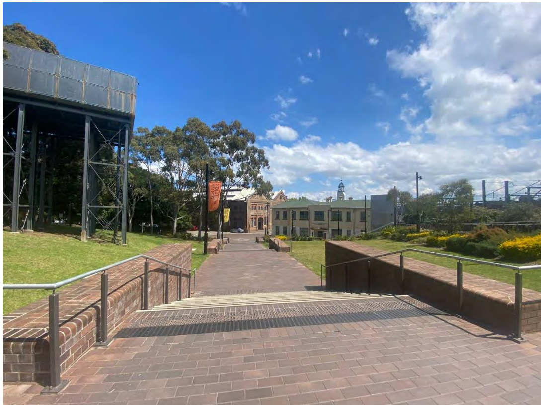
Figure 4.155: South western view from Cornwallis Street towards the Water Tower, Work Manager's and Timekeepers Office and New Locomotive Workshops (Source: Curio Projects)
