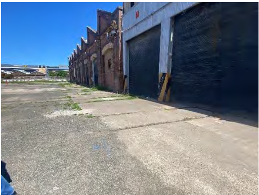
Southern view of Fan of Tracks connecting with the Paint Shop and Former Suburban Car Workshops (Source: Curio 2021)
