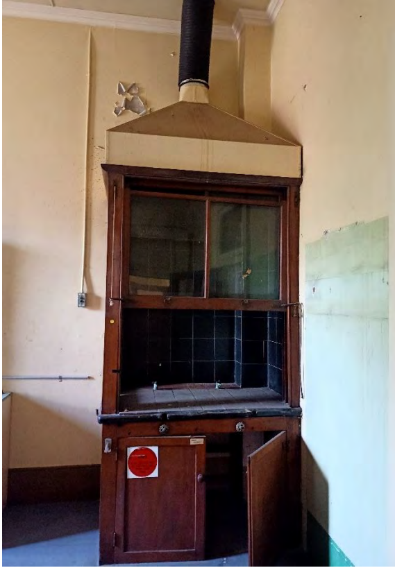
Figure 4.86: Exhaust cabinet on the first floor of the Scientific Services Building No.1 (Source: Curio 2021)
