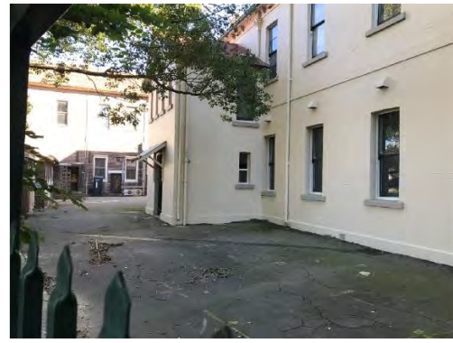
Figure 4.53: View west across the southern façade of the CME Building, Scientific Services Building No.1 visible in the background (Source: RPS Group)
