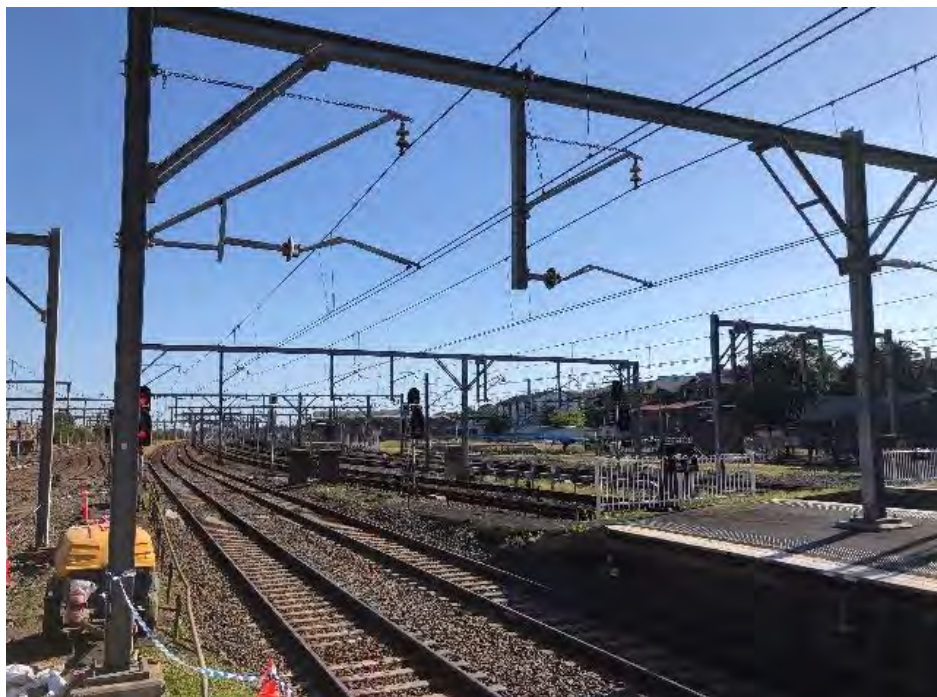
Figure 4.179: View from Redfern Station northwest to Paint Shop Sub-Precinct (Source: Curio 2020)
