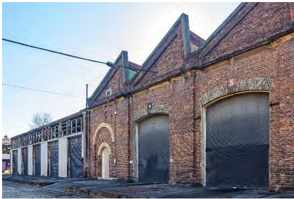
Figure 4.7: Paint Shop western elevation, 1912 Paint Shop Extension (former Suburban Car Workshops) visible in the background (Source: Curio 2021)
