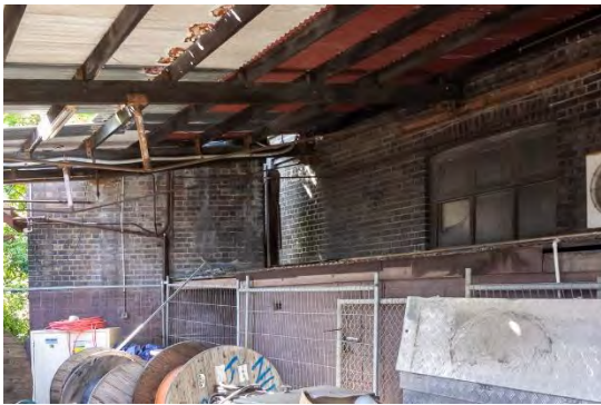
Figure 4.105: Northern view of the western façade of the TEC with attached awning and Overbridge Footing in the background (Source: Curio 2021)
