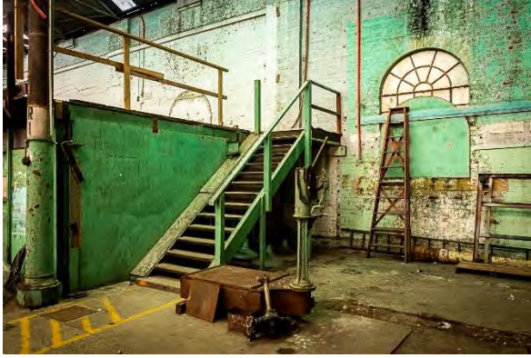
Figure 4.15: Stairs in northeast of Paint Shop, Track 6a to mezzanine along northern wall (Source: Curio 2021)
