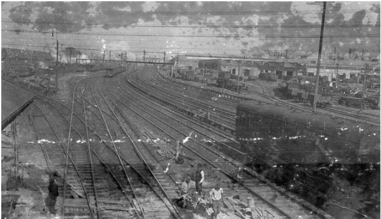
Figure 3.27: Taken from the southern end of Redfern Station c1912, south along main rail line towards Carriage Workshops (North Eveleigh in right of image). The sawtooth roof of the Paint Shop can be seen in the midground/right of the image (Source: SRAO)
