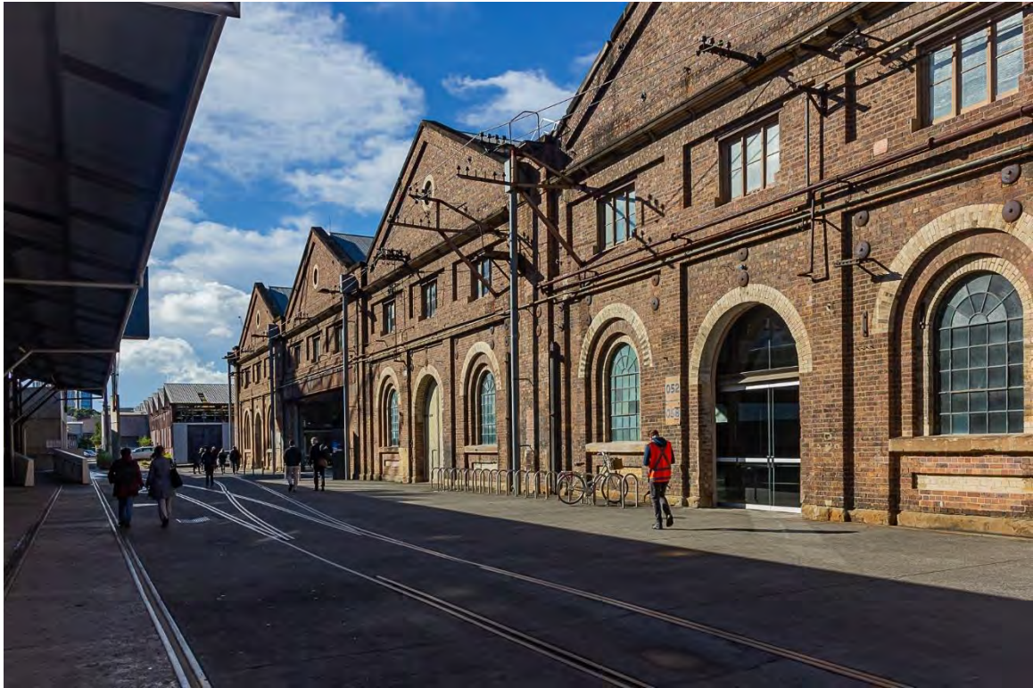
Figure 4.191: Eastern view towards the Former Suburban Car Workshops and Traverser No.1 from Carriageworks Way between Carriageworks and Blacksmiths Workshop (Source: Curio 2021)
