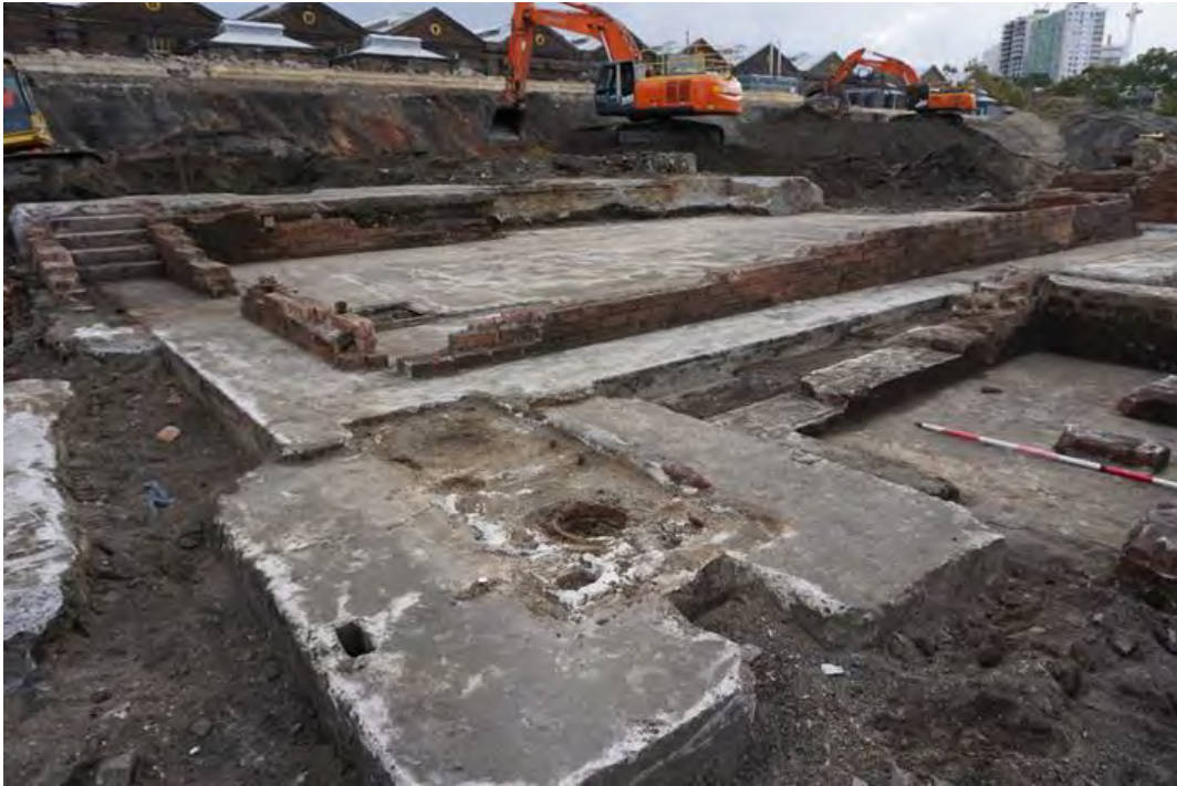
Figure 5.2: Example of structural remains of the former Foundry uncovered within the Building 2 footprint, archaeologically recorded during construction works (Source: Curio 2017)
