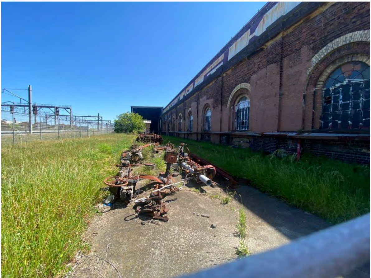
Figure 4.25: Paint Shop southern elevation, view west towards Carriage Lifting Crane annex (Source: Curio 2021)
