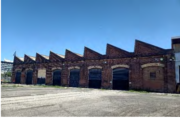
Figure 4.9: South western view of the Eastern façade of the Paint Shop (Source: Curio 2021)
