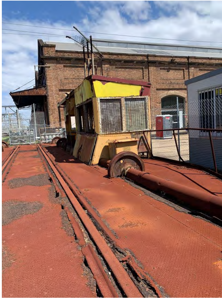
Figure 4.98: Western view of Traverser No.1 with Carriage Workshops in the background (Source: Curio 2021)
