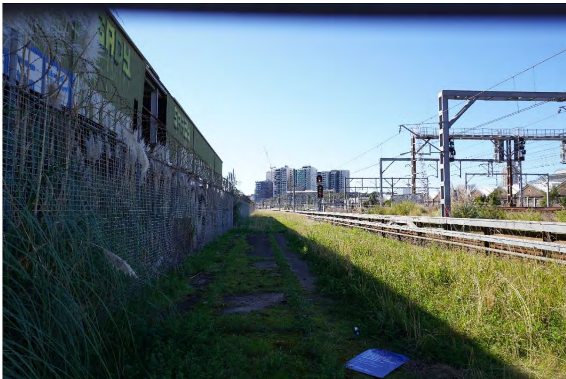
Figure 4.185: South eastern view along the southern boundary of the subject site south of the Paint Shop and Carriage Lifting Crane (Source: Curio 2021)
