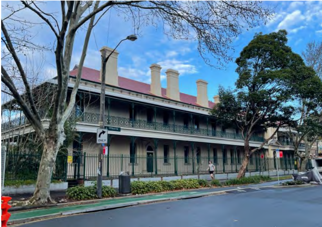
Figure 4.37: View south-west of the Chief Mechanical Engineer's office from Wilson Street (Source: Curio 2021)
