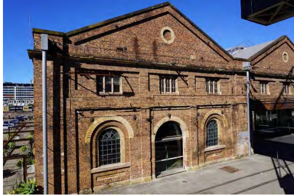
Figure 4.144: Southern view of the Carriage Workshops abutting the western boundary of the subject site (Source: Curio Projects)
