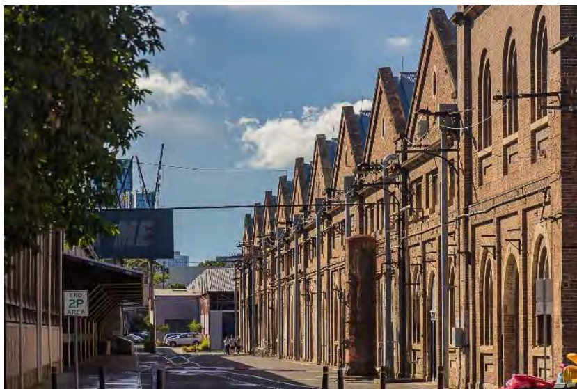
Figure 4.3: View east along Carriageworks Way towards Paint Shop Sub-Precinct, Paint Shop northern façade visible in the background. Northern façade of Carriage Workshops in right foreground of image, Blacksmith Workshop awning visible in left (Source: Curio 2021)
