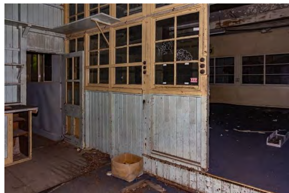
Figure 4.112: Eastern view of internal walls in the western half of the TEC (Source: Curio 2021)
