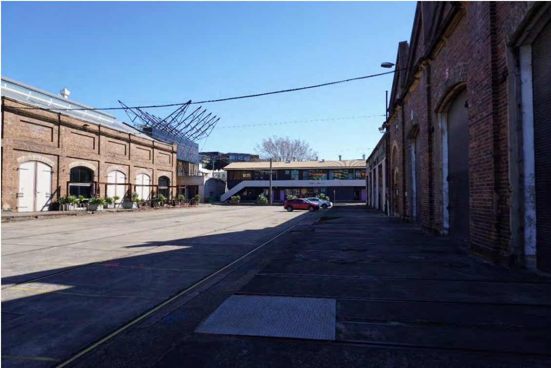
Figure 4.186: Northern view of the Carpenters, Plumbers and Food Distribution Building and Wilson Street Stairs from the Paint Shop (Source: Curio 2021)
