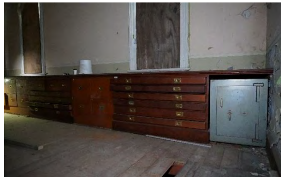
Figure 4.43: Example of degrading interior condition exhibiting water damage, mould, peeling lead paint, within CME Building (Source: Curio 2021)
