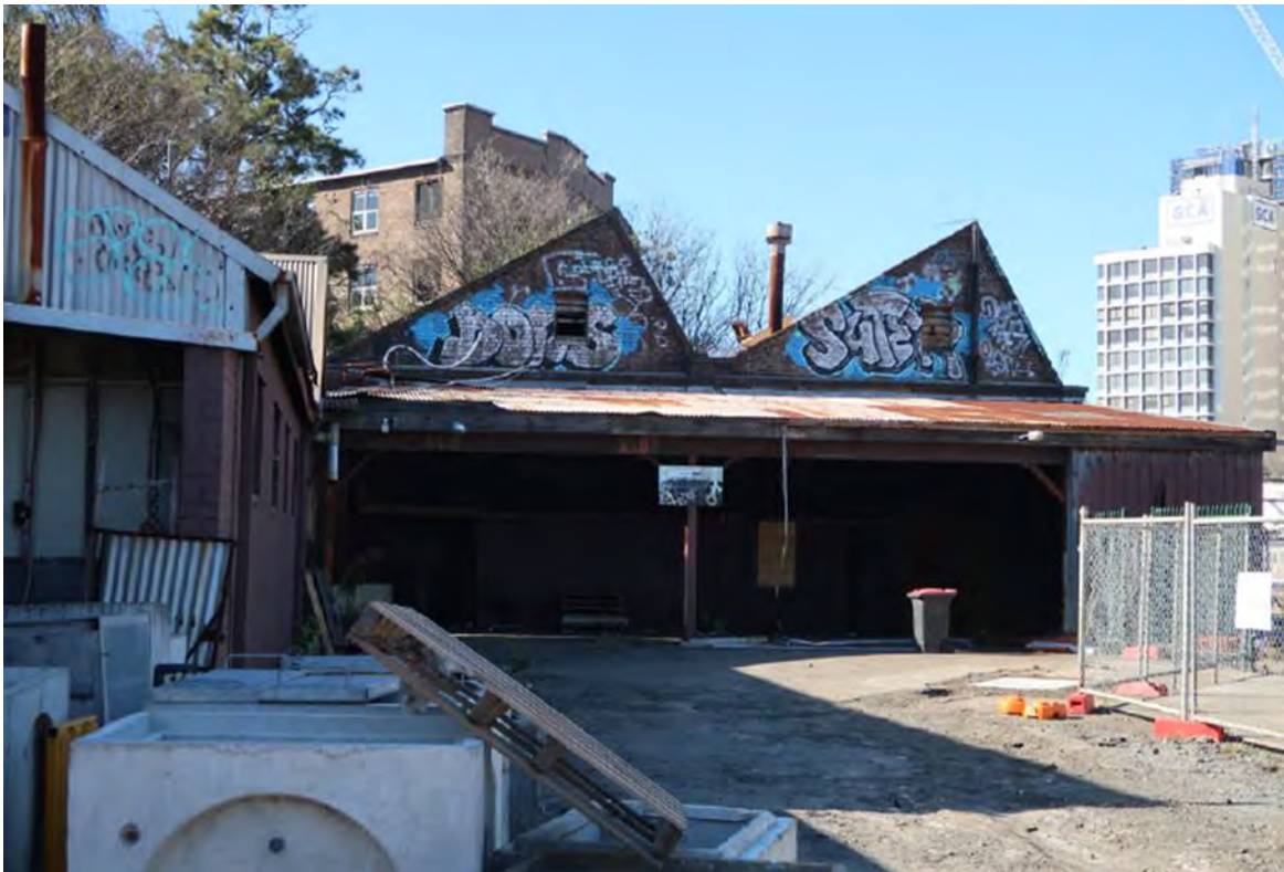
Figure 4.103: Western elevation of the Telecommunication Equipment Centre, later addition western awning extending from main building (Source: TZG Architects 2020)
