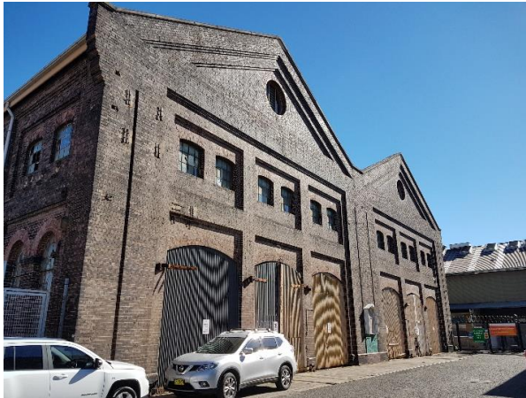
Picture 1 Eastern Elevation of LES
