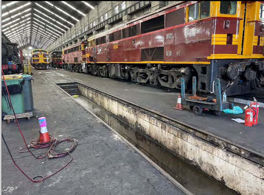
PHOTO 3: MAINTENANCE AND REPAIRS TRENCH WITH POOLING WASTE WATER
