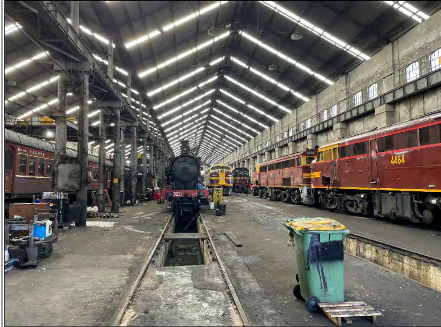
PHOTO 2: INTERNAL STRUCTURE OF LES WITH MAINTENANCE TRENCH VISIBLE, FACING EAST
