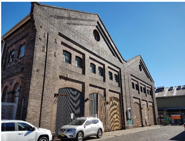
Picture 1 Eastern Elevation of LES
