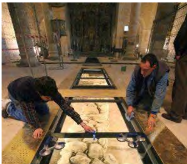
Figures 4.12 Examples of archaeology view reinforced glass floors with lighting
