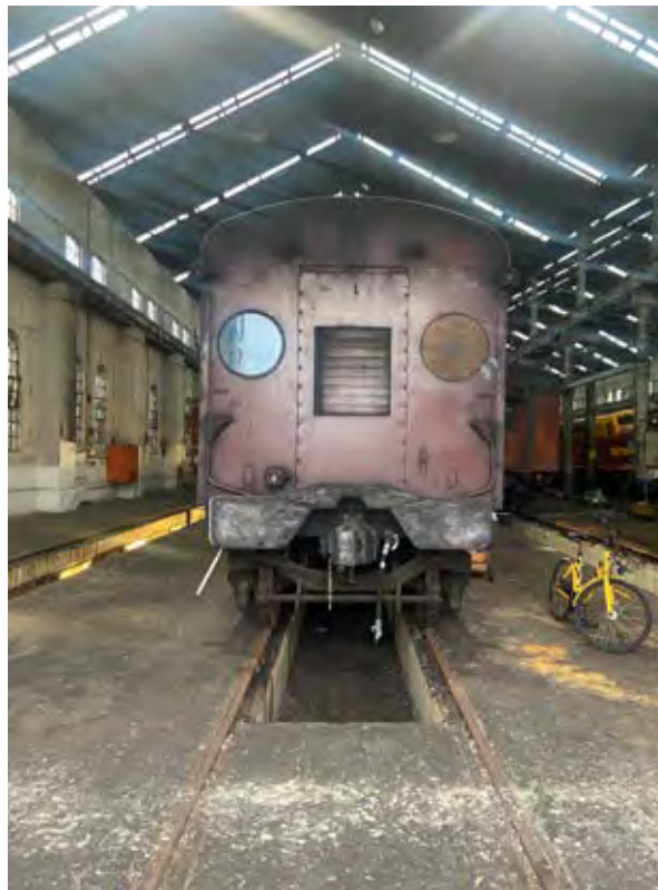
Figures 4.11 Examples of Inspection pits, Large Erecting Shop
