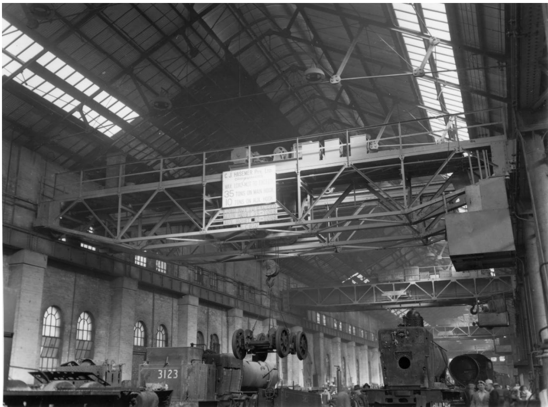
Figure 3.22: One of the Large Erecting Shop's massive overhead cranes carries an engine's bogie, consisting of its wheelset and axles (Source: State Rail Authority Archives, State Archives NSW, 15941, NID 601/24)
