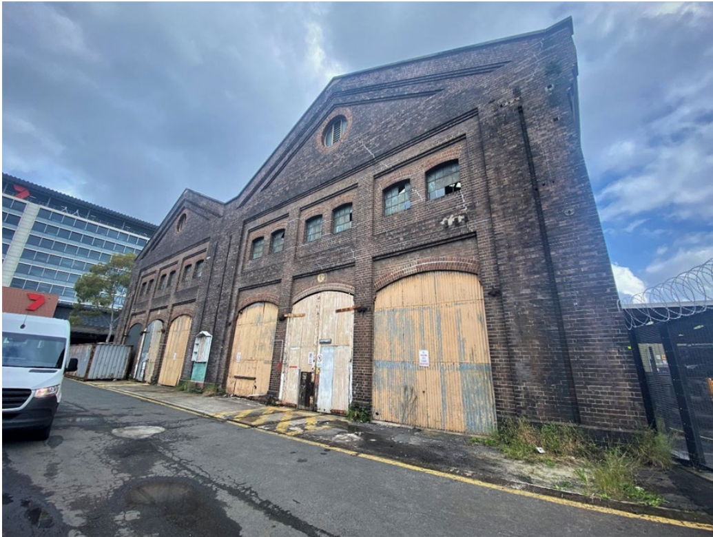
Figure 4.12: Eastern façade of the LES showing the corrugated iron clad doors and infills. Source: Curio Projects, 2022
