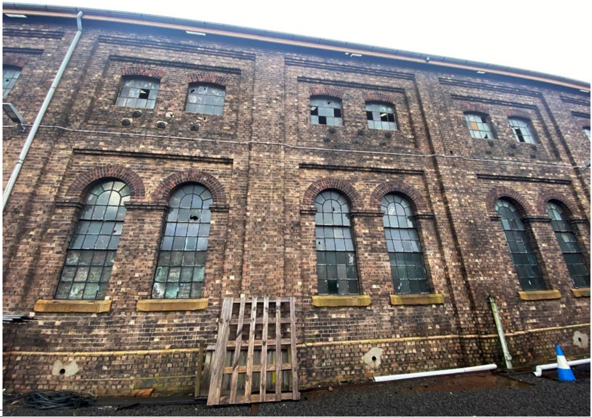
Figure 4.11: LES building facade configuration showing brickwork, engaged columns, upper and lower window example. Source: Curio Projects, 2022
