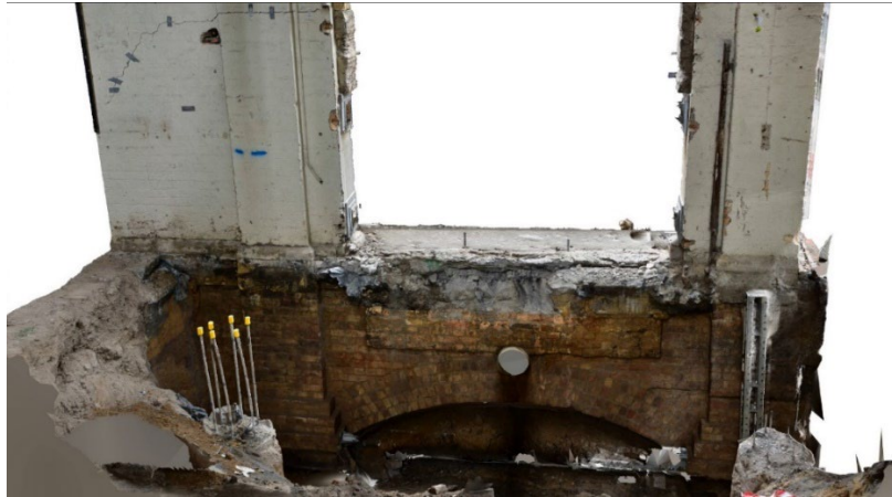
Figure 5.4: Photogrammetry model of Brick footings and arch of Locomotive Workshop uncovered and recorded during archaeological monitoring of construction works (Source: Curio 2019)
