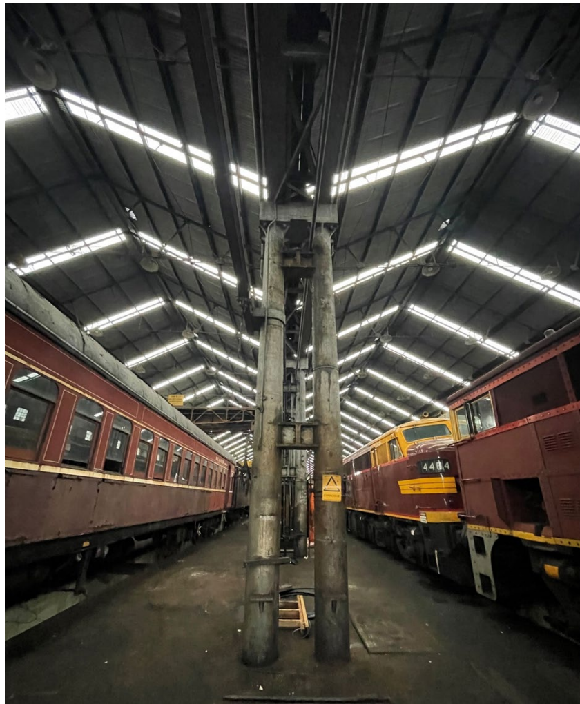
Figure 4.19: Cast Iron Columns Supporting the Roof Structure. Source: Curio Projects, 2022
