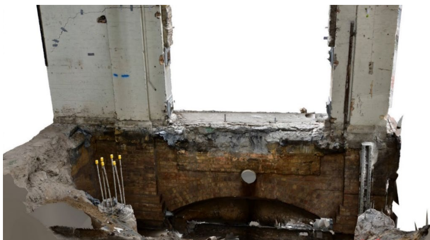
Figure 5.4: Photogrammetry model of brick footings and arch of Locomotive Workshop uncovered and recorded during archaeological monitoring of construction works. Source: Curio Projects, 2019.
