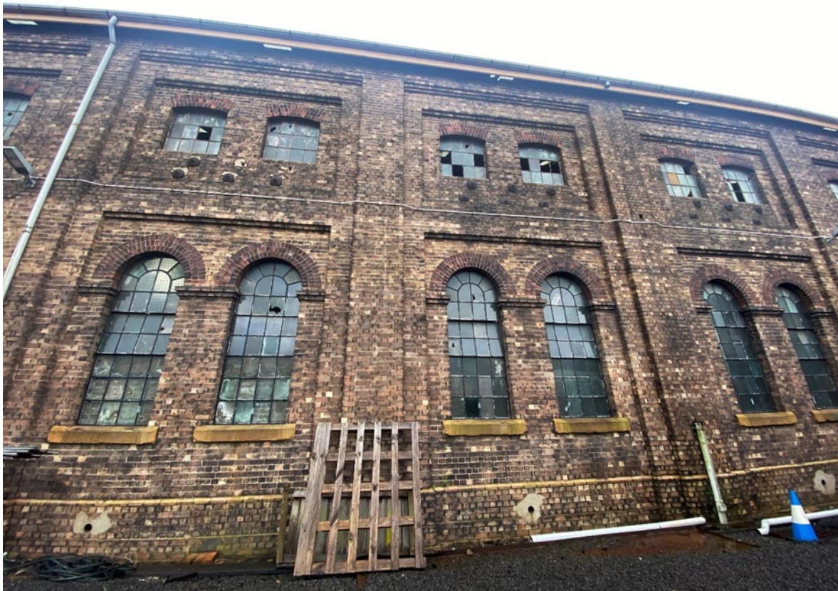
Figure 4.11: LES building facade configuration showing brickwork, engaged columns, and upper and lower window examples. Source: Curio Projects, 2022
