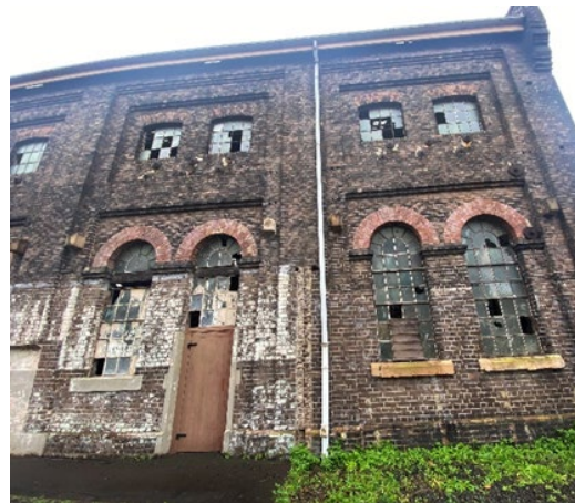
Figure 4.16: South wall single entry doors and modified window. Several glass panels of the existing windows are damaged and require replacement. Source: Curio Projects, 2022
