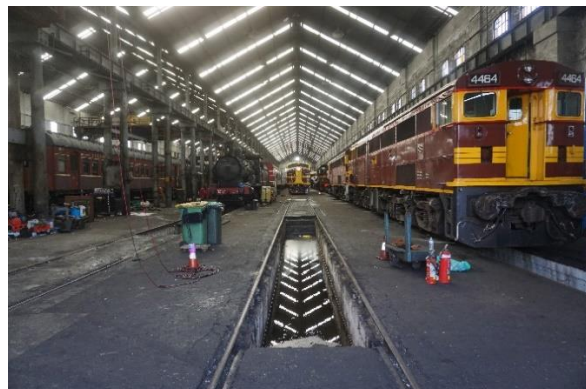
Figure 6.12: Internal view of the LES highlighting the pits located across the building's footprint (Source: Curio 2022)
