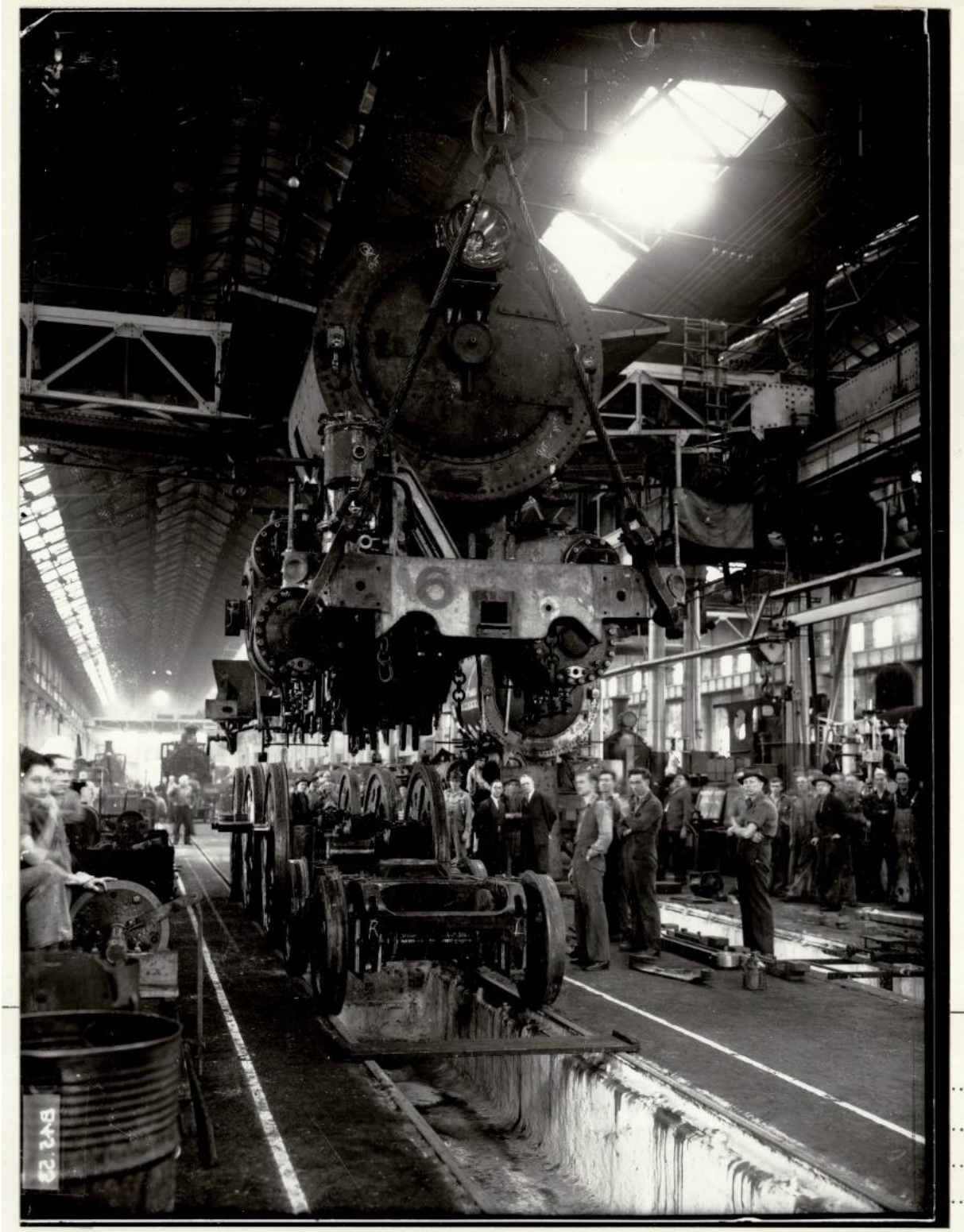
Figure 4.3: A steam locomotive engine is lifted off its wheelset and bogie by a crane in the LES. Note the access pit in between the tracks for working on the underside of the engine (Source: NSW State Archives)
