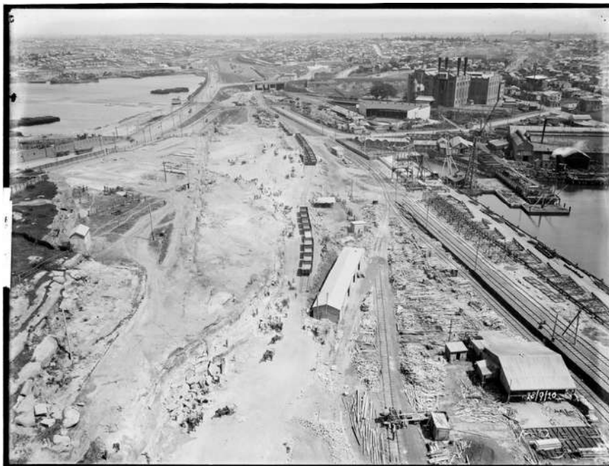
Figure 5.4.2: Quarrying at Glebe Island for Wheat Silos. White Bay completed to Stage 1 visible in the background together with the steel mill and locomotive shed. 14
