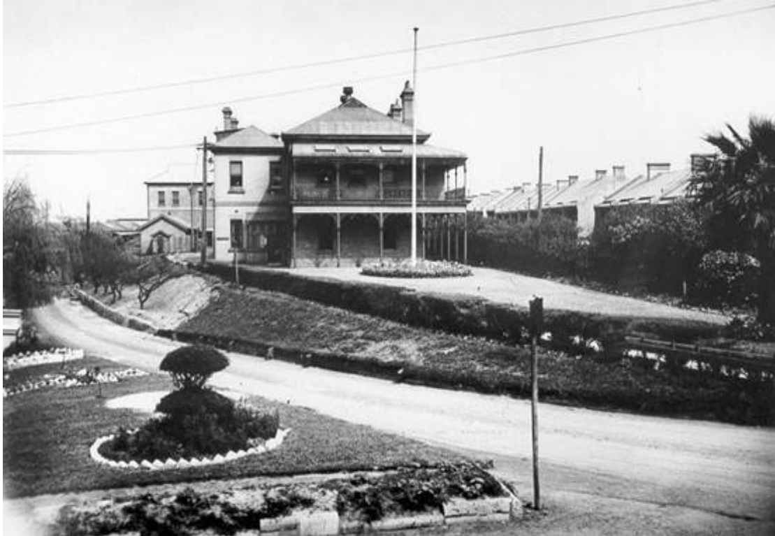
Figure 2.33 – Photo of the Chief Mechanical Engineers Office believed to be circa early 1920s. Although the trees that can be seen in this photo probably no longer exist, it is the authors opinion that the larger and currently remaining Canary Island Date Palms date to a period just after this photo, possibly around 1930 and the larger Camphor Laurels probably date to a period around 1940 to 1950 when these species were still commonly planted in public landscapes around Sydney (Source: Central to Eveleigh Facebook page and Caldis Cook - CMEO CMP, 1997)
