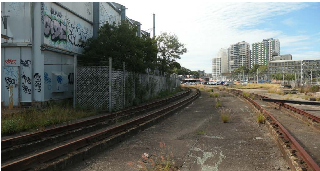
Figure 3.13 - Currently the site is a neglected and largely inaccessible industrial landscape with a variety of degraded landscapes and buildings. Although there is some 'green cover', the vast majority of this is simply weed and grass growth amongst the degrading and over the otherwise impermeable pavements. The existing 'canopy coverage' with the site itself is less than 7% (Photo: Arterra)
