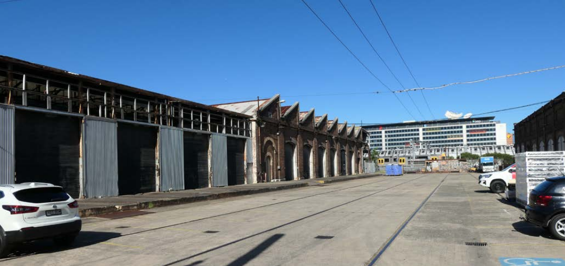
Figure 2.18 - Photo illustrating Paint Shop, Suburban Car Workshop, and Traverser. (Photo: Arterra).
