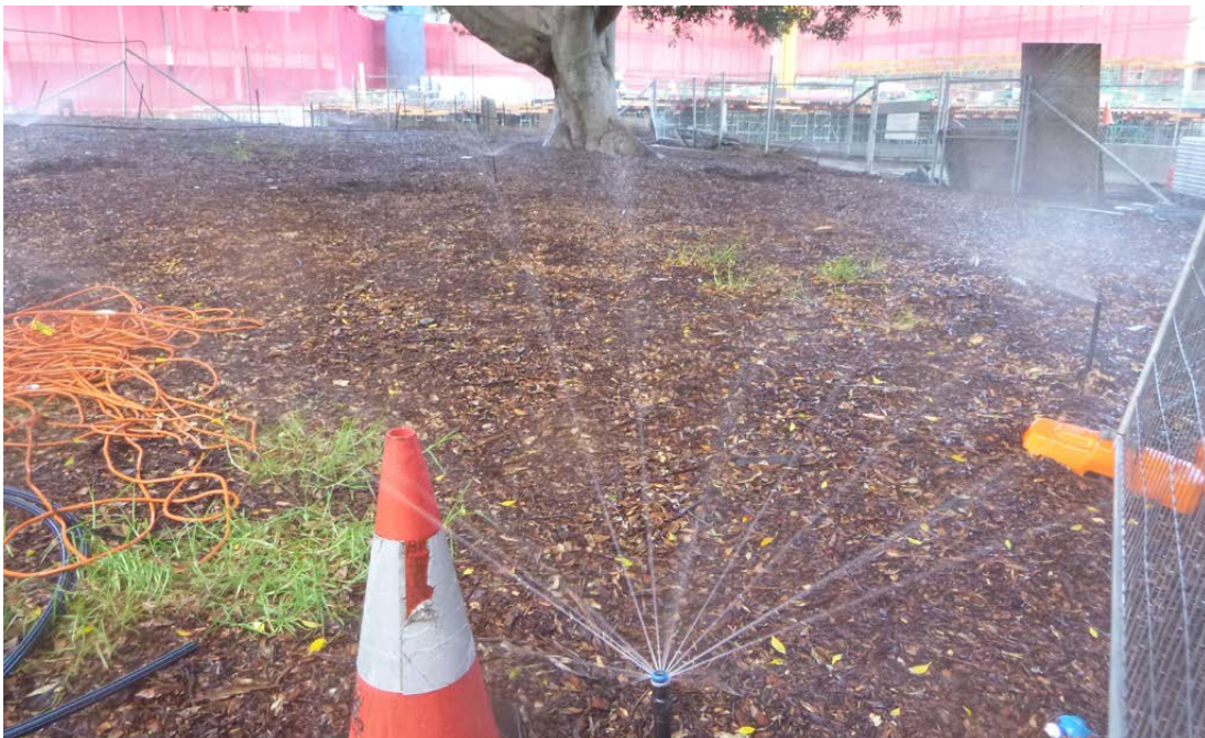
Figure 5.4– Example of a temporary irrigation system provided to trees during construction periods. This can be a very valuable way of ensuring tree health and vitality is maintained and also promote new fibrous root growth closer to the trees. (Photo: Arterra)
