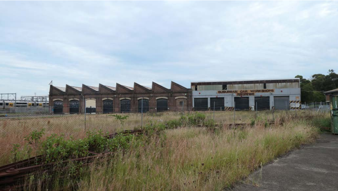
Figure 2.19 - Photo illustrating the fan of Tracks and the Paint Shop and Suburban Car Workshop illustrating that the majority of the site is historically devoid of trees and other green infrastructure. (Photo: Arterra).
