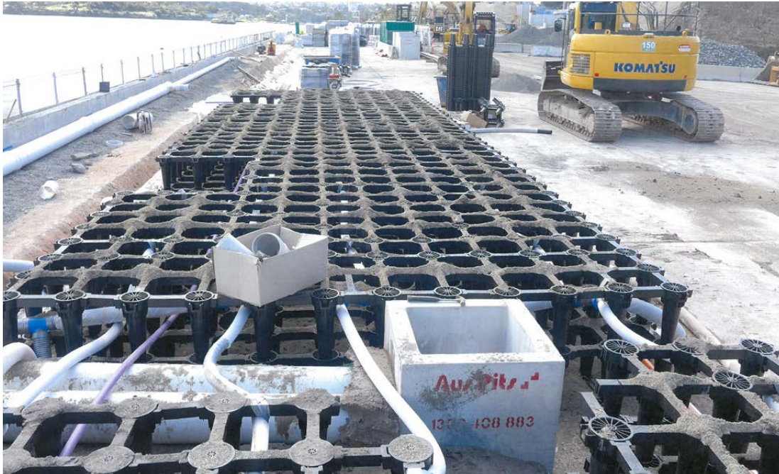
Figure 4.17—Numerous methods are now available of integrating trees and the necessary soil volumes within urban environments while still allowing pavements and roads to continue successfully above. The above illustrates the proprietary system Strata Vault by Citygreen being used at Barangaroo Sydney.
