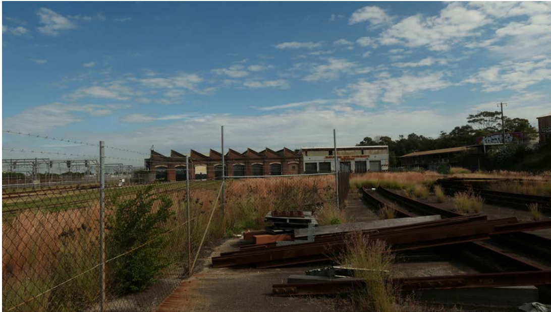
Figure 2.38 – Photo illustrating the extensive levelling for the railway development and the creation of the large workshops and other sheds. Most existing soils are anticipated to have been substantially altered and lost during this process and replanting will require extensive intervention and efforts to recreate suitable growing conditions for new trees. (Photo: Arterra)
