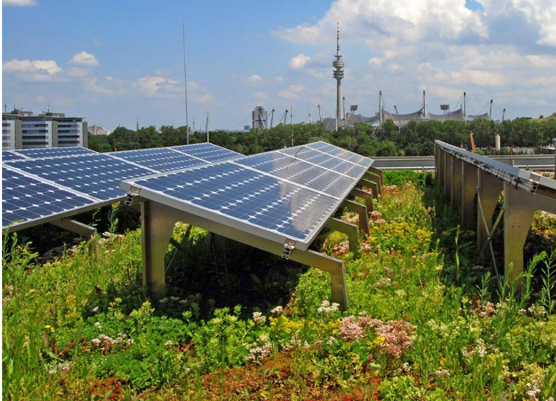
Figure 4.6 – Provision of green roofs and on-structure podium planting will be a vital component of the green infrastructure provision of the precinct. It can be combined with photovoltaic arrays and can greatly contribute to reduced urban heat and increased biodiversity and habitat values and connection to Country (Source: ZincoGreenRoofCo - Toronto [Pinterest])
