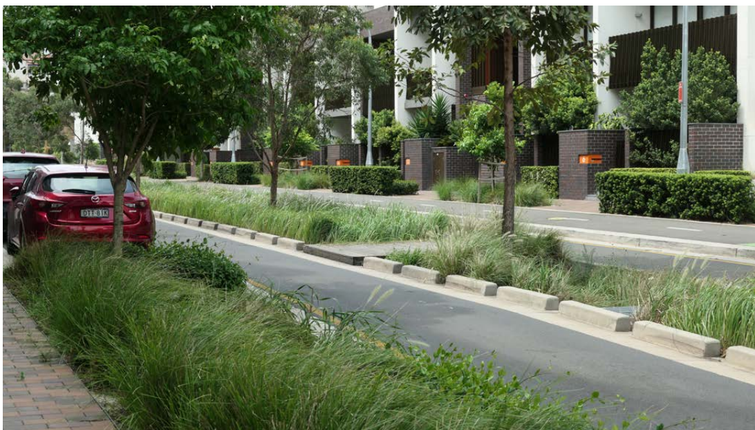
Figure 5.6– Example of a rain gardens, WSUD and tree planting at Harold Park redevelopment, Glebe, that would be equally applicable and expected at the Paint Shop Sub-Precinct. (Photo: Arterra)
