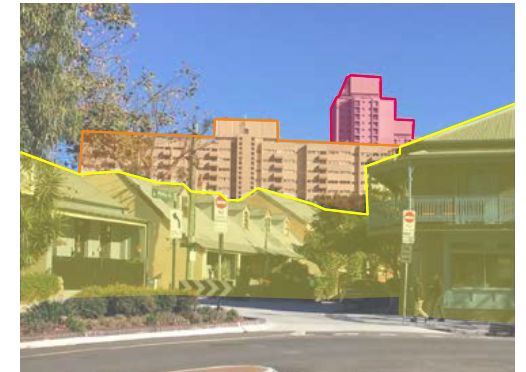
Fig.6.3.13 Redfern Estate HCA near Redfern Oval with Waterloo Estate beyond; view from Phillip Street
