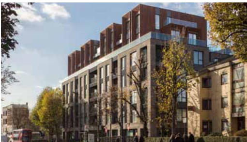
Fig. 6.2.24 Camden Courtyards, UK Source: Sheppard Robson, 2017
