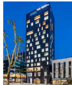
Fig. 6.2.27 The Book Company Headquarters, Source: N.E.E.D Architecture, 2017
