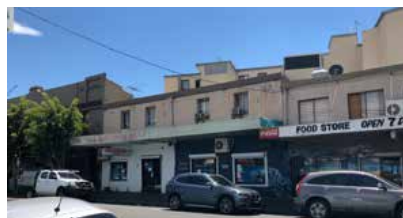
Fig. 5.2.5 Shops along Raglan Street
