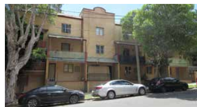
Fig. 5.4.6 Dwellings along Wellington Street
