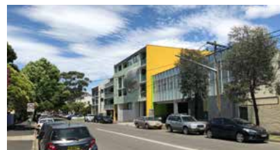
Fig. 5.3.3 View south along Cope Street
