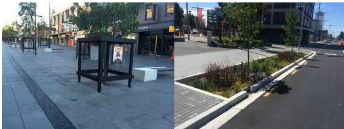
Figure 19 Examples of at-source WSUD in highly urban environments
