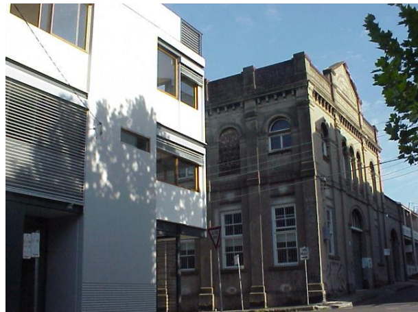
Picture 40 – View of Turner Street.
