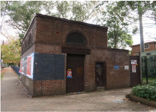
Picture 23 – Privately owned and locally heritage listed sub-station fronting McEvoy Street (address being 336 George Street)
