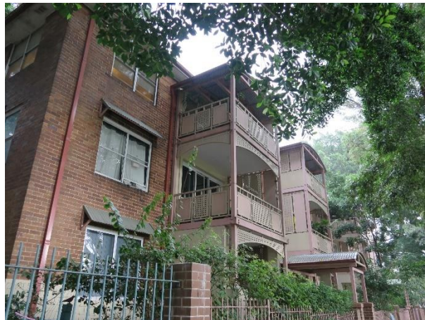
Picture 4 – Northern elevation of one of three of the first blocks, as viewed from Raglan Street
