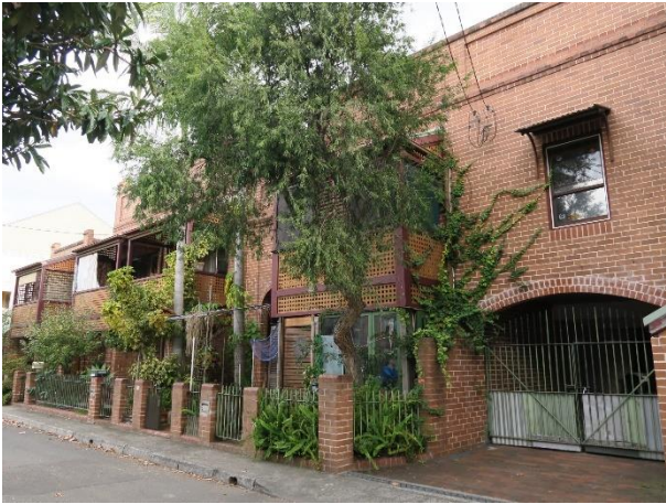
Picture 15 – Referential infill development at 97-109 Cooper Street
