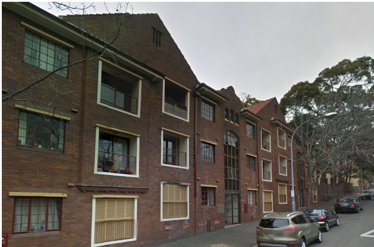
Source: Google Street View, July 2015
