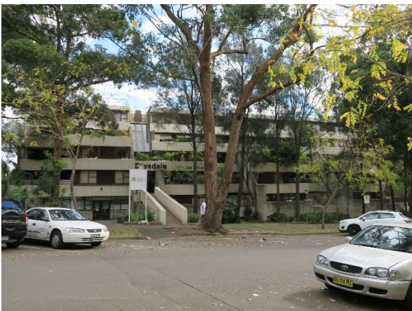
Picture 11 – Principal elevation of ‘Drysdale’ from Pitt Street
