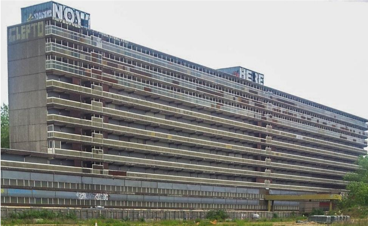
Figure 102 – View of The Heygate Estate prior to complete demolition works, c. 2013-2014
