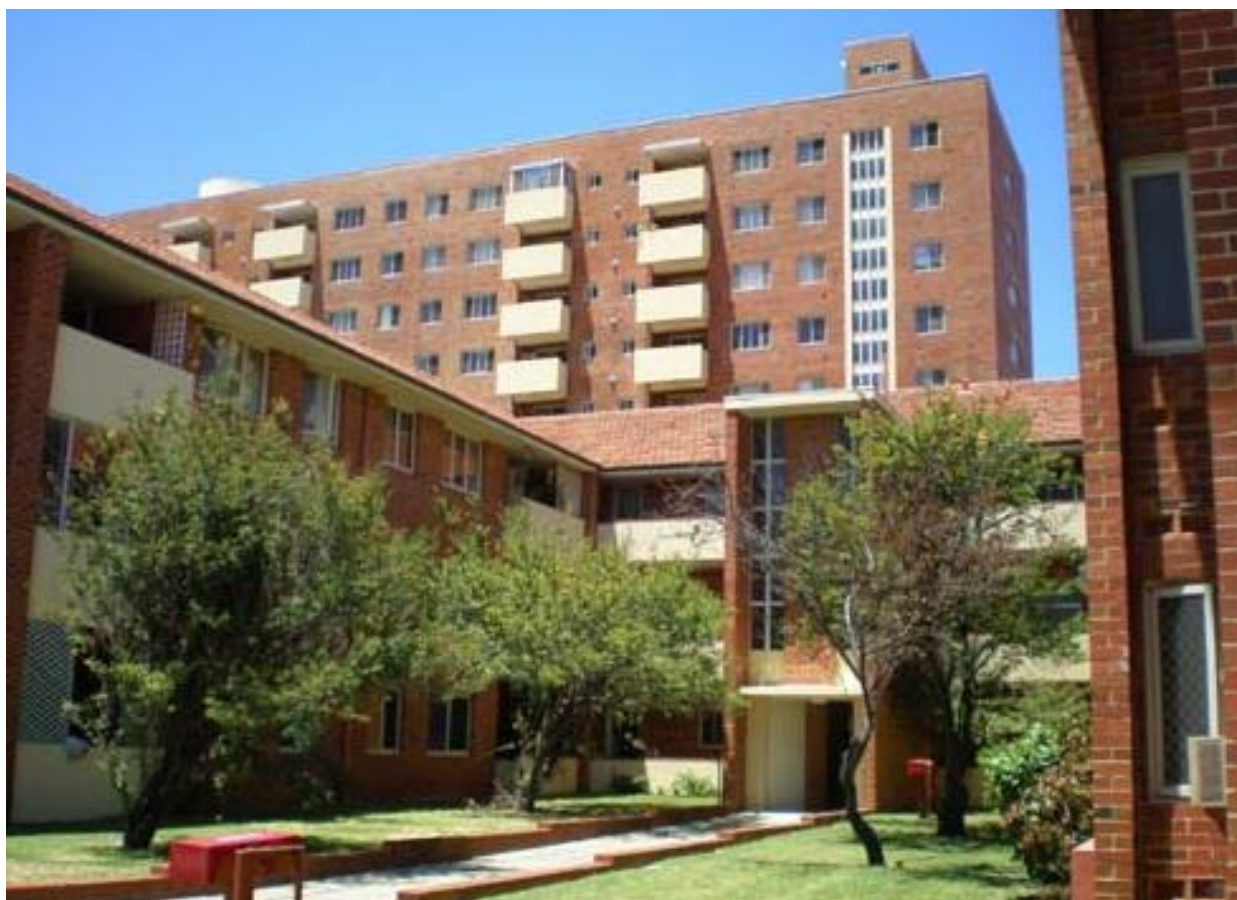
Figure 124 – The Wandana Apartment Block, 2008
