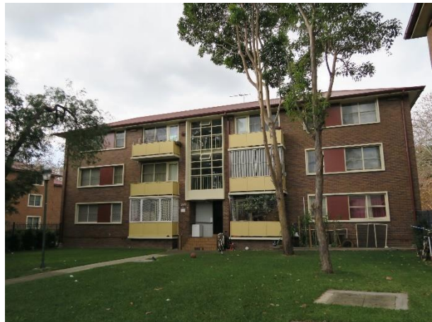
Picture 8 – 249 Cope Street, facing east
