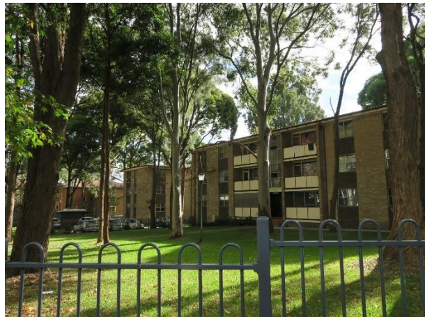
Picture 6 – The southern elevation of the walk-up flat building at 339-341 George Street, taking from McEvoy Street
