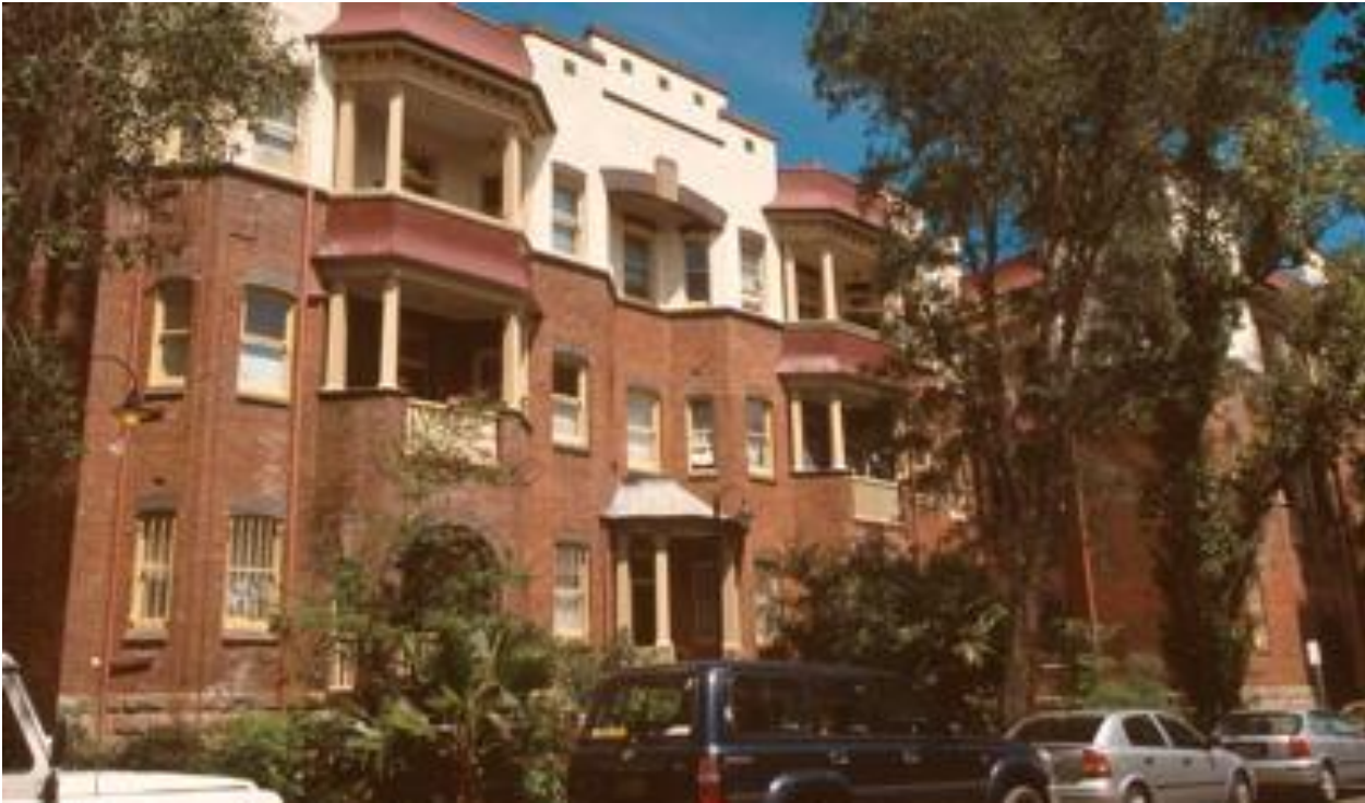
Figure 63 – View of the Strickland Building, date unknown
