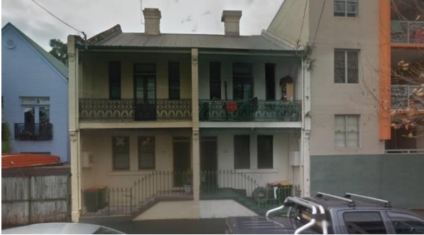
Figure 23 – View of terrace pair from Cope Street.
