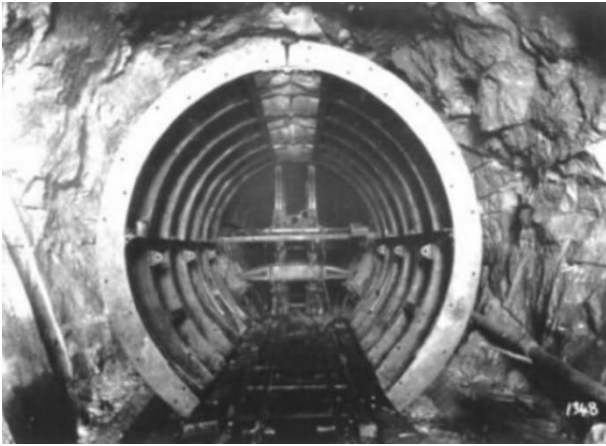
Picture 33 – Indicative view of the Pressure Tunnel
