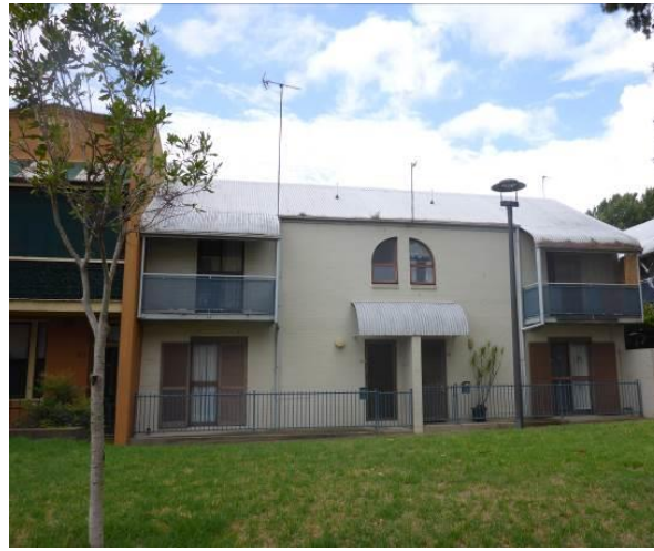
Picture 78 – Terraces along Forbes Street, featuring referential arched windows and overall form in a contemporary style
