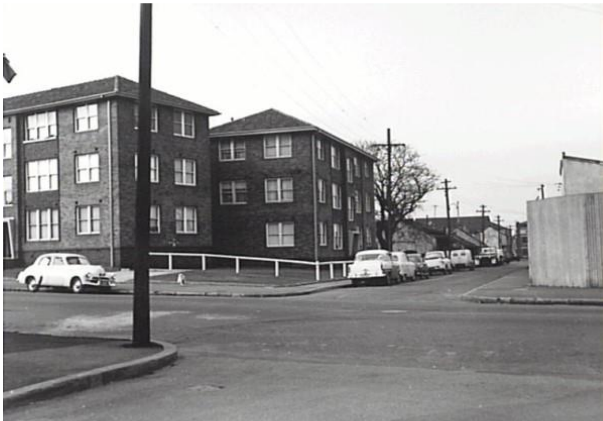
Figure 43 - The completed Blocks 1 and 3 on the corner of Raglan and Cooper Streets, Waterloo in 1961. Note the houses and sheds fronting Cooper Street in the distance that are yet to be demolished
