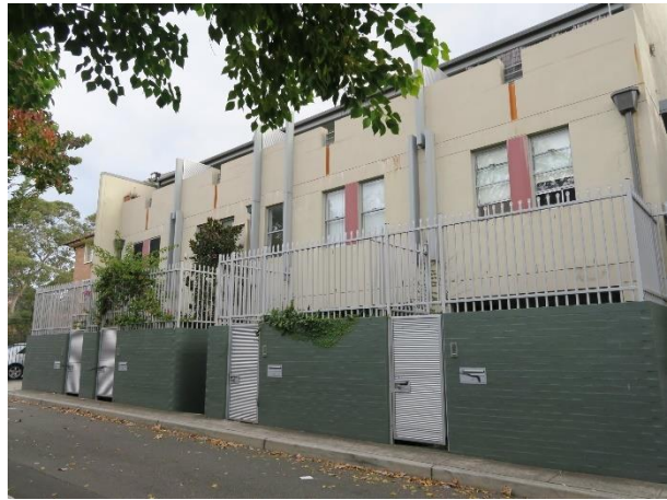
Picture 22 – Rear elevation of privately owned land at 233 Cope Street
