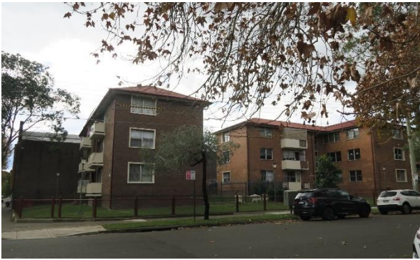
Picture 9 – Typical walk-up buildings at 6-8 John Avenue
