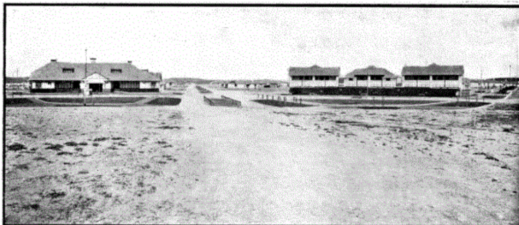
19] View of Suburb down Cook Avenue, from Entrance.
