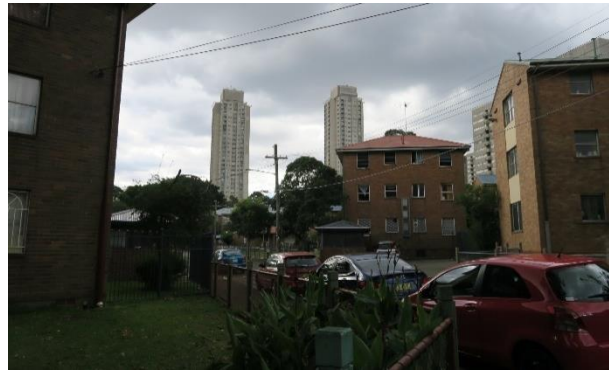
Picture 10 – Typical walk-up buildings facing north along Cooper Street, with Matavai and Turanga visible in the background
