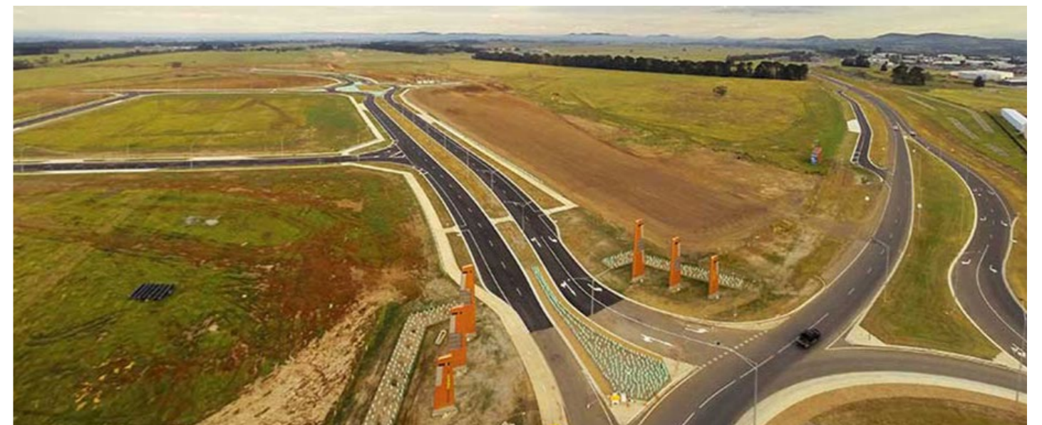
Figure 166. Aerial Photo of Ballarat West Precinct
