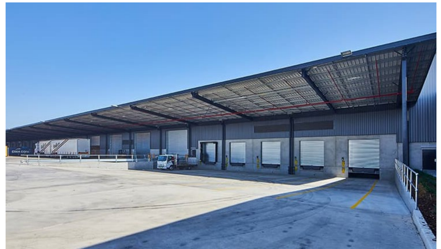
Figure 170. Photograph of exemplar warehouse in the Calibre Warehouse Estates
