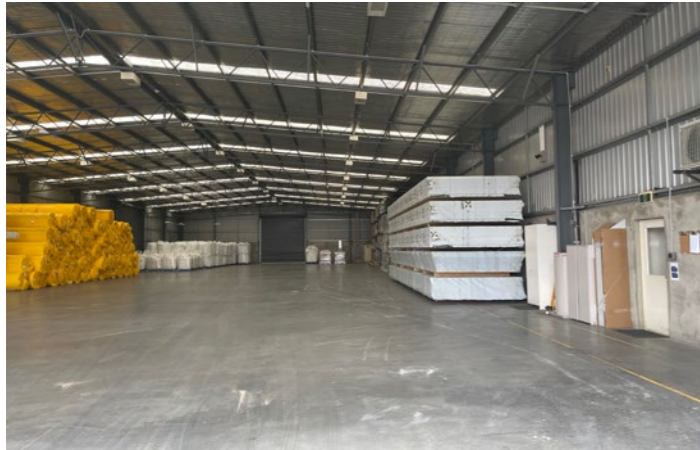
Figure 60. Storage facility adjacent the Rail Hub
