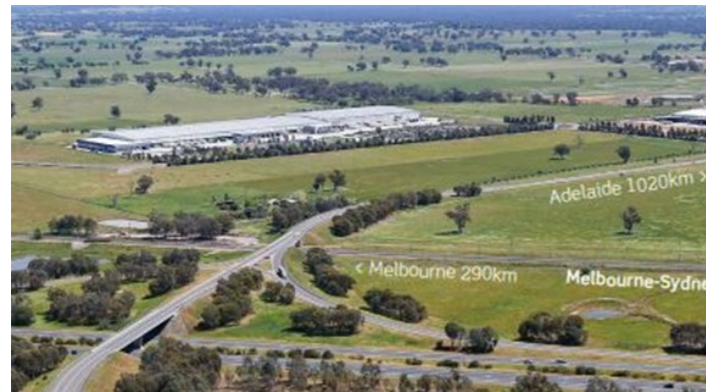
Figure 176. Aerial photo of Logic Precinct
