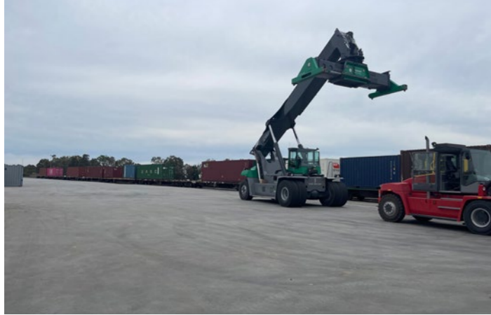
Figure 59. Ettamogah Rail Hub in action
