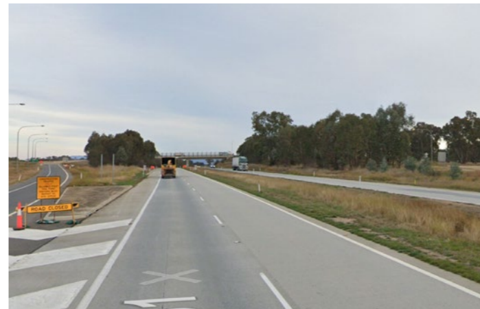
Figure 62. Waggga Road off ramp along the Hume Highway
