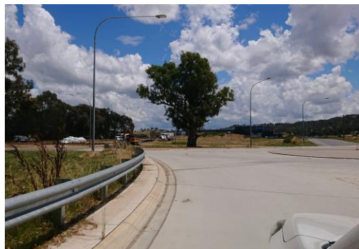
Figure 3-9 | A view looking west entrance to the Nexus industrial hub
