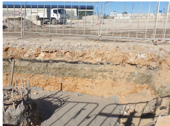
Figure 13: Excavated pit showing layers of fill
