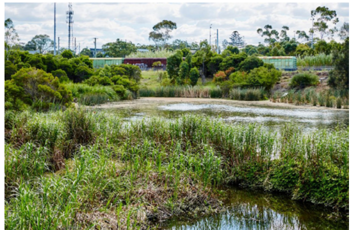
Figure 60: Constructed wetlands are good at removing sediments and heavy metals. (Source: Sydney Water)
