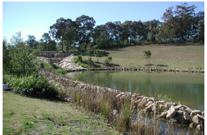
Figure 59: Sediment basins are designed to slow water down so sediments can settle. (Source: Sydney Water)
