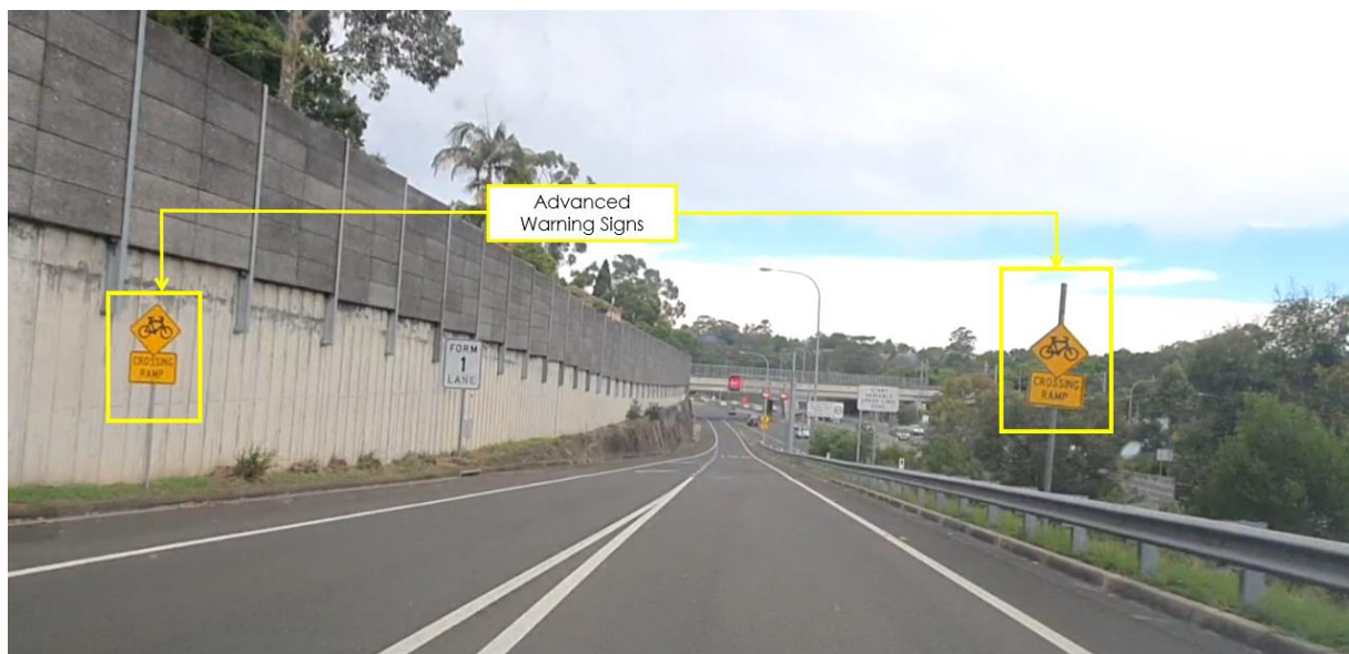
Figure 3: Existing Cycle Crossing Warning Signs
