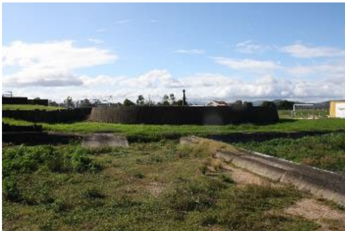
Photograph 8.35 Casino Sewerage Treatment Plant within Inspection Area 4 (ERM 2022)
