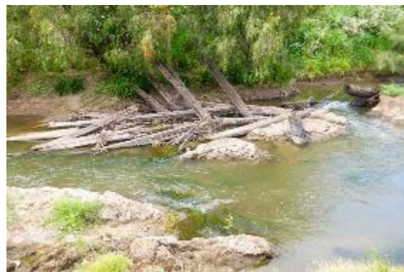
Photograph 10.11 Remnant wharf structure, possibly Grime's Wharf (2018) (Clarence Heritage, 2019: 13).
