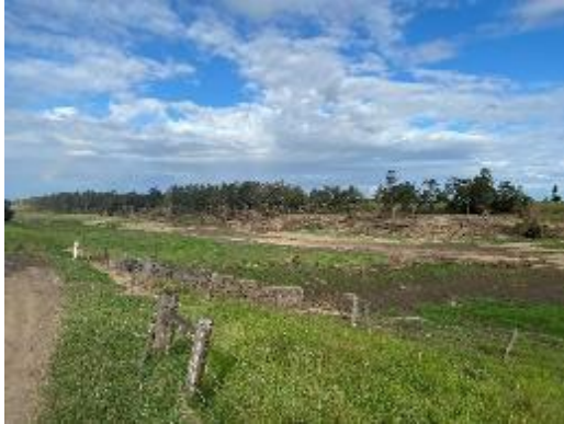
Photograph 8.36 Significant erosion visible on the southern bank of the Richmond River (ERM 2022)
