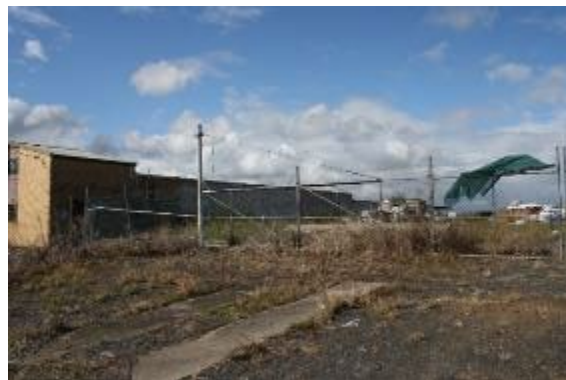
Photograph 8.26: Industrial estate of SU7 (ERM 2022)
