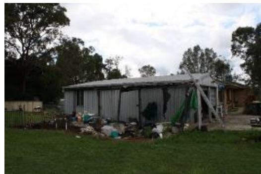
Photograph 8.16: Modified area along western boundary of SU4 (ERM 2022)
