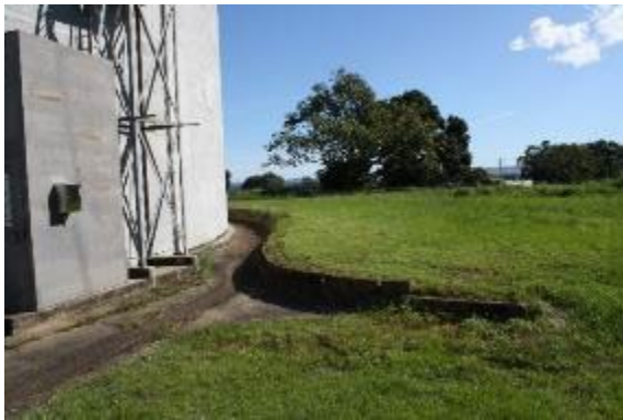
Photograph 8.23: Large water tanks located on the crest on the hills within SU6 (ERM 2022)
