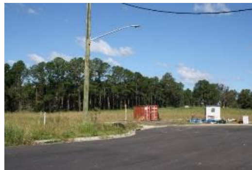
Photograph 8.18: Newly constructed road of SU5 (ERM 2022)
