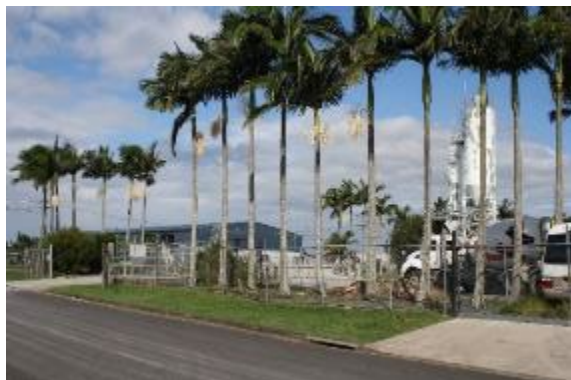
Photograph 8.25: Industrial estate of SU7 (ERM 2022)
