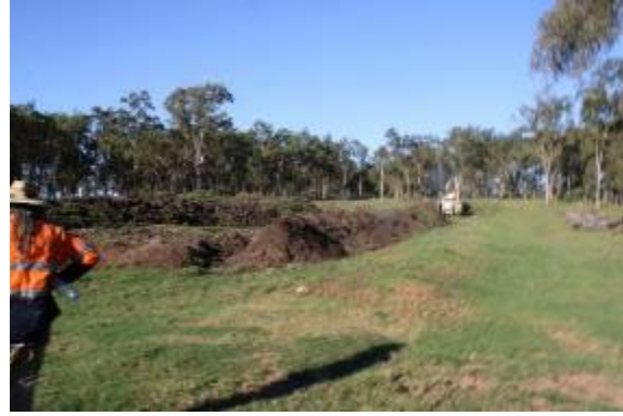
Photograph 8.6: Severe ground disturbance in SU2 (ERM 2022)
