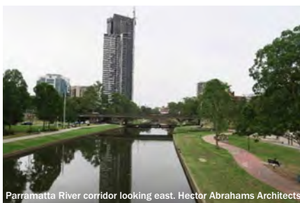
Parramatta River corridor looking east. Hector Abrahams Architects
