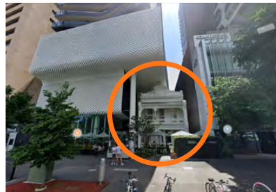
Fifty Albert: 42-50 Albert Road, Melbourne. Extent Heritage
