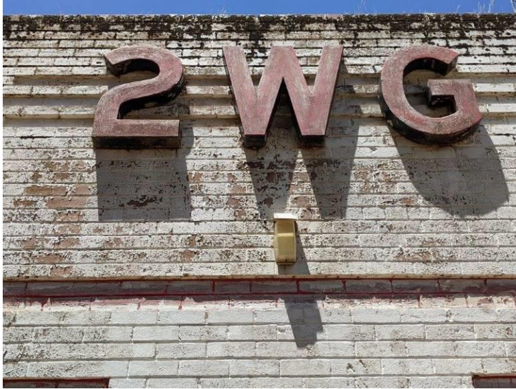
Photograph 2 Detail view of the steel letters on the front elevation also noting the recessed brick banding detail, typical of the period and style.
