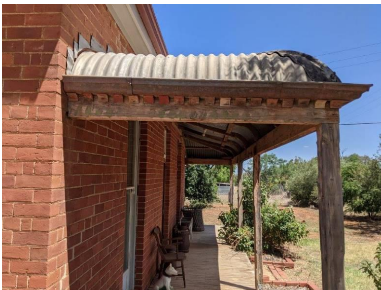
Photograph 11 Postal receiving office (former), Detail view of the North Elevation, noting the timber dentil brackets to the gutter on the bull nose verandah
