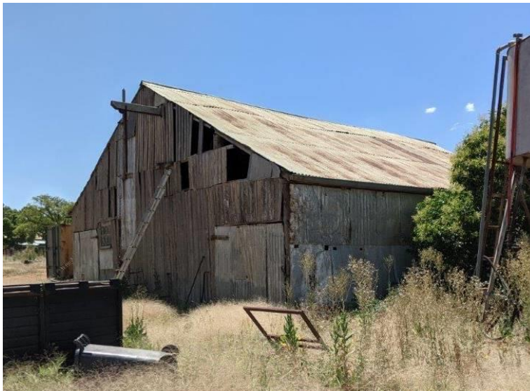
Photograph 4 View of the West elevation, noting the remnant timber boards in a paling layout on this gable side and the protruding timber hoisting beam. The galvanised iron short roofing sheets appear original.
