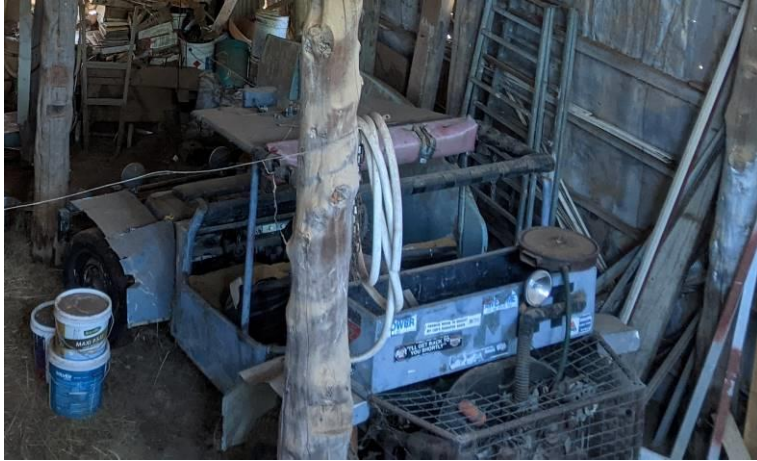
Photograph 16 Close view of the two posts where halving cuts denote where rails were fixed, possibly indicating the use of the bays between the posts for stabling. A closer inspection with internal access may reveal further details.
