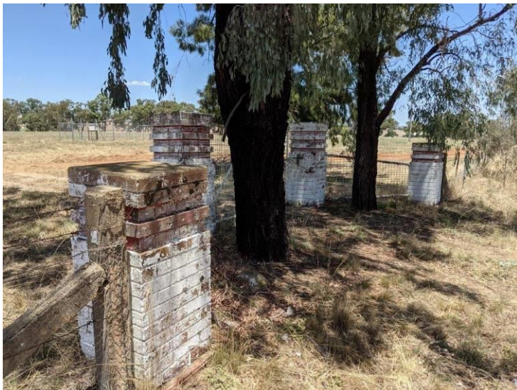
Photograph 14 Oblique view of the entrance, looking south-west to show the arrangement of the four piers with their detailing and the two angled sides and noting the original pink brick colour where the paint has eroded.
