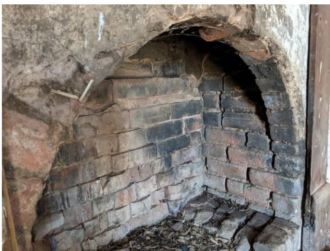
Photo 14 Detail view of the fireplace with arch construction detail
