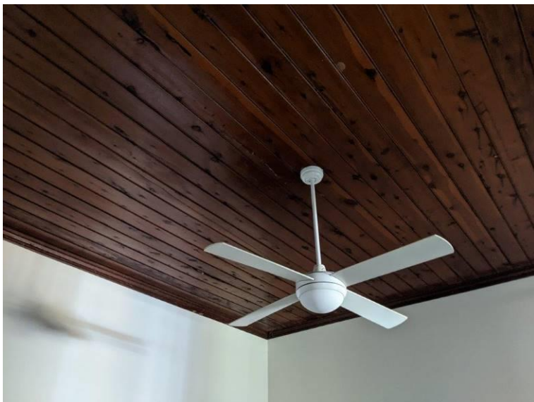
Photograph 17 View of the original timber boarded ceiling in the rear north-east room.
