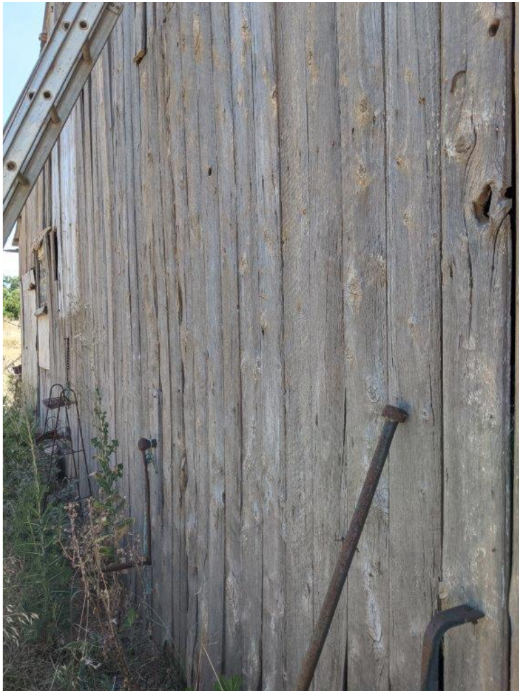
Photograph 7 Close view of the square cut paling boards on the West elevation, noting the remnant off-white or whitewash external finish.
