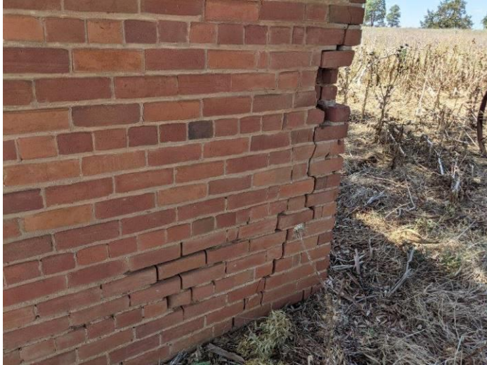
Photo 26 View of the south western subsided corner and damaged brickwork.
