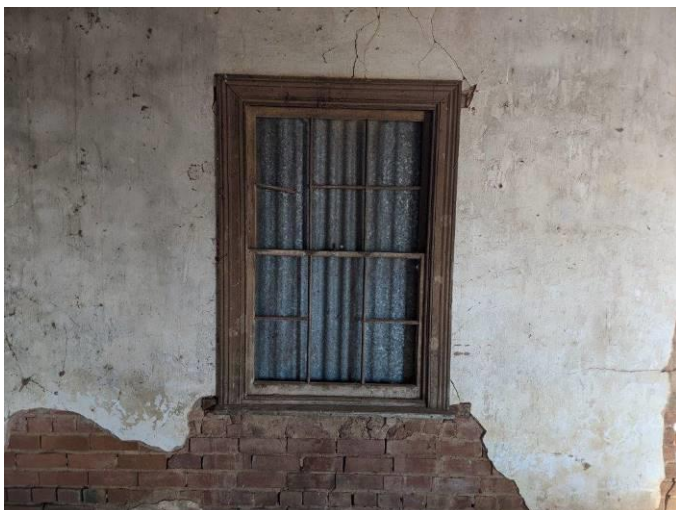
Photo 19 Remnant front double hung sliding sash window and surround and remnant lime plaster with lime wash.
