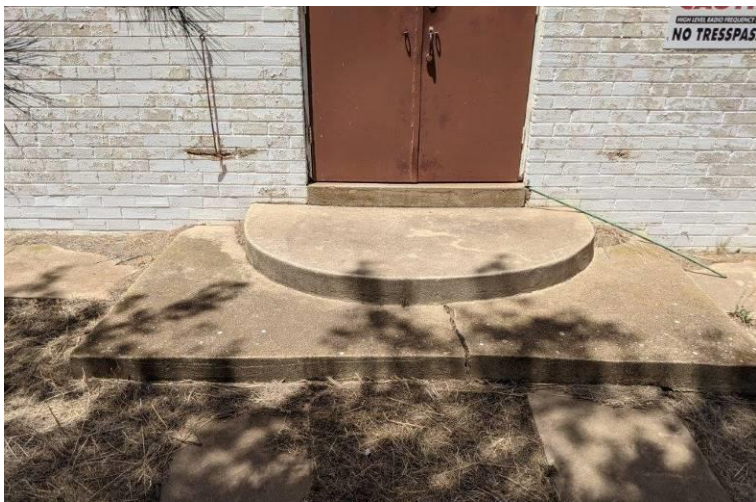
Photograph 11 A detail view of the entry with two concrete strips ending at the rectangular podium step and the semi-circular pad and double steel doors with hold-open strap and wear mark on the wall.
