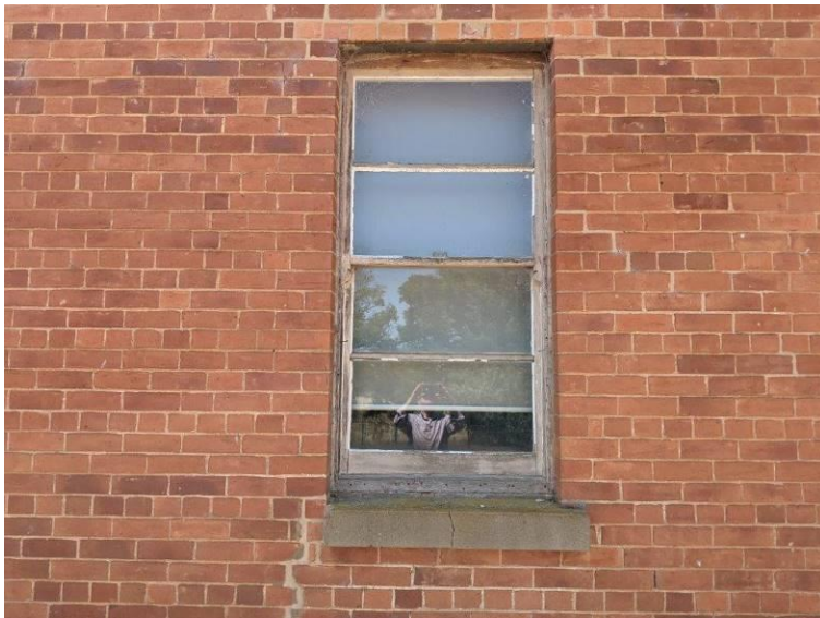
Photograph 6 Post Office (former), Detail view of the timber double hung sliding sash window circa Inter-war period, conserved brickwork, rendered sill, replaced lintel, the South Elevation
