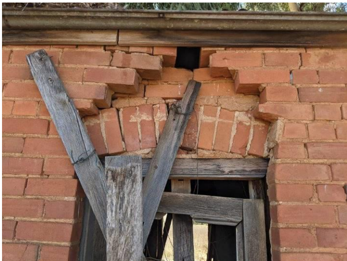
Photo 27 Detail view of the damaged rear door and missing brickwork.
