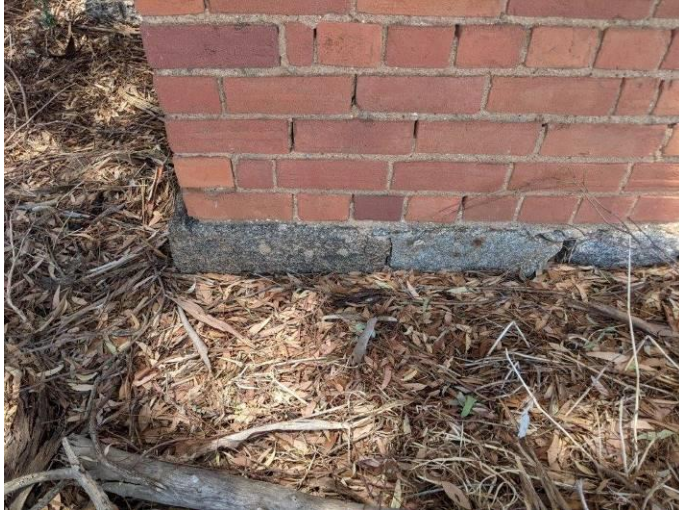
Photo 9 Detail view of the granite block foundation to the brick walls
