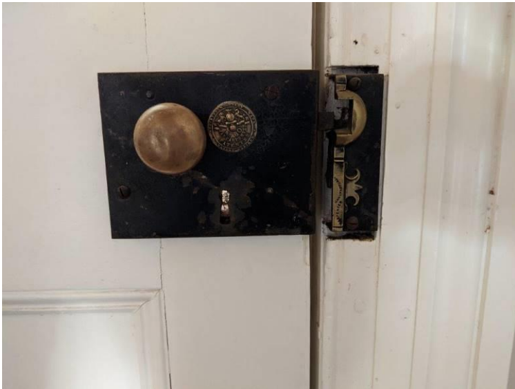
Photograph 20 Detail of the original rimlock hardware to the front door
