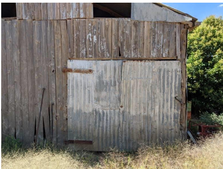
Photograph 5 A detail view of the galvanised iron sheet clad door at the south west corner of the West elevation, noting the early steel hinges and boards fixed in paling manner.
