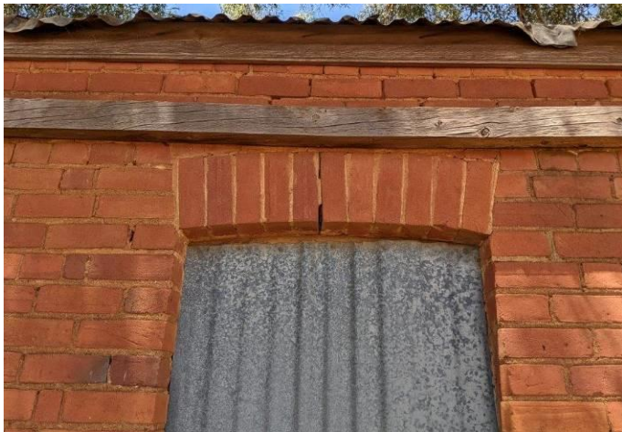
Photo 7 Detail view of the former front verandah wall plate and rubbed brick lintel to the window.
