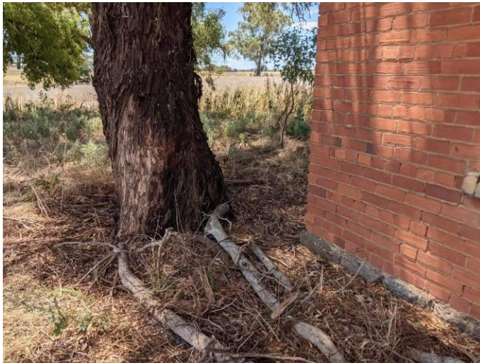
Photo 10 Detail view of the North west corner and proximity of the large eucalypt causing root damage to the foundation and walls
