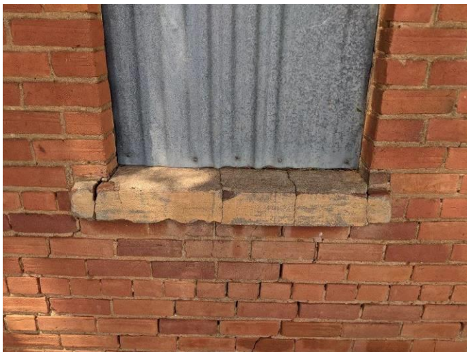
Photo 8 Detail view of the rendered brick sill to the window – one of two.
