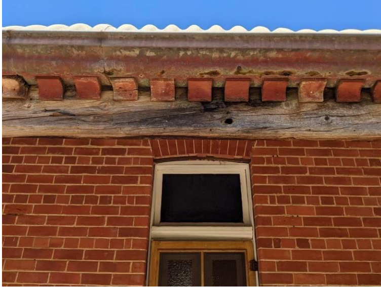
Photograph 14 Detail of the front elevation showing the timber detailing to the verandah beam, fanlight, lintel and front door.
