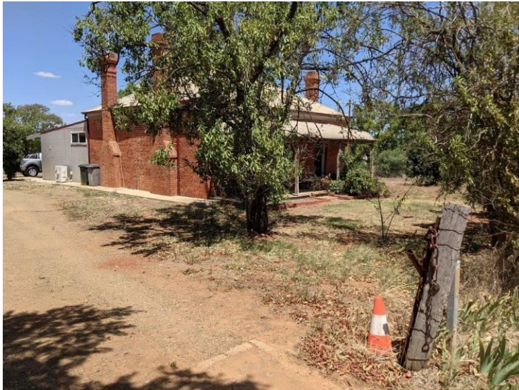
Photograph 15 General view of the frontage from the entry gate showing the North elevation with verandah and east elevation with brick chimneys and then the later refurbished rear skillion roofed extension.
