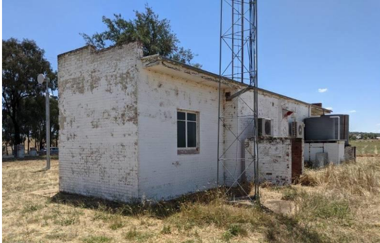
Photograph 4 View of the South and East elevations noting the expressed skillion roof and guttering.
