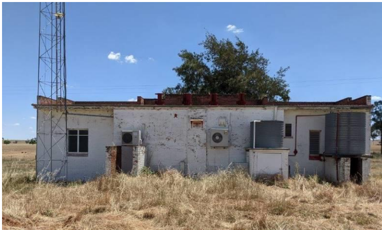
Photograph 5 The East Elevation, noting the brick tank stands, roof ventilators and original windows. Redundant elements which are not original may be removed and the character and integrity reinstated
