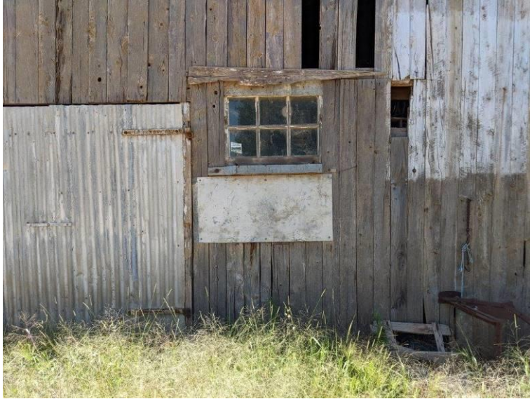
Photograph 8 Close view of the central portion of the West elevation, noting the random character of the elements and the re-used timber window patched into the wall.
