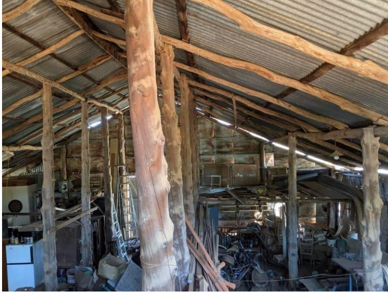
Photograph 14 View from the upper opening in the western wall to illustrate the original timber post and pole framing (undressed) while the purlins or battens are square cut.
