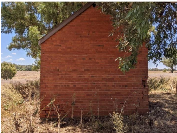
Photo 25 View of the South Elevation with settlement and root damage.
