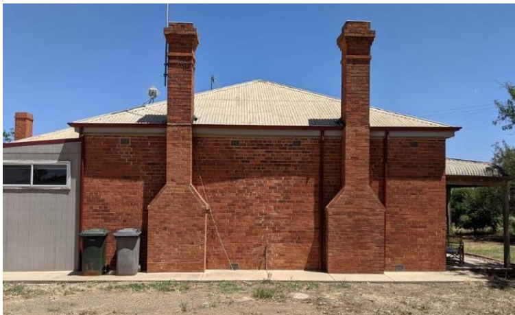
Photograph 10 Postal receiving office (former), View of the North Elevation, noting the brick chimneys, boxed eave, conserved brickwork, perimeter stabilising concrete path and modified rear skillion roofed element.
