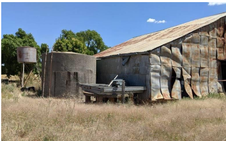
Photograph 2 View of the South elevation, noting the sheets in detail on the East side which appear to be flattened steel drums.
