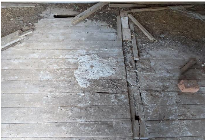
Photo 11 Detail view of the flooring and removed central partition wall
