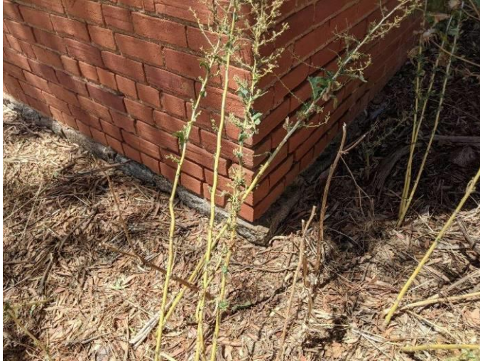
Photo 23 The rare full granite foundation and rising salt damp to the lower 600mm of brickwork
