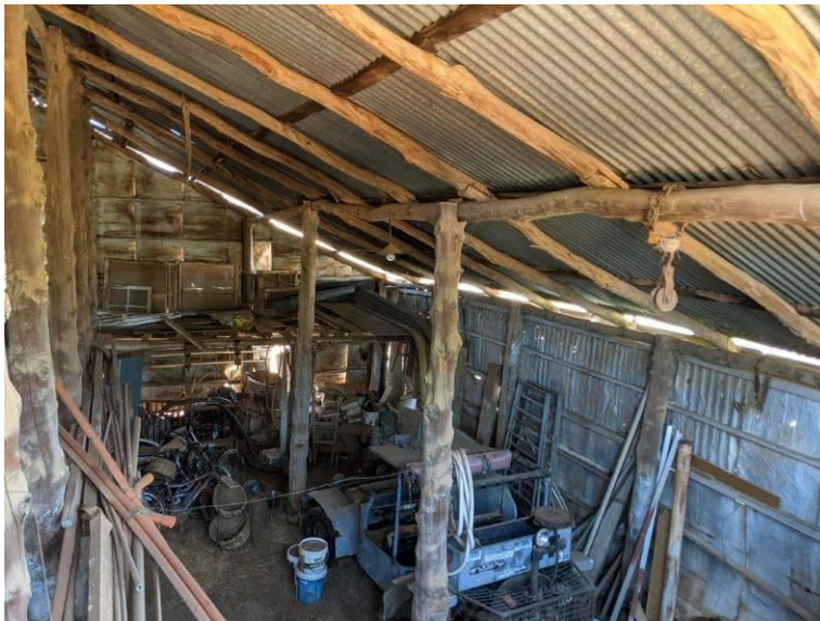
Photograph 15 View from the upper opening in the West elevation, looking towards the southern wall where the sheeting is fixed to square cut rails.
