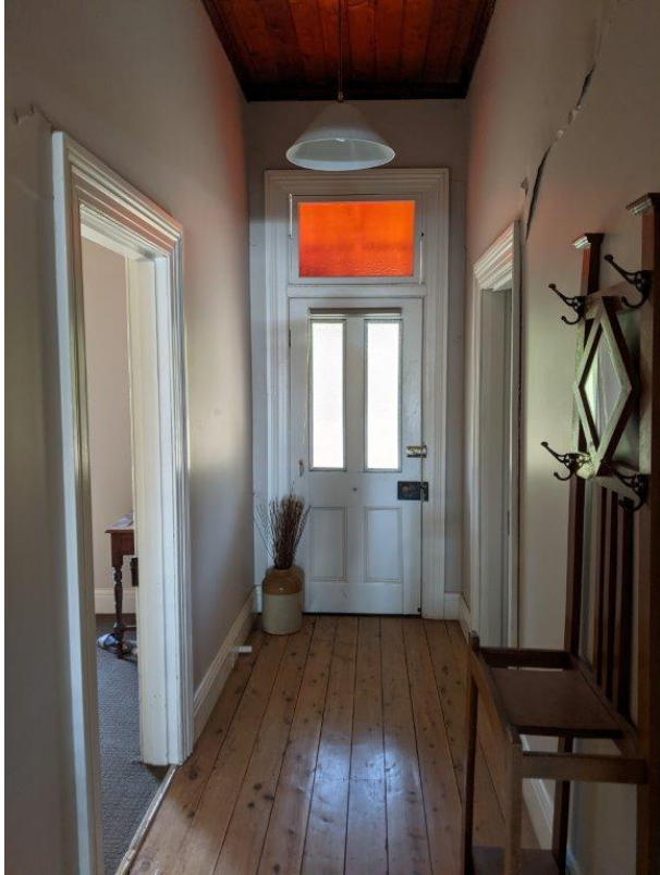
Photograph 18 Close view of the front passage noting the joinery, front door with fanlight and timber boarded ceiling. Walls show evidence of subsidence cracking.
