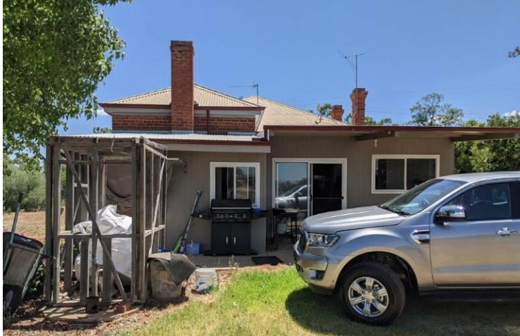
Photograph 9 Postal receiving office (former), View of the rear East Elevation, noting protruding room, hipped galvanised iron short sheet roofing, brick chimneys and modified rear skillion roofed elements.
