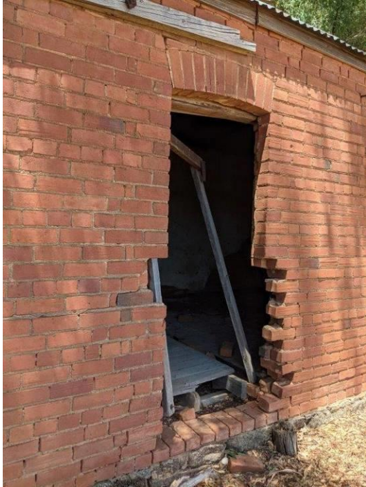
Photo 4 Detail view of the front door in the front West Elevation and wall plate indicating a verandah
