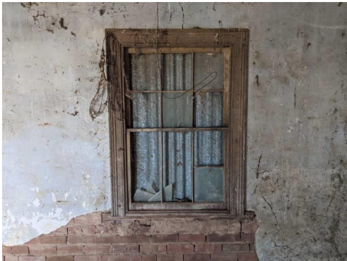
Photo 21 Remnant front elevation timber double hung sliding sash window and internal plaster. The window joinery is of a very high standard with excellent detailing.
