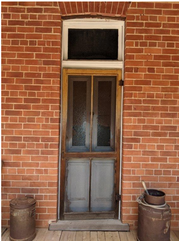
Photograph 13 Note the bond pattern. This is described as a Common bond with full headers every fourth course and three courses of full stretchers. The lime mortar joints are flush
