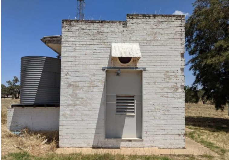
Photograph 7 View of the North Elevation with modified – increased opening and infill
