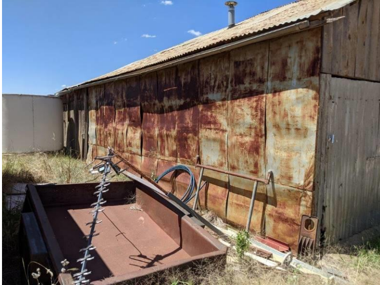
Photograph 10 View of the North elevation where the exterior is clad in similar steel sheet from flattened drums and the standard galvanised iron quad guttering.
