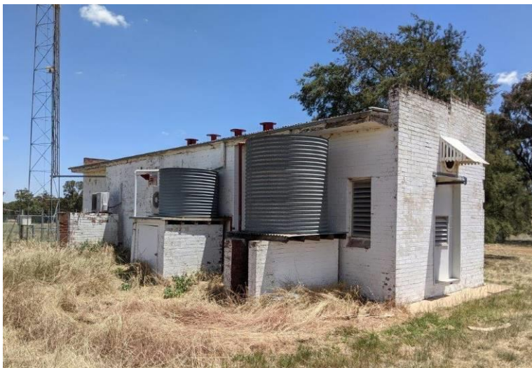
Photograph 6 View of the East and North Elevations, noting the returning parapet on the northern side wall and the later awning to protect the access door and the significant roof ventilators above.
