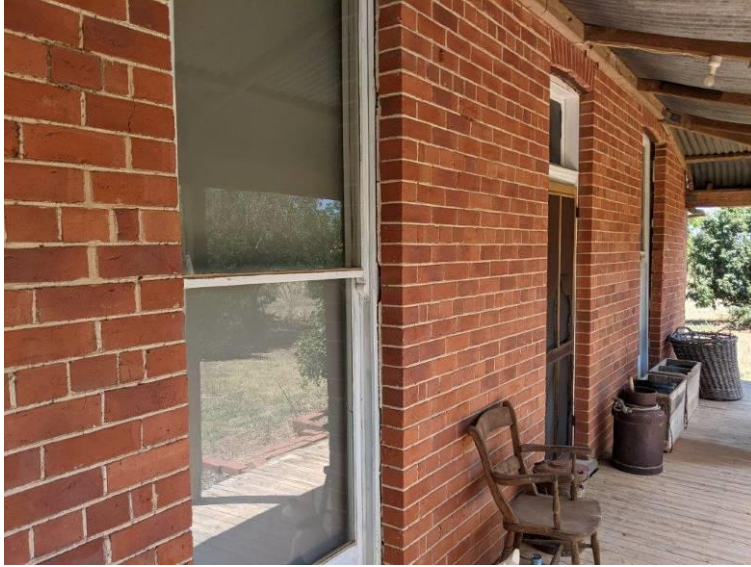
Photograph 12 Postal receiving office (former), Detail view of the North Elevation, noting the rare full height double hung windows and front door with fanlight.
