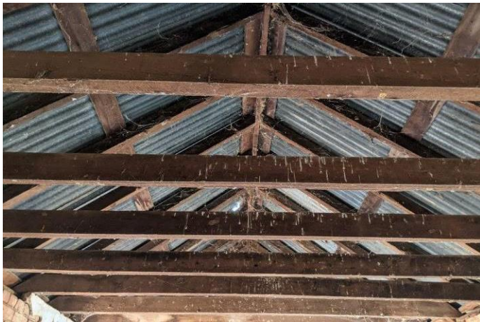
Photo 18 Detail view of the timber roofing and ceiling joists or collar ties. The fully carpentered structure is traditional set of fully dressed rafters and triangulating joists. There is no evidence of a structured ceiling.
