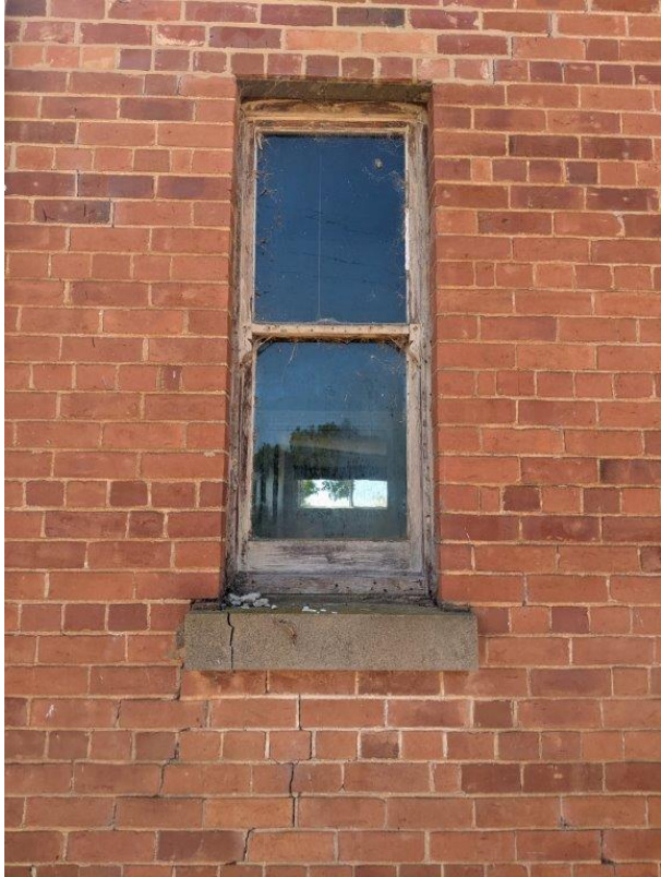
Photograph 7 Post Office (former), Detail view of the narrow timber double hung sliding sash window circa Inter-war period, rendered sill, altered lintel and the South Elevation
