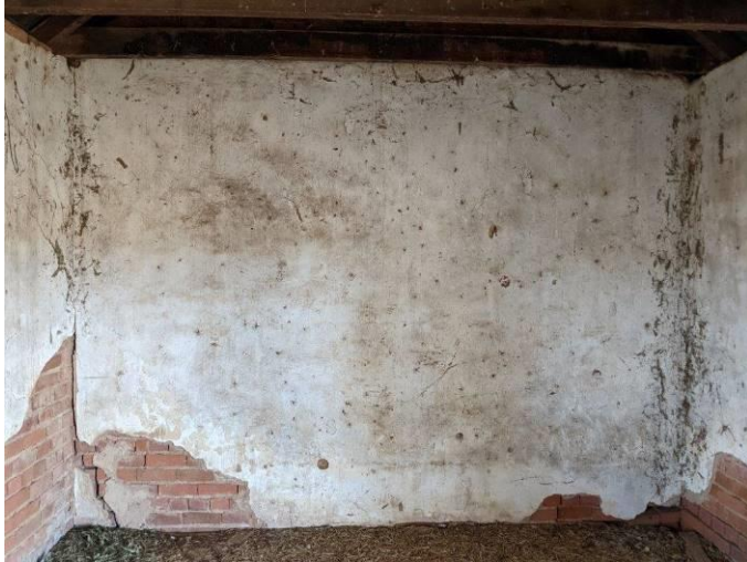
Photo 20 Plaster wall on the South Elevation with damage due to settlement and rising salt damp.
