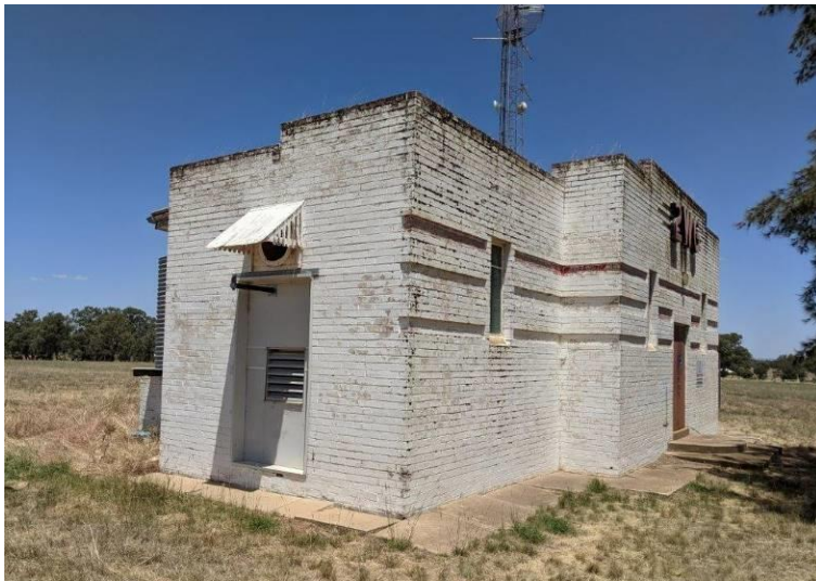
Photograph 8 The North and West Elevations noting the abrupt change to the decorative brickwork and the perimeter concrete paving intended to reduce subsidence.
