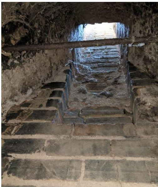
Photo 13 Internal view of the chimney with suspension rod.
