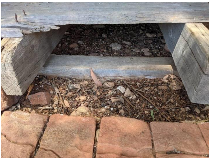
Photo 22 View at the front door where the sub-floor is exposed, noting the in-ground beams supporting the joists. The structure is in sound condition given the damp conditions.
