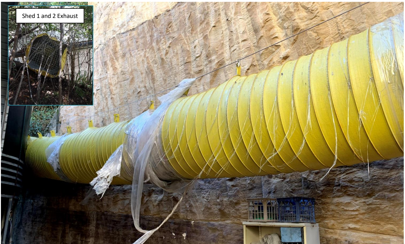
Photo 3 Duct Serving Shed 1 and Shed 4 Wet Scrubbers
