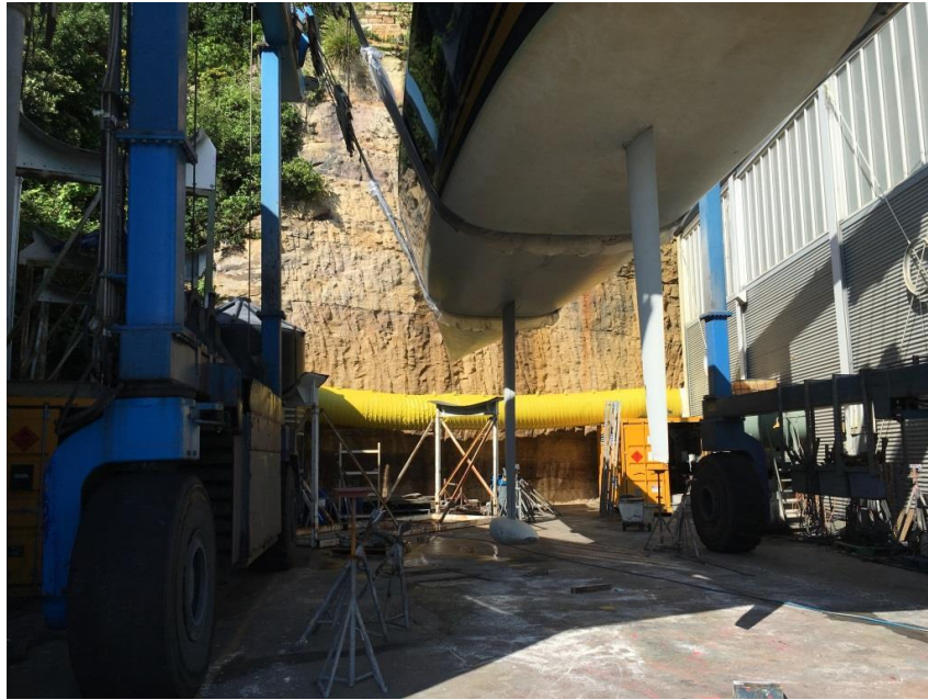
PHOTOGRAPH 0-3 SHOWING DUCT CONVEYING EMISSION FROM SCRUBBER BODY TO SAMPLING POINT TO ENABLE REPRESENTATIVE SAMPLE TO BE COLLECTED
