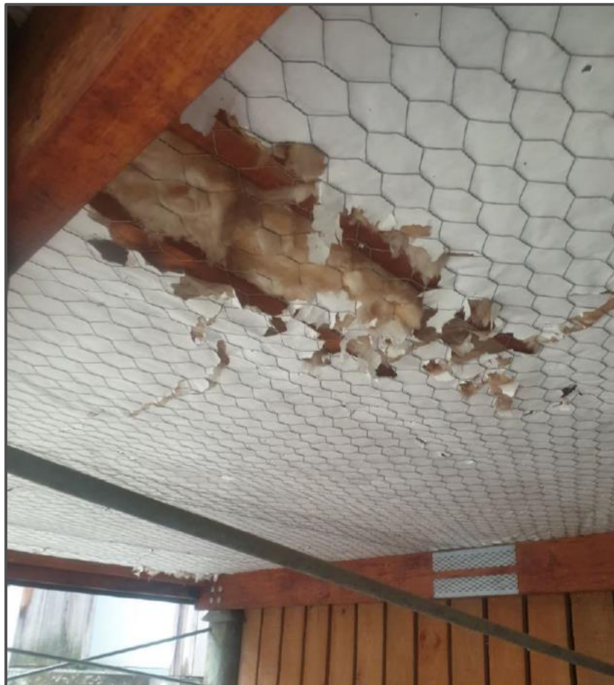
Figure 6 | Example of underfloor to be repaired (item d) (Source: Applicant's documentation)
