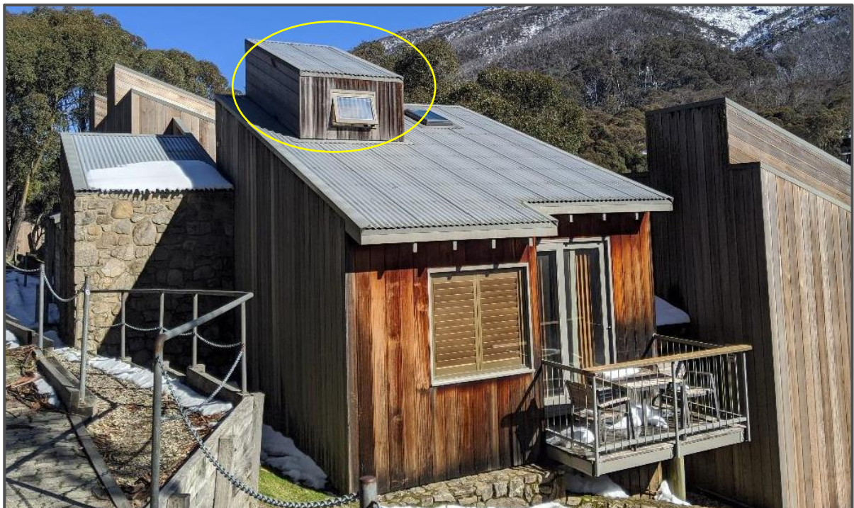
Figure 4 | Example of lantern pop outs to be replaced with metal cladding (item b) (Source: Applicant's documentation)
