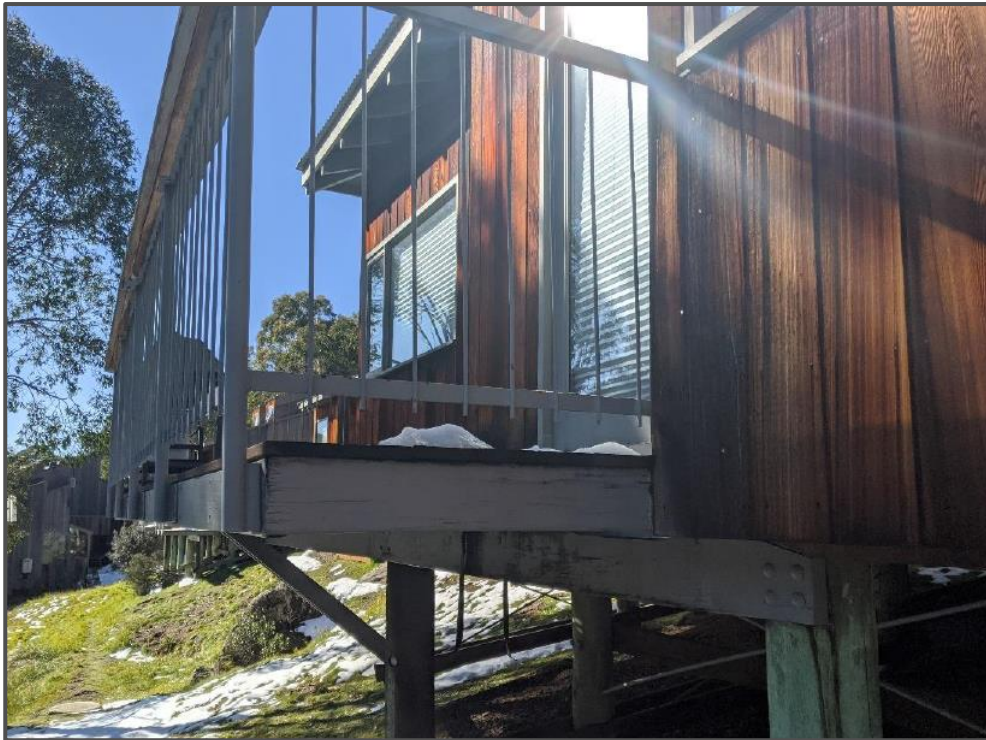
Figure 5 | Example of decking and deck fascia to be replaced (item c) (Source: Applicant's documentation)
