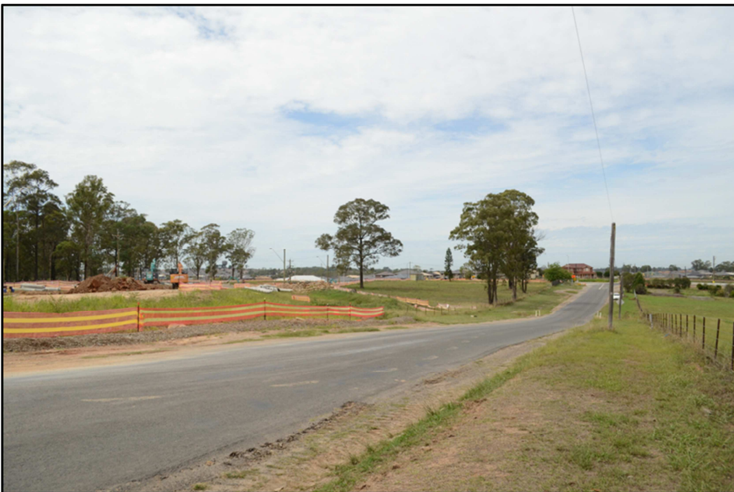
Looking north along Tallawong Rd
