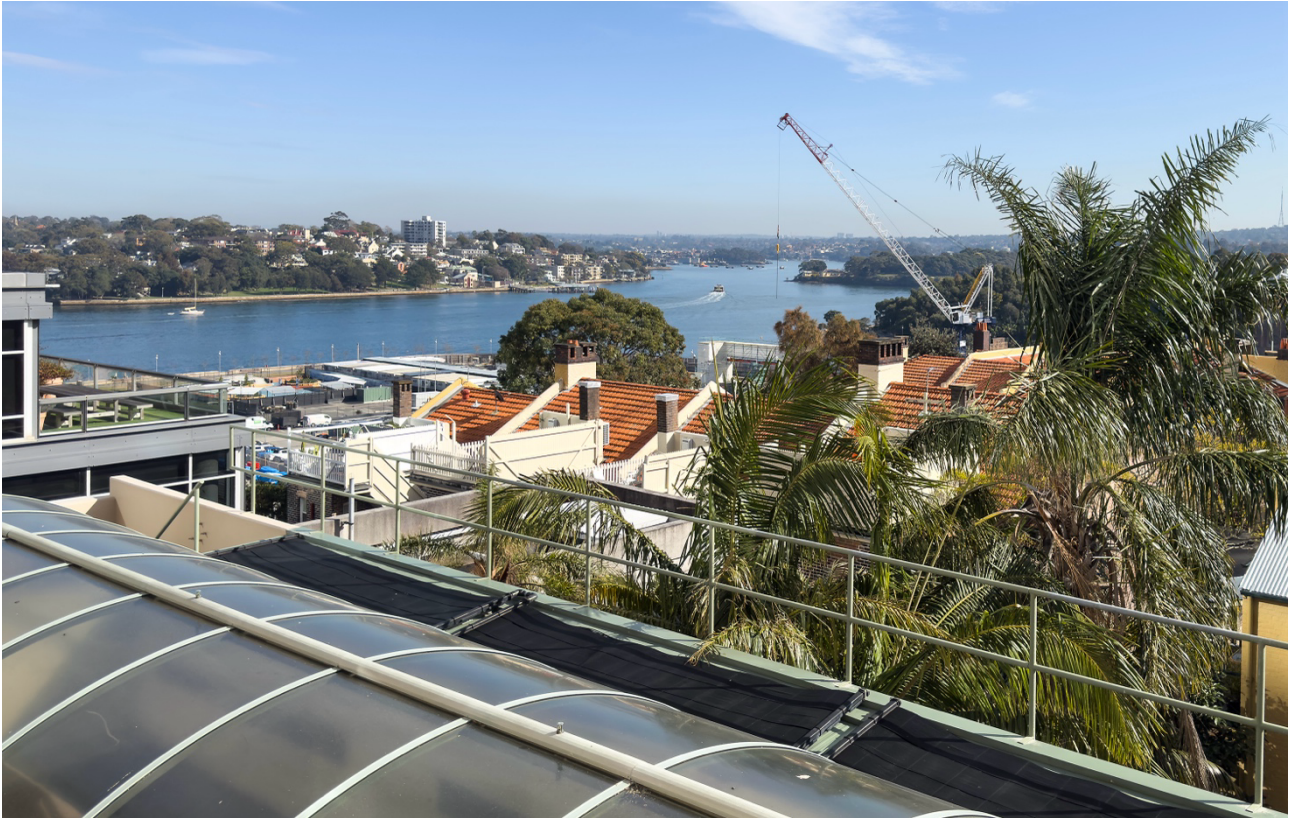
CURRENT VIEW FROM LEVEL 6, HIGHGATE MILLERS POINT
