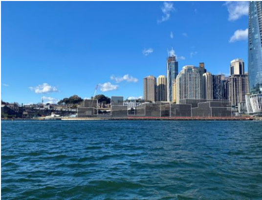
Figure 15: Indicative Approved Building Envelope. Peacock Point, facing east (Source: Digital Line).
