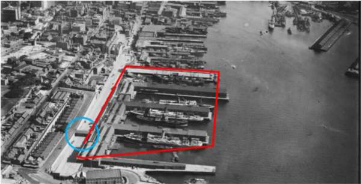
Figure 12 Aerial view showing the approximate study area (red) in c1930 after the demolition of Clyde Street and the creation of High Street and Hickson Road. The former bridge connection over Hickson Road to High Street is shown circled in blue. (Source: GML amended NLA, PIC 1561114257 LOC 21)
