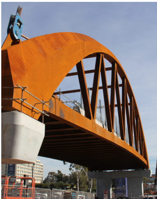
Parramatta Light Rail Bridge
