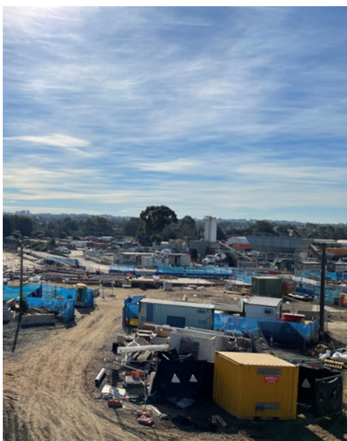
Parramatta Light Rail under construction
